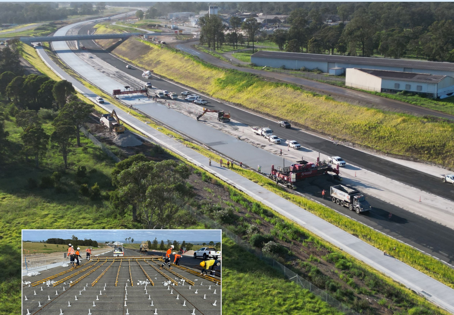
M12 central road pavement being installed, including the shared path
