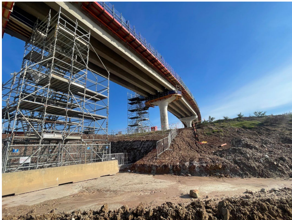
Bridge construction in progress. Note evidence of erosion on batters from recent rainfall.
