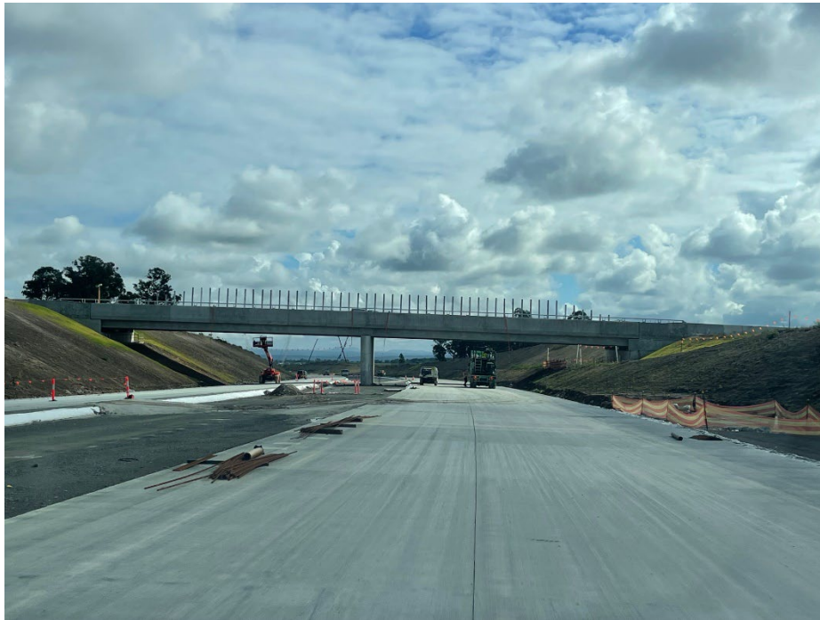
Main alignment looking south showing final pavement.
