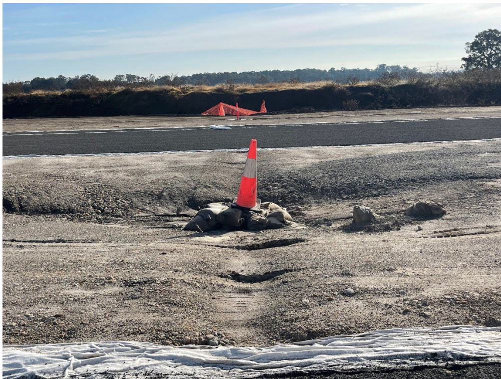
Permanent stormwater pits with ERSER controls in place.
