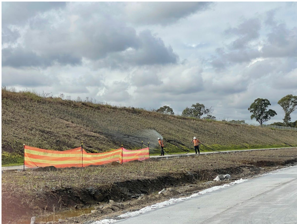
Cutt 22 – hydro mulching works in progress.
