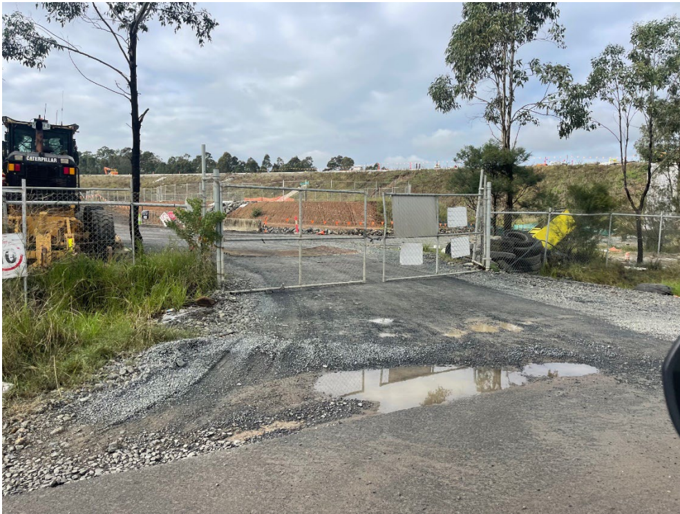
Gate 7 – stabilised access with rumble grid.
