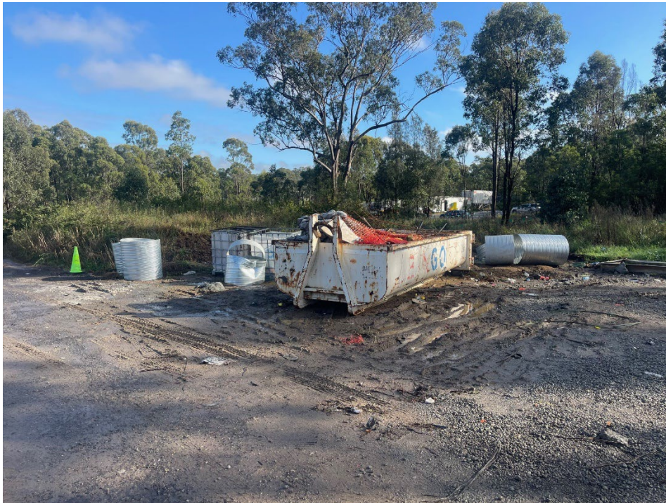
M12C-03- OBS -03 - Gate 5 – waste bins at capacity and IBCs containing residual liquids without secondary containment.
