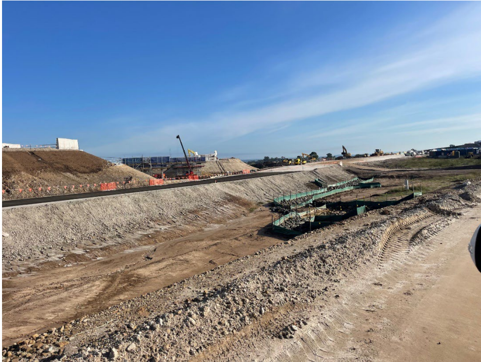
Main alignment, sealing works in progress. Rock lined stormwater drainage channel with a perimeter sediment fence installed.
