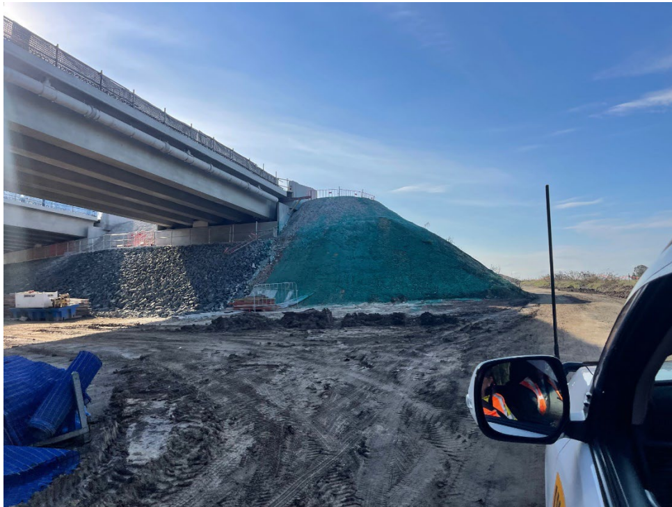
Bridge batter recently sprayed and stabilised with polymer.
