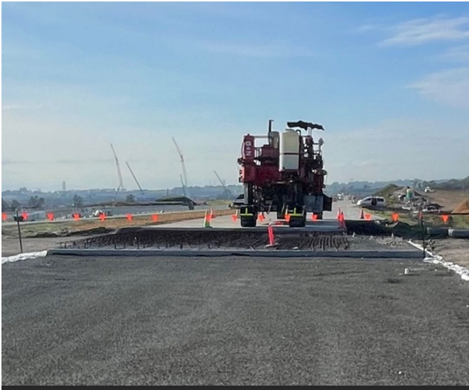
Current extent of mainline concrete pavement with asphal sealant beneath.
