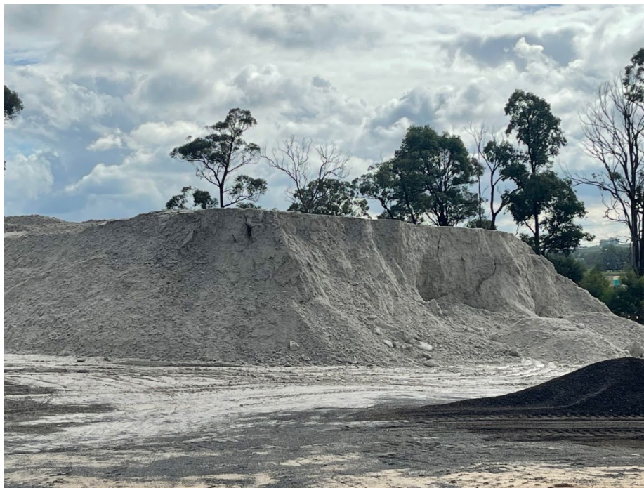
M12C-03- OBS -07 - Stockpile yard – crusher dust stockpile stored greater than 2m high and with vertical sides.
