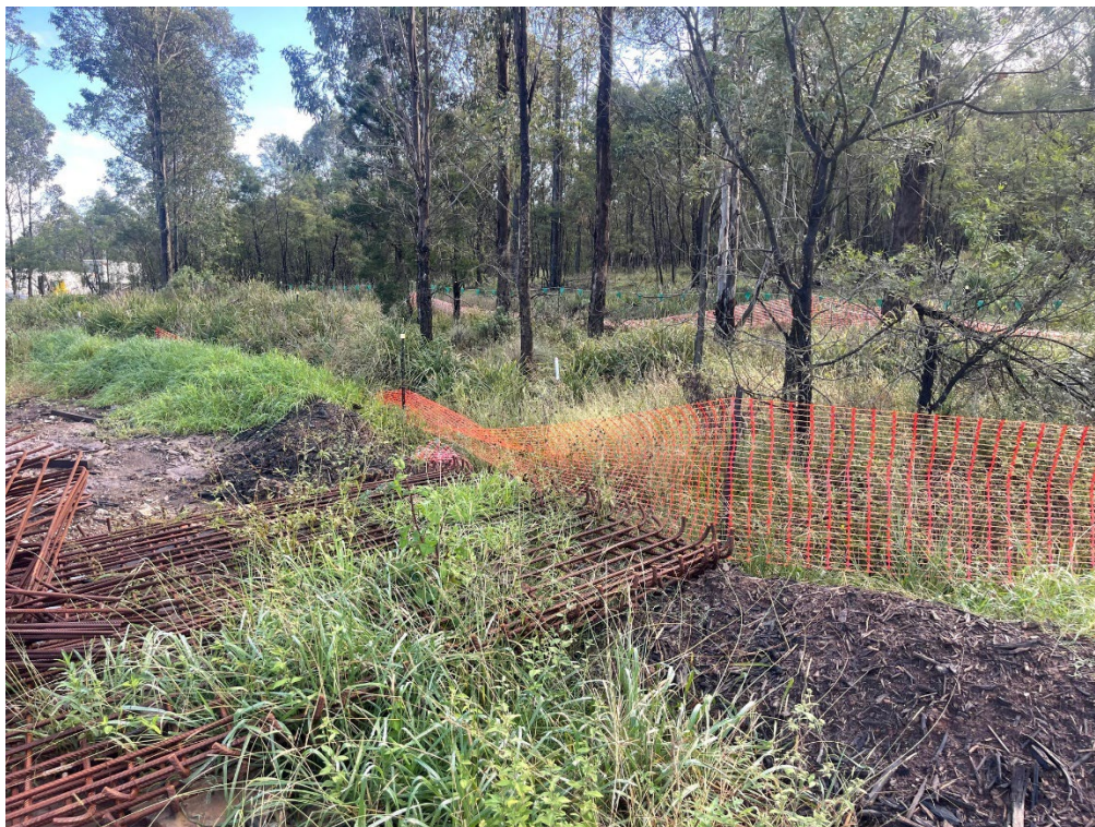
Gate 5 – environmental protection zone with fence demarcation.
