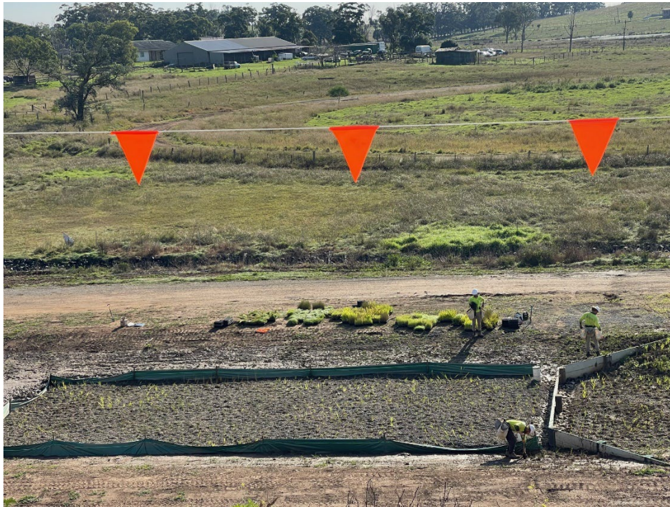
Close up view of bioretention basin – note the aquatic flora being installed for removal of organic pollutants.
