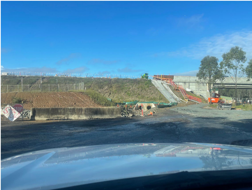
Bridge 10, Gate 5, entrance to site.
