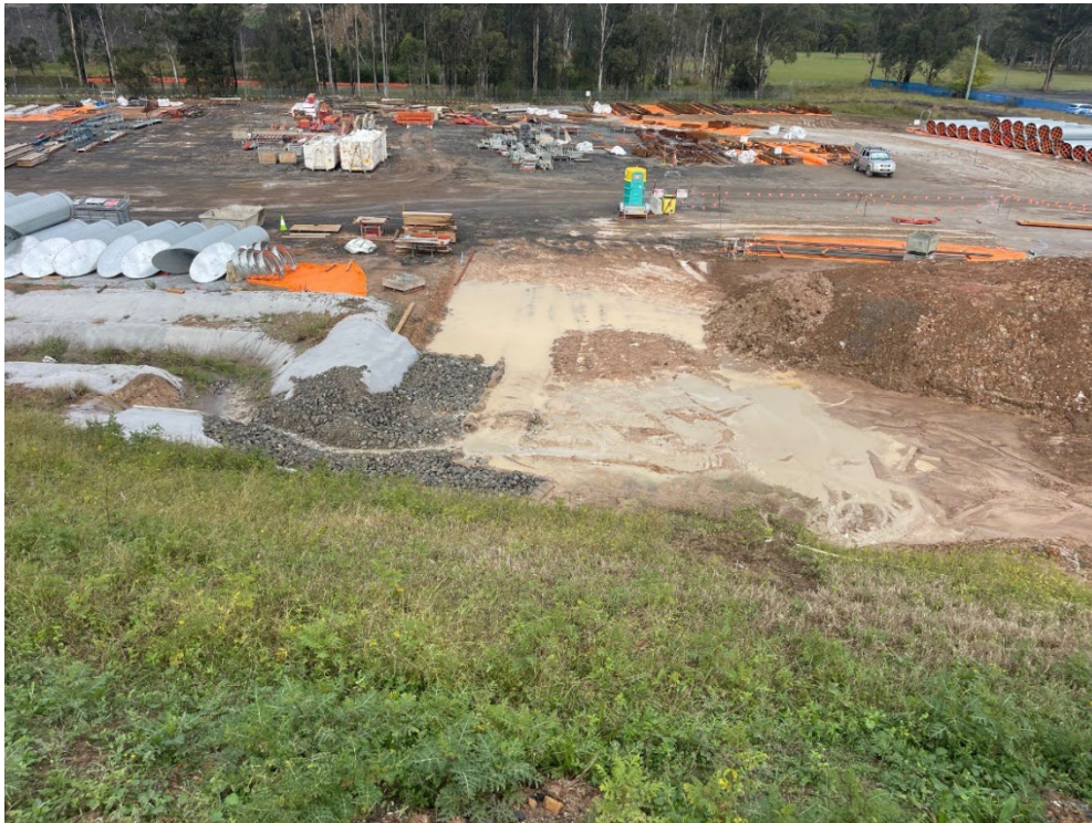
Bridge 9, rip-rap sediment controls at entrance to drainage channel.
