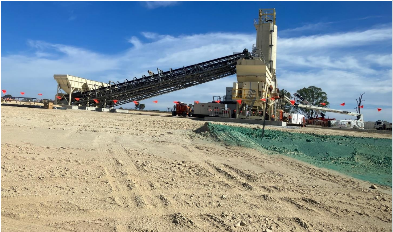
Batch plant soon to be commissioned. Bunds stabilised with polymer.
