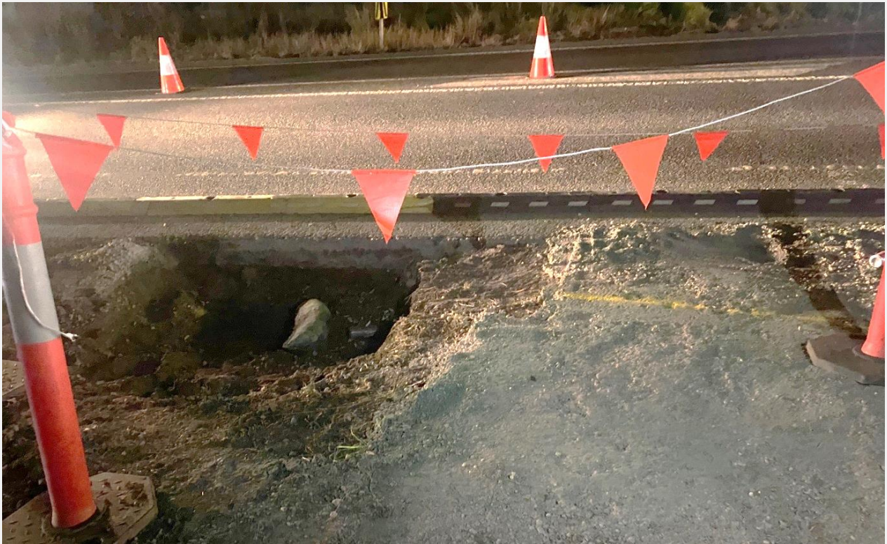
Yellow line is alignment of asbestos pipe.
