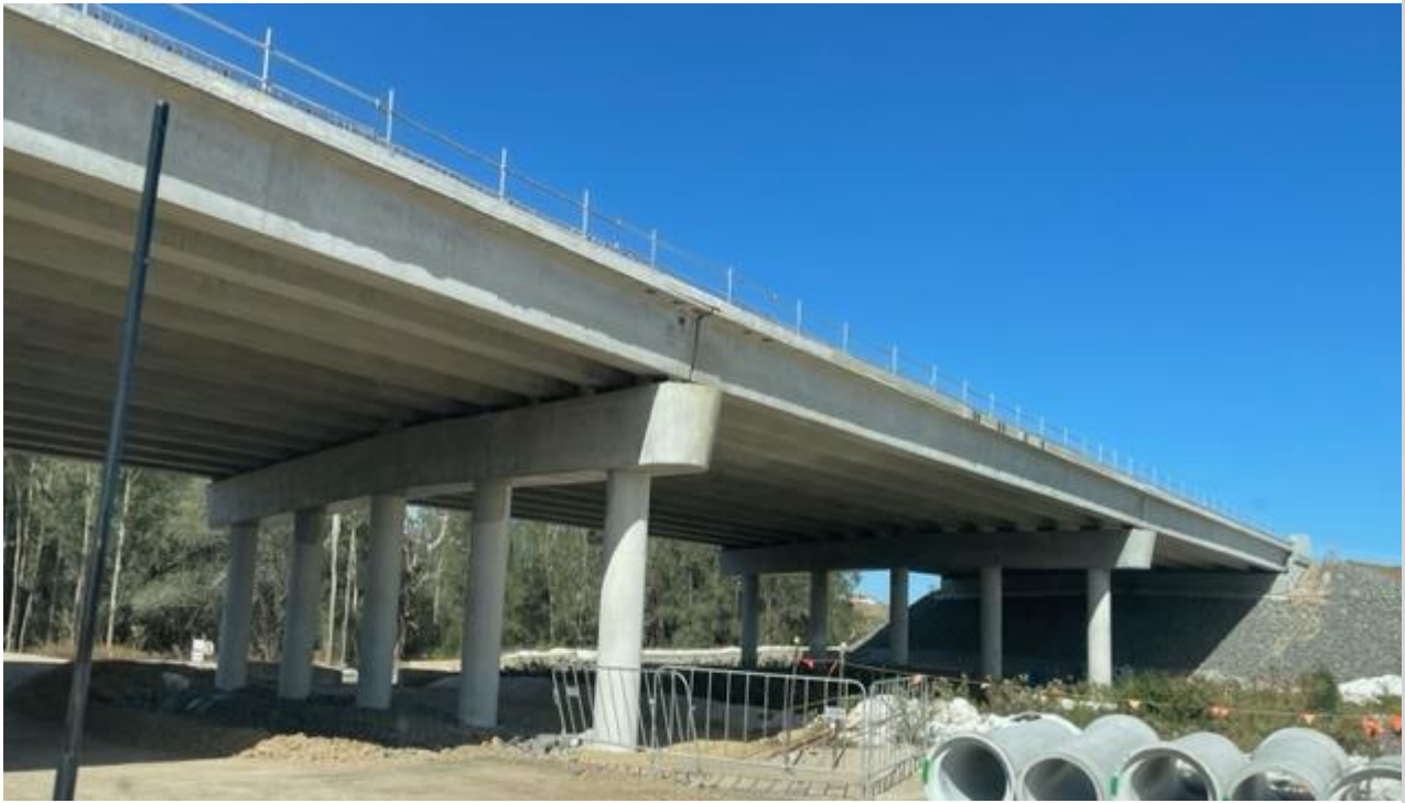
Super T Girders installed
