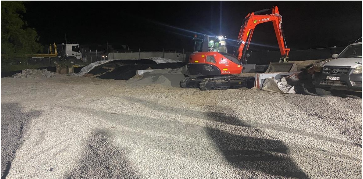
Rock placed to stabilise ground at AF13 site compound.
