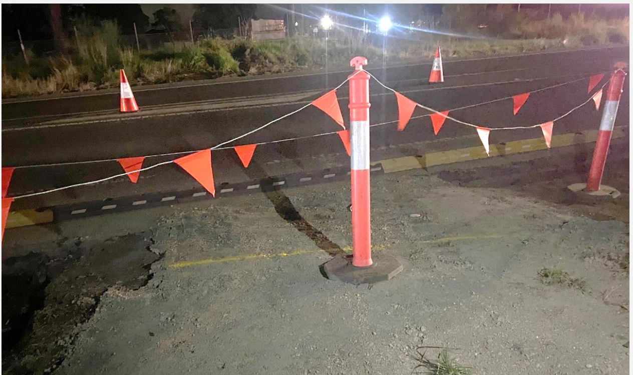
Yellow line is alignment of asbestos pipe.
