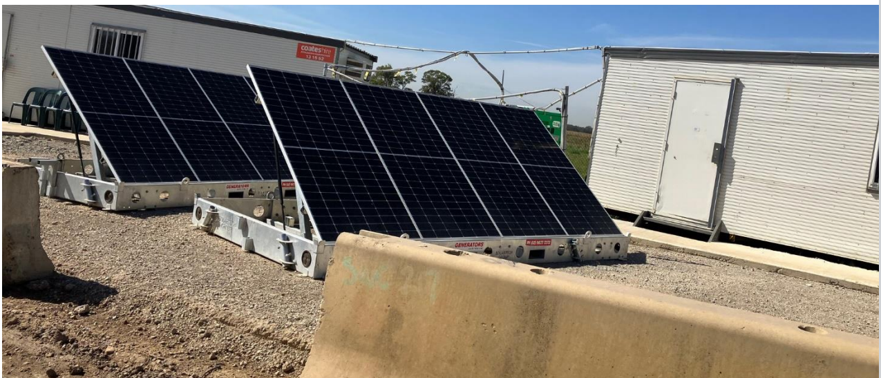
M12 Central solar panels in place for hybrid generator at Range Road facility.
