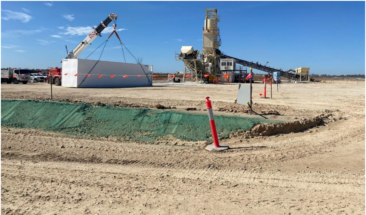
Batch plant soon to be commissioned. Bunds stabilised with polymer.
