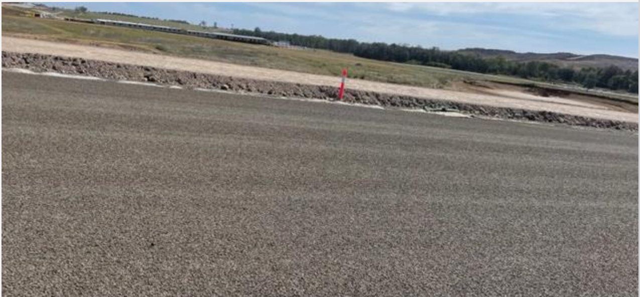
Chip sealing of some areas complete
