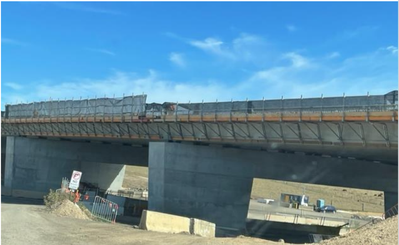
Super T Girders installed
