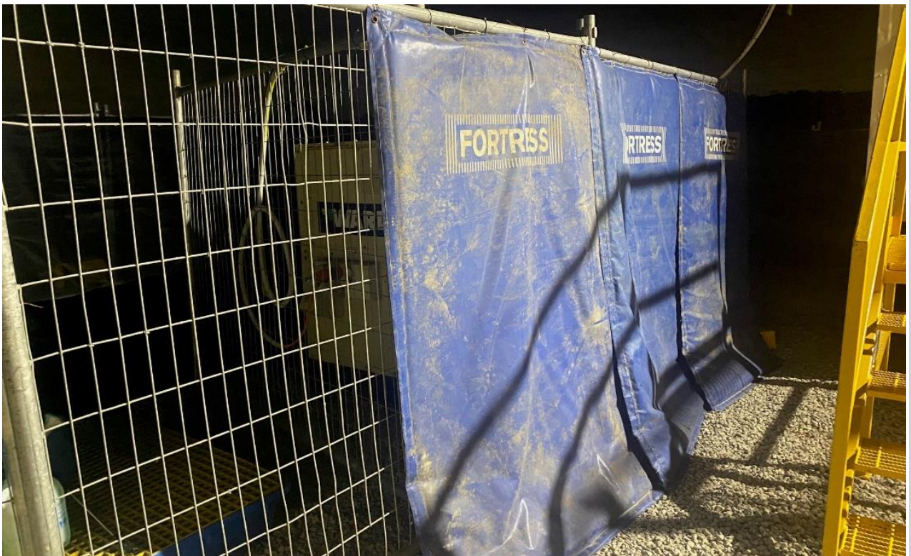
Noise blankets installed around the generator at AF13
