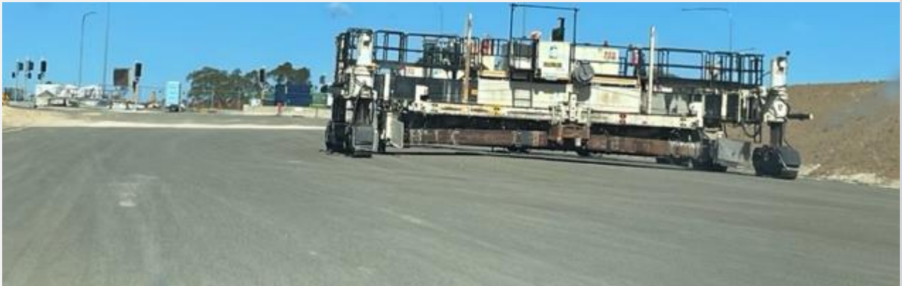
Concrete Slip form Paver at The Northern Road end of works.
