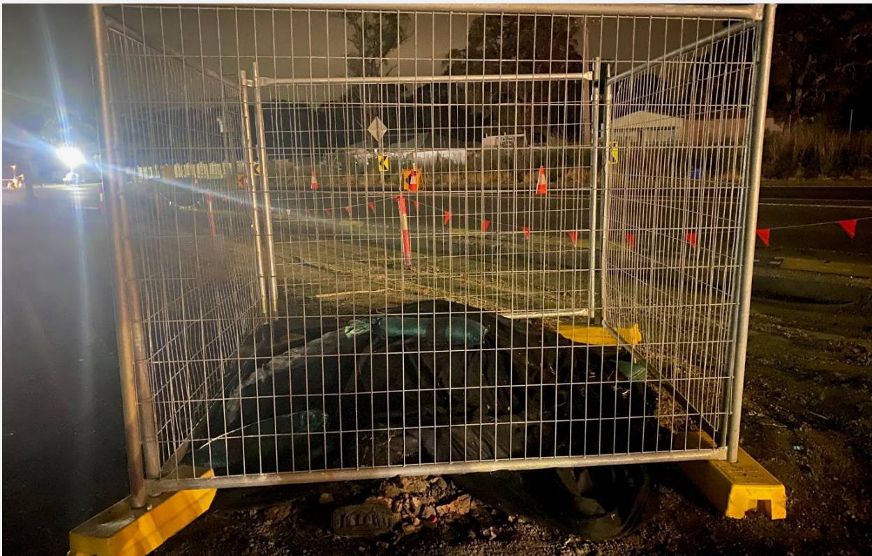
Asbestos find fenced and covered.
