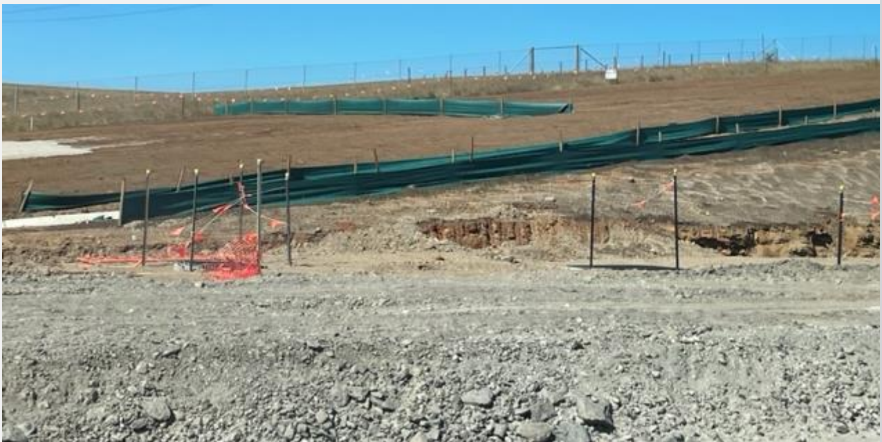
Sediment fencing in place
