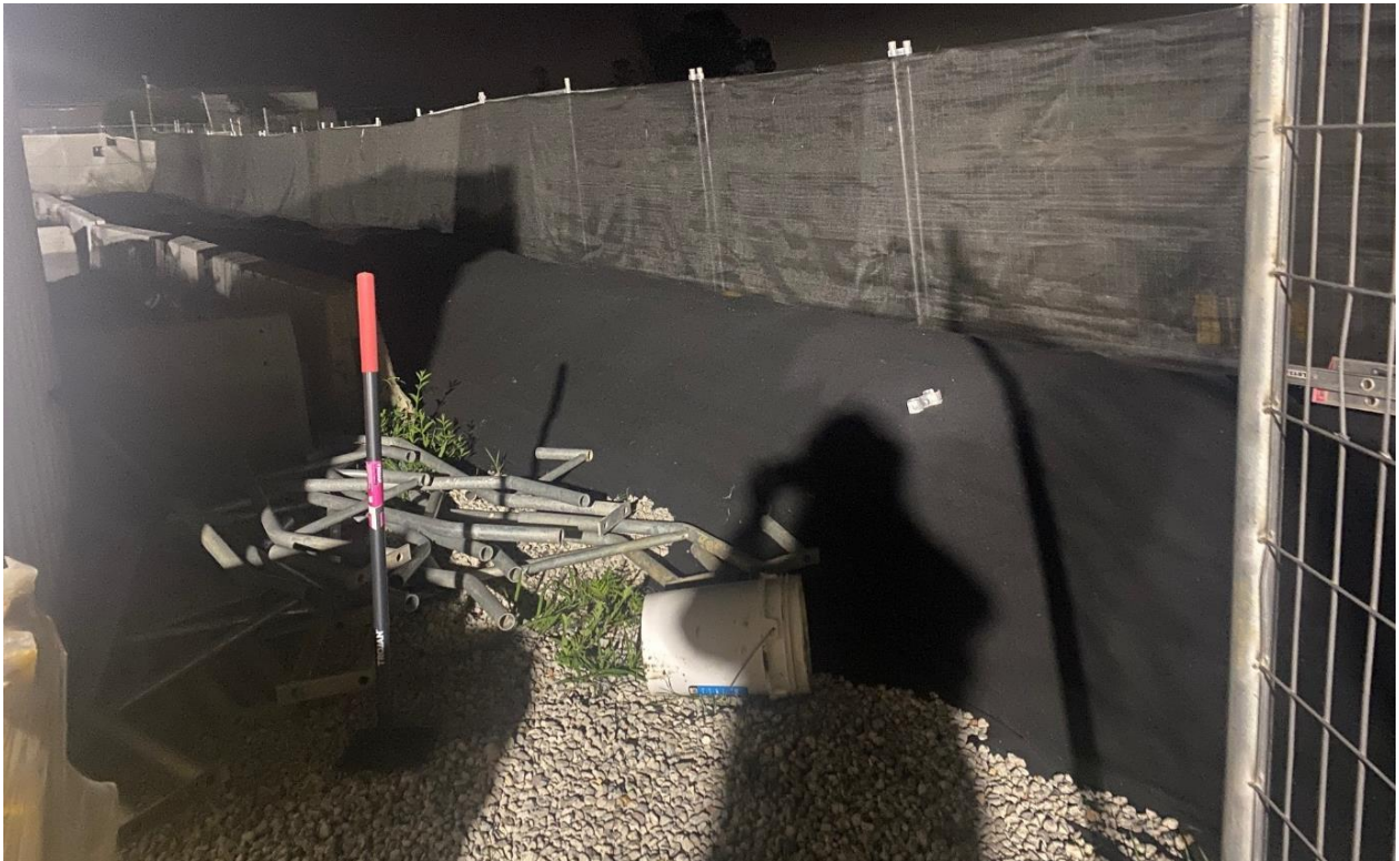
Shade cloth fencing and covered bunds at AF13 site compound.
