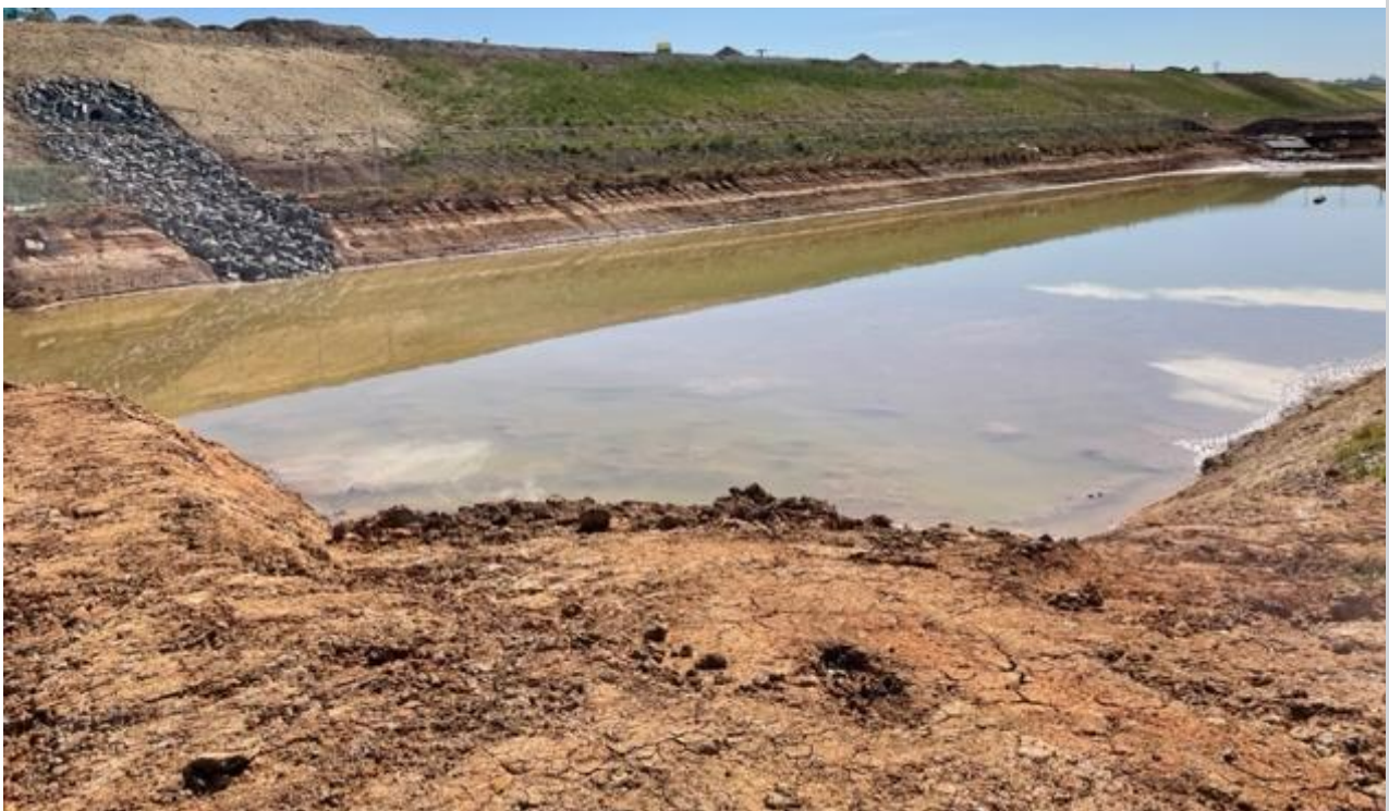
South Creek sediment basin M12 Central
