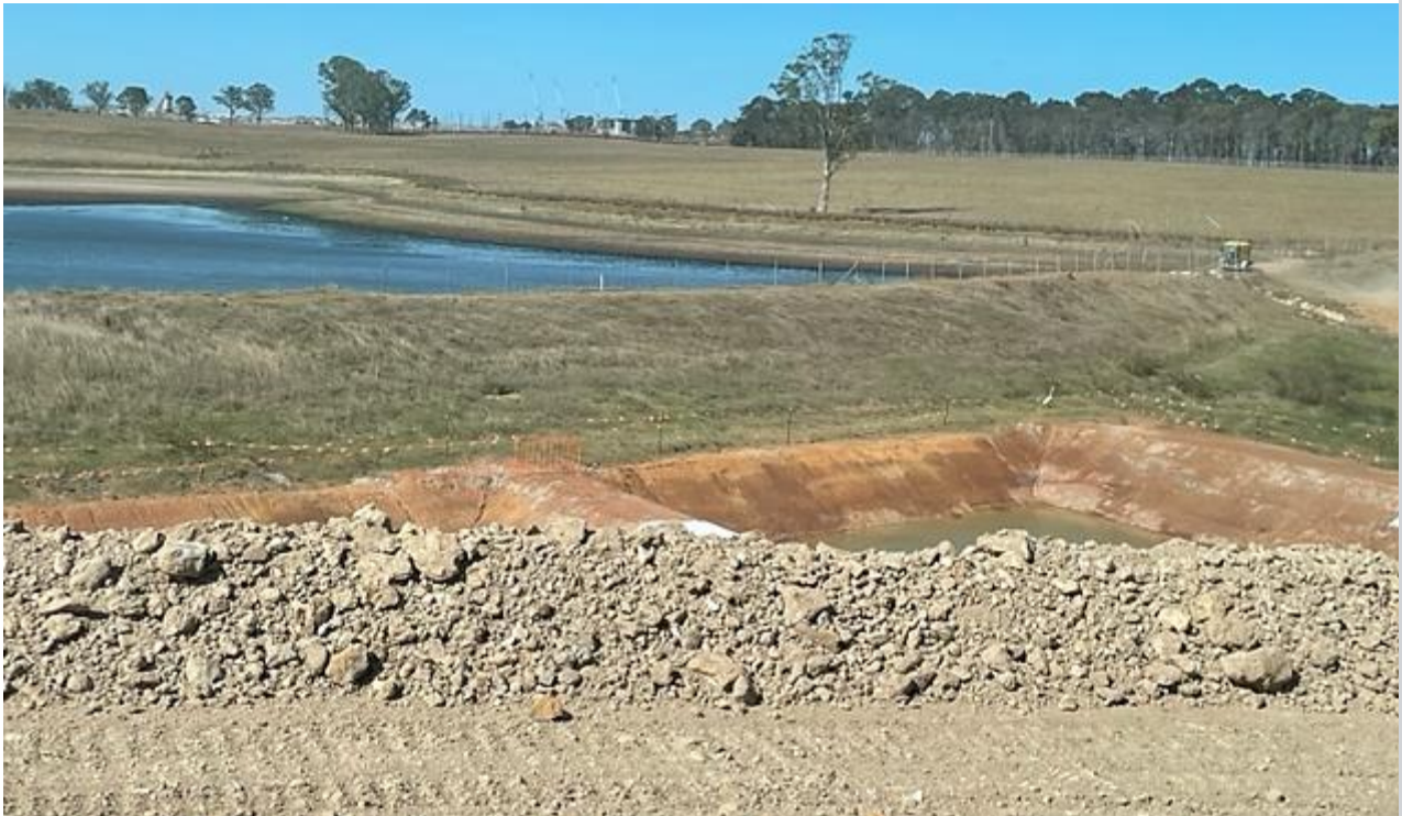
Permanent basin with additional basin for overflow
