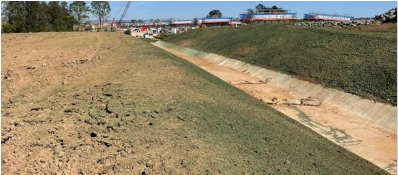
Permanent spillway leading into South Creek, M12 Central
