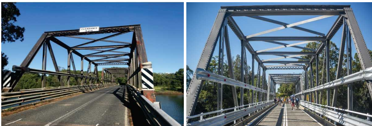
Raleigh Bridge before and after - 2019 showing the repaired and repainted bridge.
