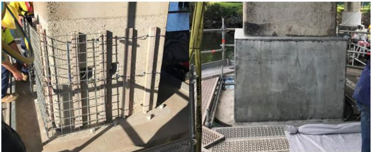
Figure 3-3: Installation of cathodic protection – Wardell Bridge 2019
