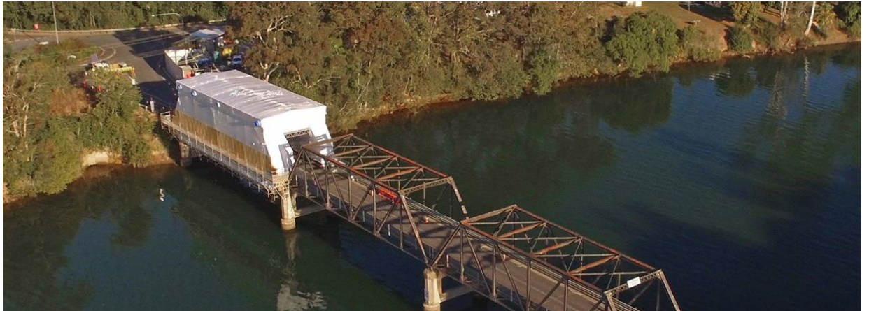
Figure 3-5: Containment system – Raleigh Bridge 2018
