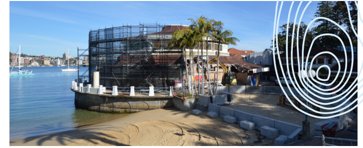
Scaffold set up around the building
