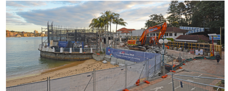
Large excavators carrying out demolition work of the building structure
