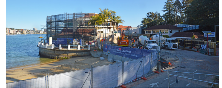
Site ready for the first excavator to begin demolition work
