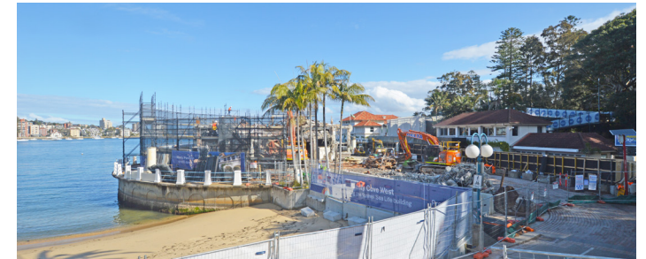
View of the roof being removed
