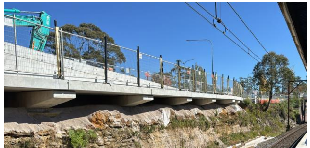
The precast walkway installed in March at Medlow Bath Station.
