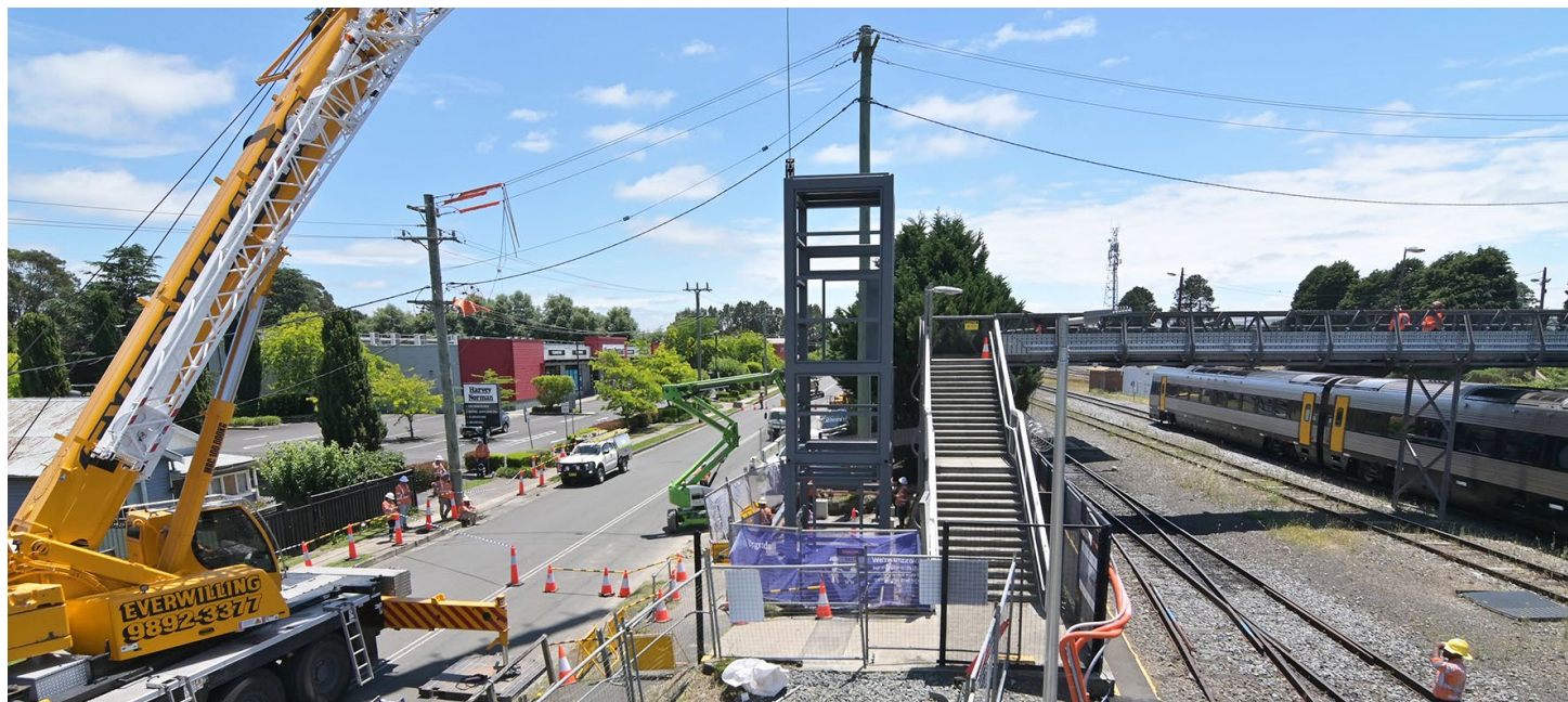
The Lackey Road lift structure has been lifted into place alongside the existing footbridge.
