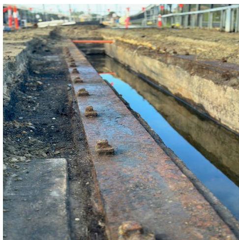
Archaeological finds from the stabling yard upgrade excavation: L-R: Ash Pit (c. 1910) for steam train waste, Inspection Pit (c. 1920) for undercarriage checks, and glass bottles of varying ages.
