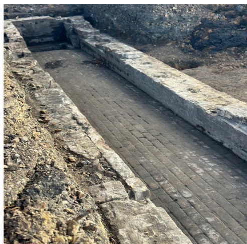
Archaeological finds from the stabling yard upgrade excavation: L-R: Ash Pit (c. 1910) for steam train waste, Inspection Pit (c. 1920) for undercarriage checks, and glass bottles of varying ages.
