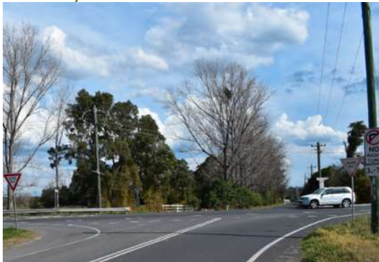
Figure 75: W View of the compound area (behind the tree cover) at the intersection of Kurrajong Road and Bells Line of Road (Lot 1 of DP 742541)
