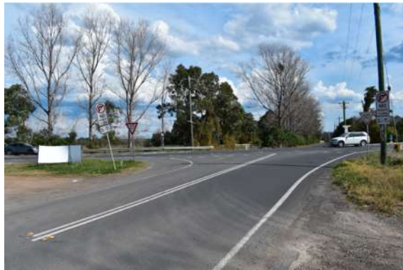
Figure 62: W View of Intersection of Kurrajong Road and Old Kurrajong Road
