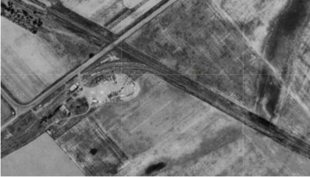
Figure 98: 1947 aerial image demonstrating potential rail siding southwest of the current Kurrajong Road towards Old Kurrajong Road (Source: Historical Imagery Viewer)
