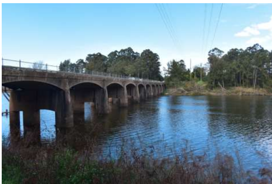
Figure 91: S View of Hawkesbury River Bridge (Source: Artefact, 2023)
