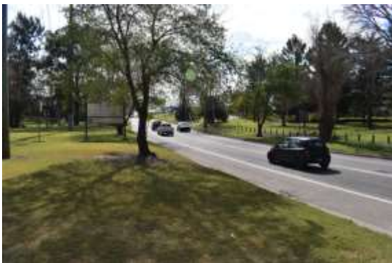
Figure 58: NW View of the park proposed compound area, with Bells Line of Road to the right
