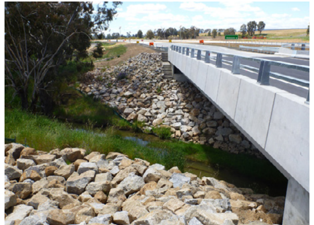
Plate 4-55: Example rock pitching (Hume highway)
