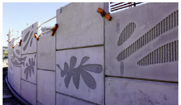
Plate 4-59: Imprinted pre-cast panels with First Nations artwork (Sydney Gateway)
