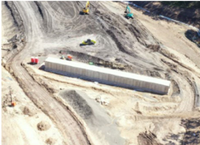
Fauna culvert installation
