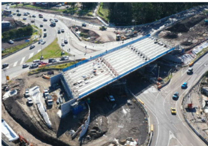
Bridge 6 girder installation
