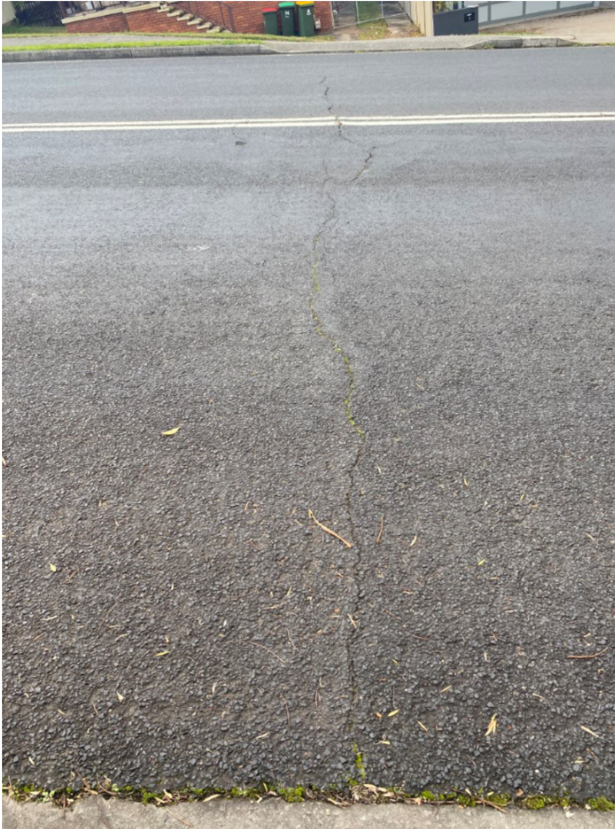
Photo 6: Pavement cracking of Dent St, between Hill and Chinchon Streets.
