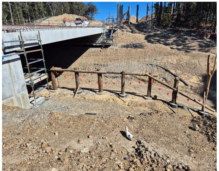
Image 4: Northern Interchange, Bridge 4 shared underpass with fauna connectivity furniture.
