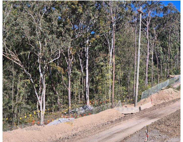
Image 6: Mainline, installation of pole to host fauna overpass connection.
