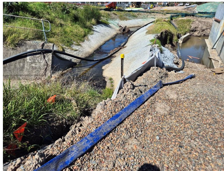
Image 3: Northern Interchange, Dark Creek culvert diversion.
