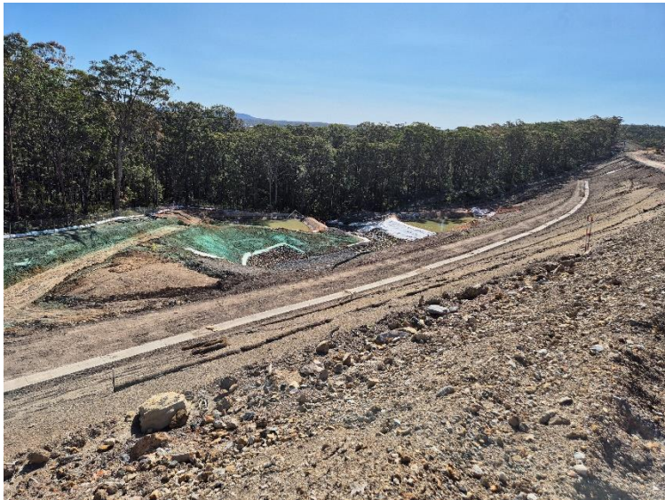
Image 7: Mainline, ErSed controls in place with soil binder being used to stabilise soils during construction.
