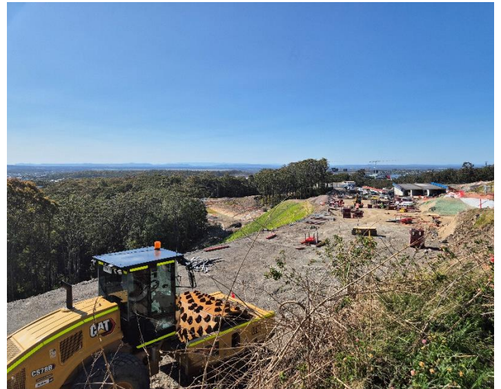
Image 8: Southern end of the project. The Green shading is landscaped batter with strong stabilising growth.
