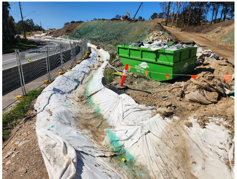
Image 4: View to the east on McCaffery Drive.
