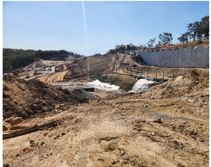
Image 8: Midway through main line, adjacent to JHH, view looking north.
