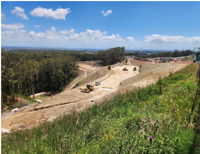
Image 7: Southern Interchange works.
