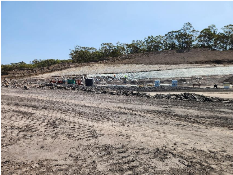
Image 5: Midway through main line, view looking west showing the shotcrete formwork.
