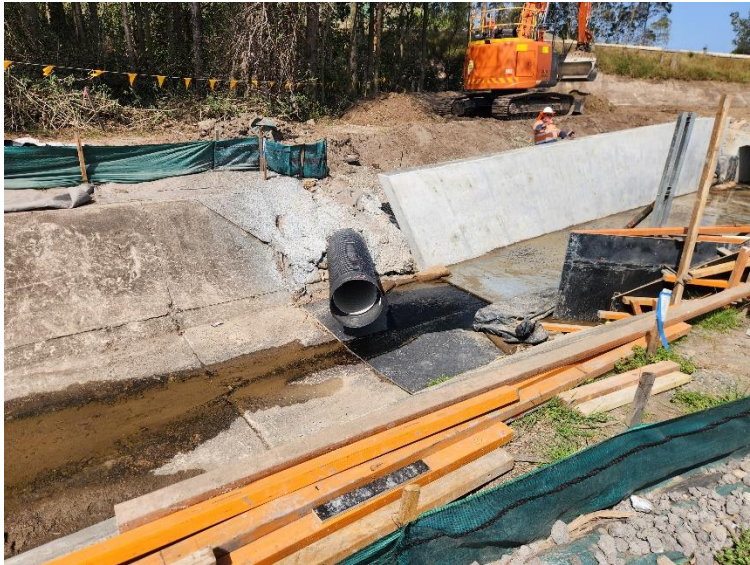
Image 7: Northern interchange, Dark Creek extension culvert works north of Newcastle Road.
