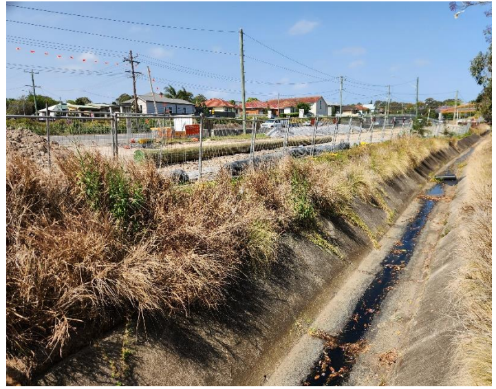
Image 6: Northern interchange, Dark Creek south of Newcastle Road.
