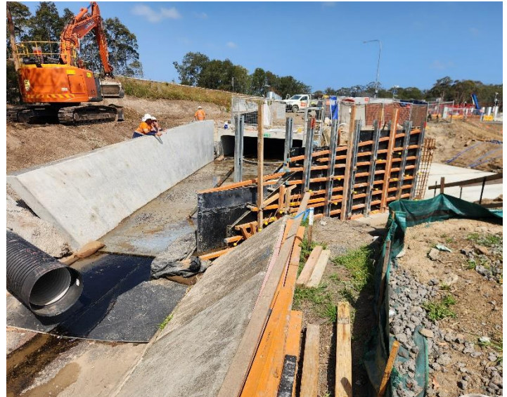
Image 8: Northern interchange, Dark Creek culvert extension works north of Newcastle Road.
