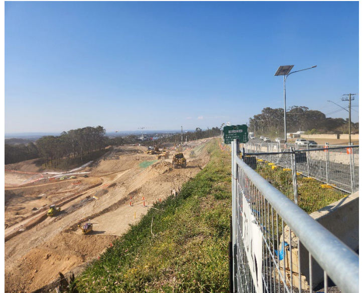
Image 8: View from Lookout Road, looking north.
