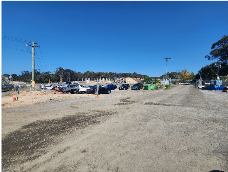
Image 1: Northern Compound (Newcastle Road) view looking east from site offices.
