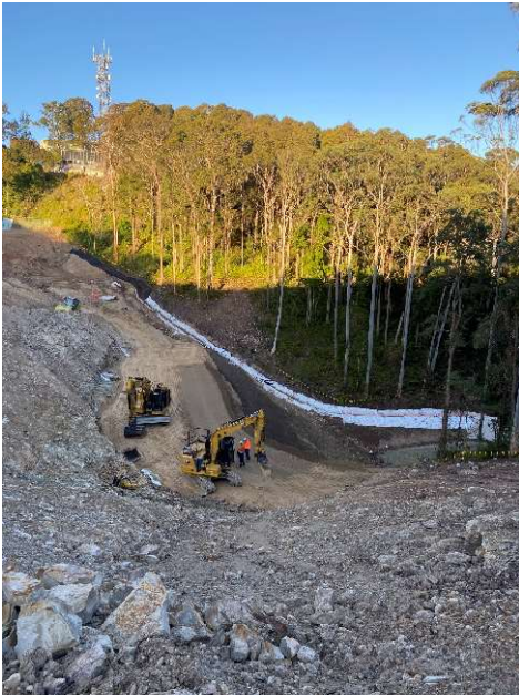
Southern Interchange – Fill 1
