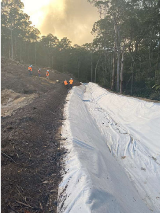
Diversion drainage during clearing
