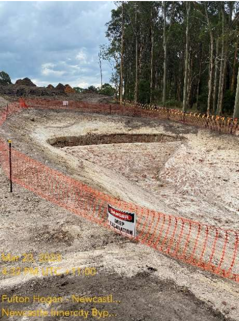
Temporary sediment basin construction
