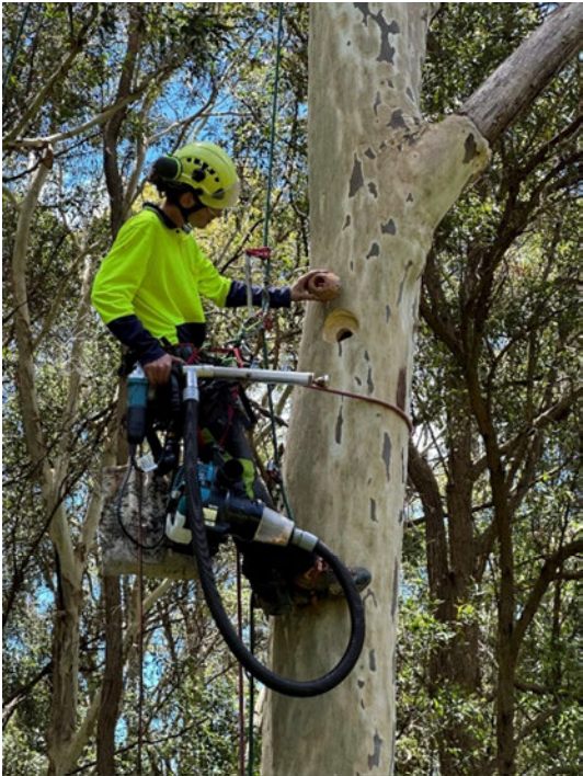
Installation of Hollow-hog
