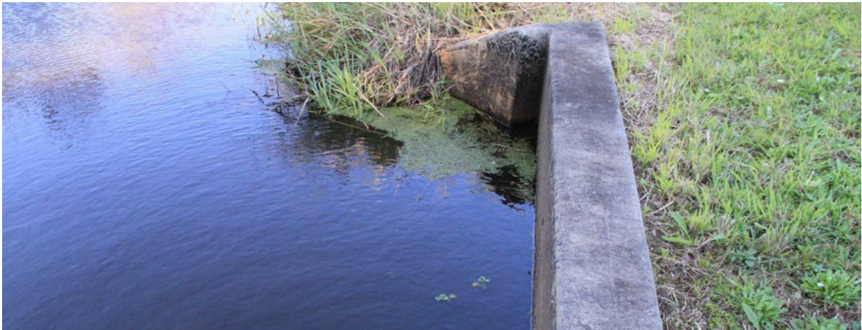
Figure 3-10: Culvert under Coopernook Road – between Pacific Highway and proposed roundabout
