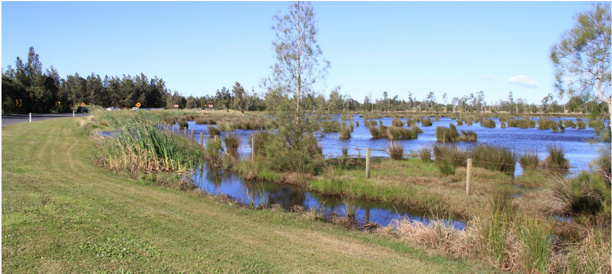
Figure 3-9: Ponding water – view south-east along southern side of Coopernook Road from eastern project extent
