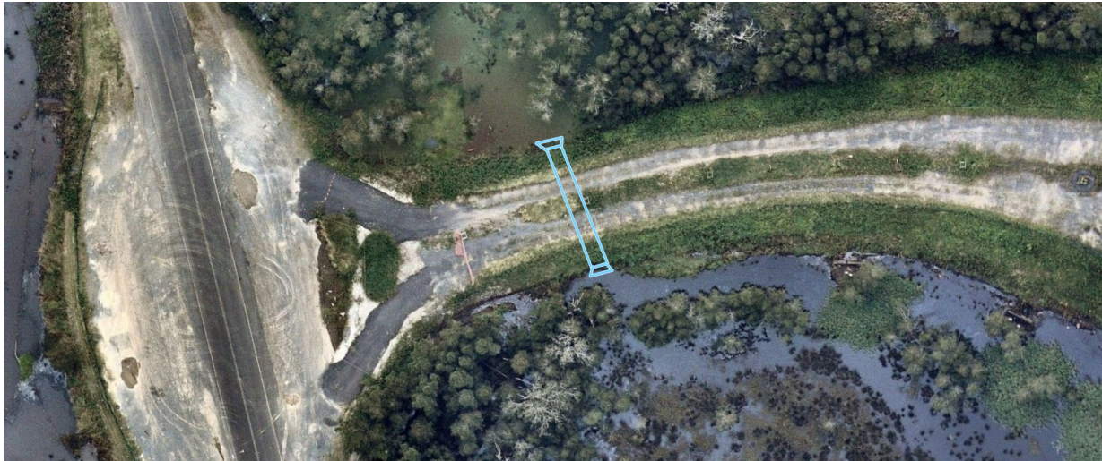
Figure 3-11: Culvert under pre-loaded area adjacent to Coopernock Road (Nearmap, 23 March 2022)
