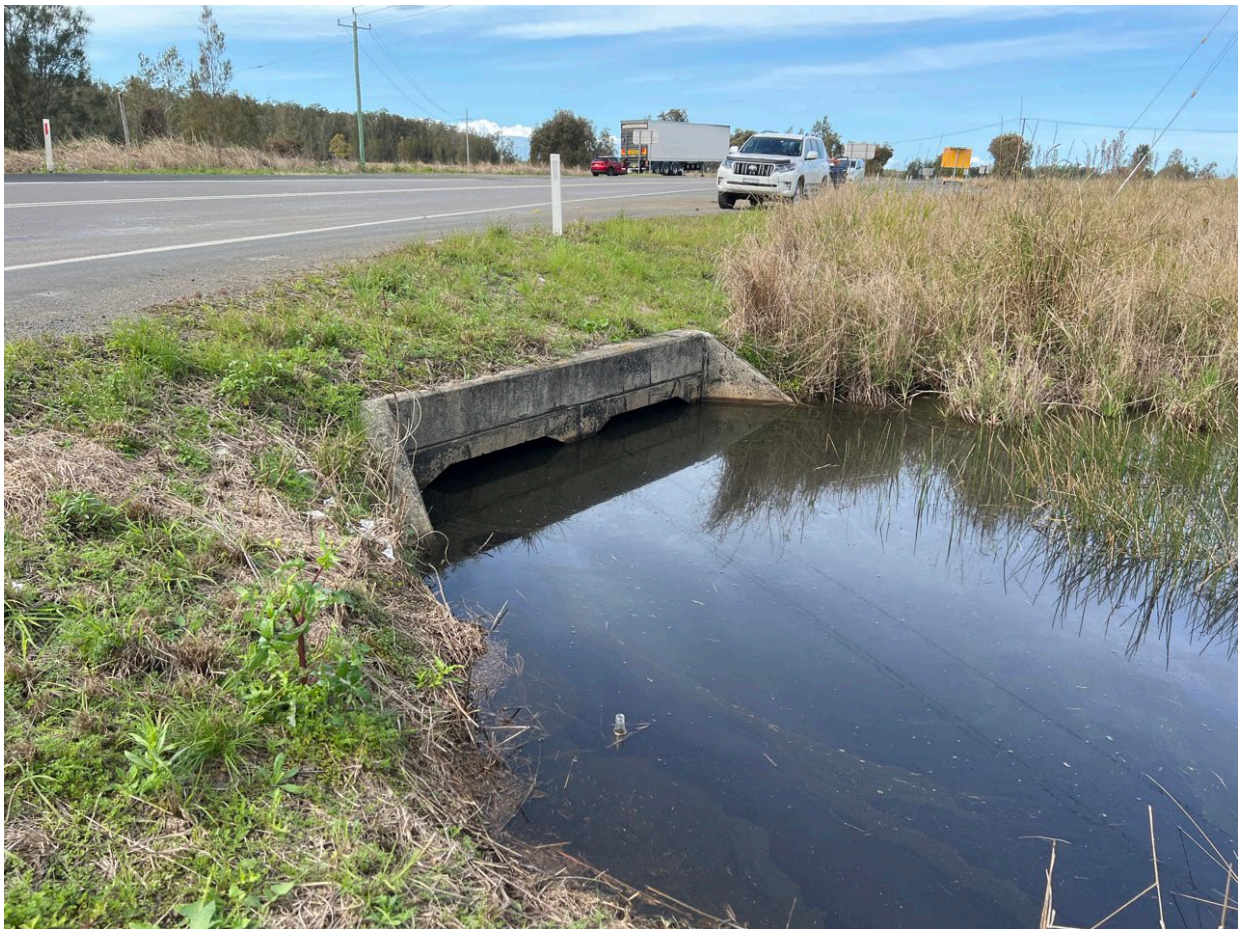
Photo 3-5: Existing road culvert within the study area
