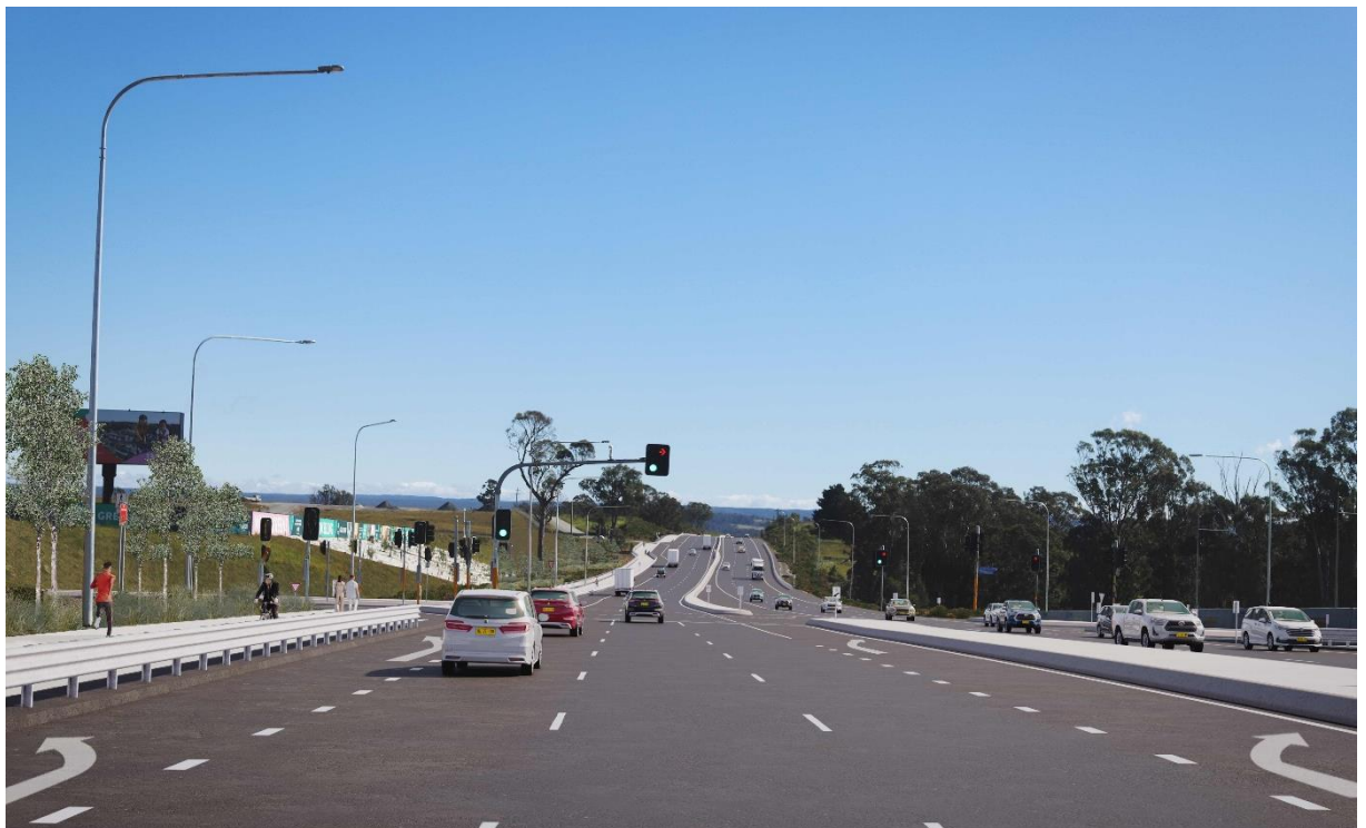
Figure 6-32: Visual representation of the proposal at viewpoint 03 – Pembroke Parade at Bingara Gorge entry (eastern approach)
