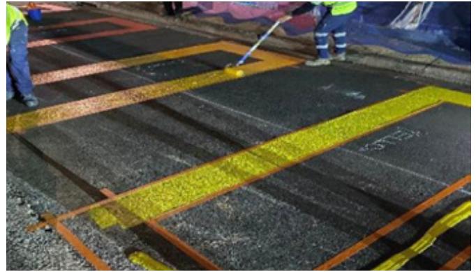
Railway Serviceway being painted. Image courtesy: Liverpool City Council.
