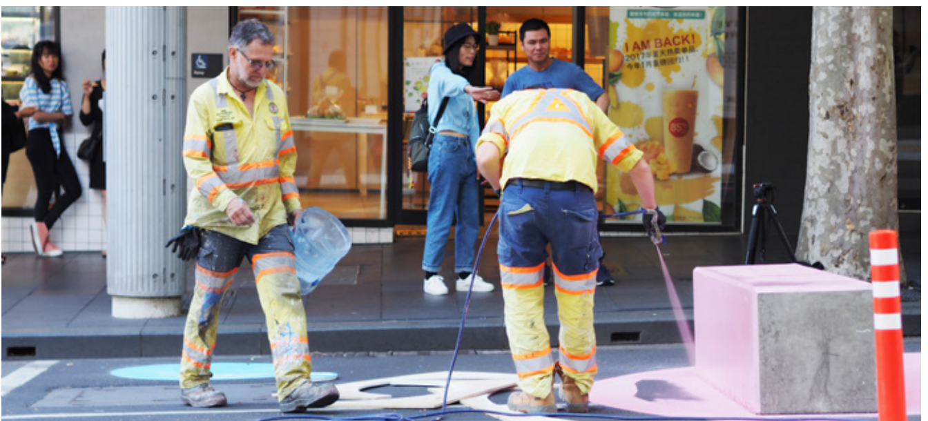
Installation of the painted design on the asphalt. Image courtesy: NSW Government.
