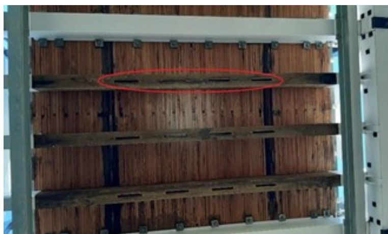
Figure 3: Deep recesses were drilled in the girders under the bridge
