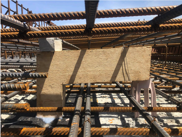
Figure 6: Microbat habitat was built within the structure of the bridge
