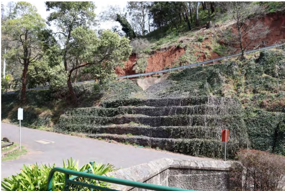
Figure 5:4 View of the failed slope from Caves House entrance: Note: modern gabions on the slope below (Source: MTS Heritage, 2021).
