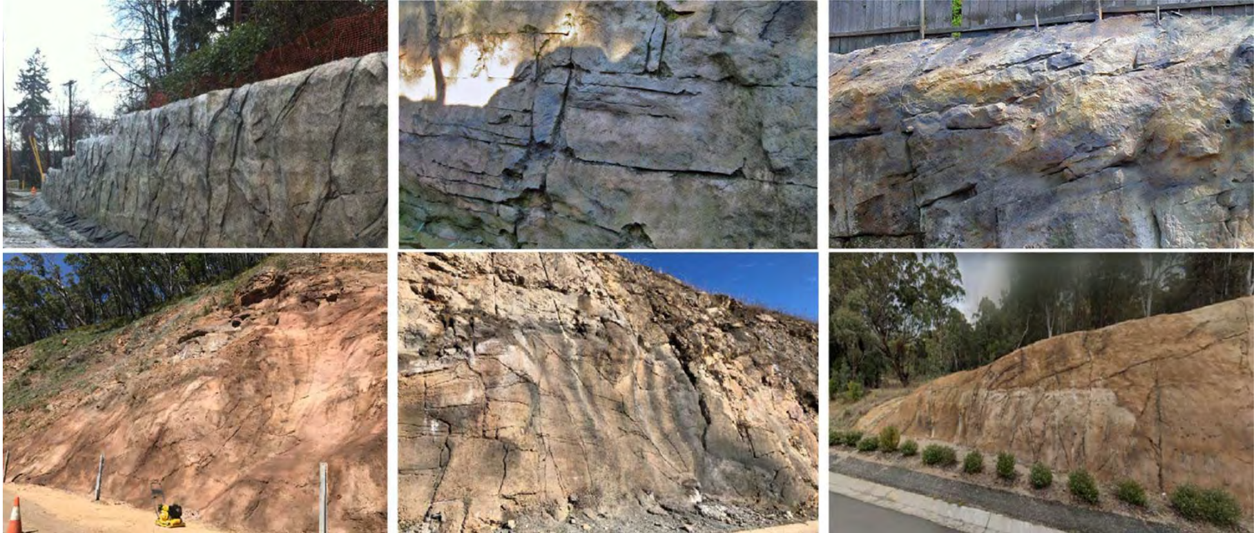
Figure 7.2: Examples of mock-rock textured finish on recent shotcrete applied to slope failures in the Sydney region (Source: J. Zyhalak, personal communication, 21 October 2021)
