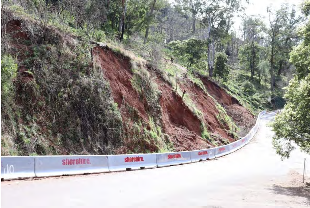
Figure 5:2 View of the failed section of Jenolan Caves Road, facing north east (Source: MTS Heritage, 2021)
