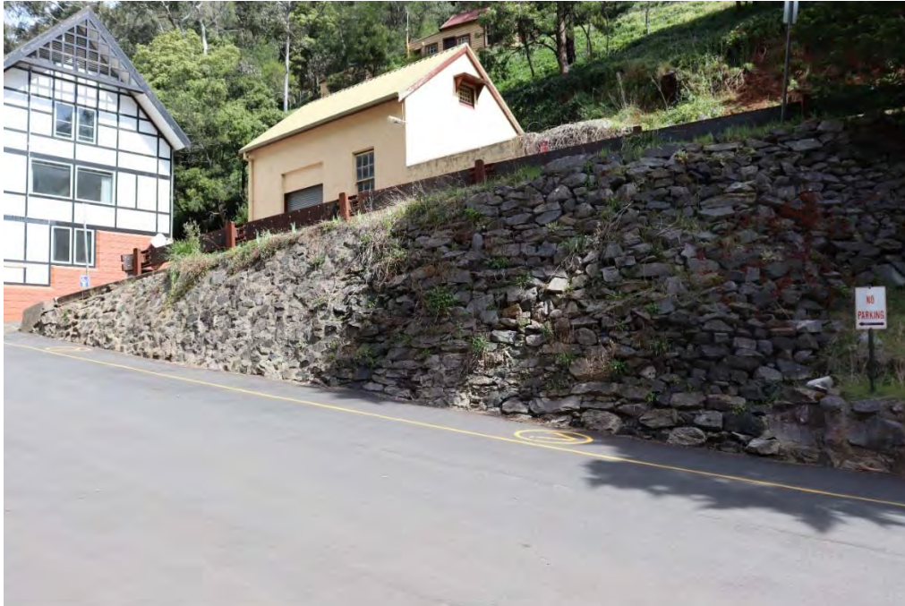
Figure 5:10 Dry stone retaining wall below Jenolan Caves Road, facing west (Source: MTS Heritage, 2021)
