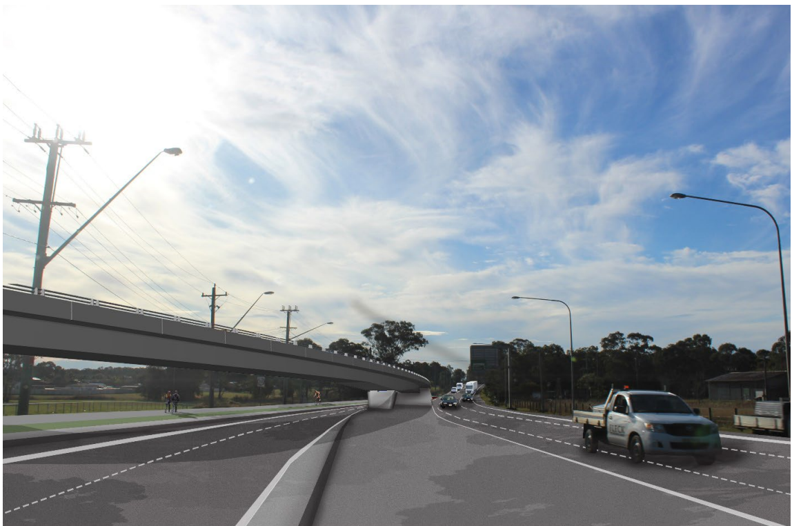
Figure 6-33 Proposed viewpoint 4 - Richmond Road, looking north towards Bells Creek bridge crossing
