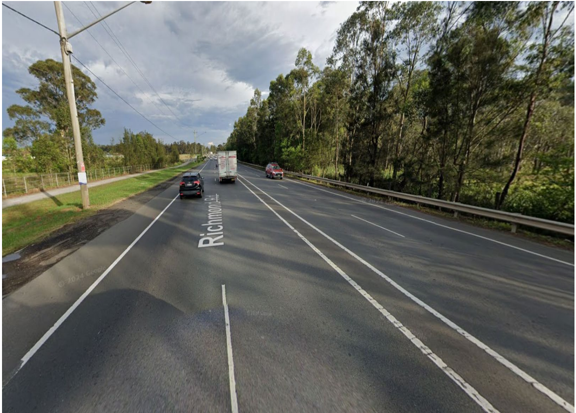
Figure 6-36 Existing viewpoint 6 - Richmond Road Bells Creek bridge crossing, looking north
