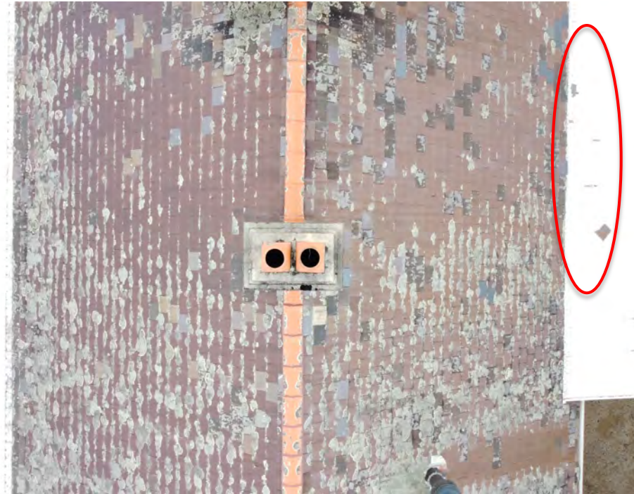
2021 Debris on adjacent roof shed from roof (Platform 1 roof)
