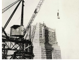
Lifted Masonry for Pylon Tower
