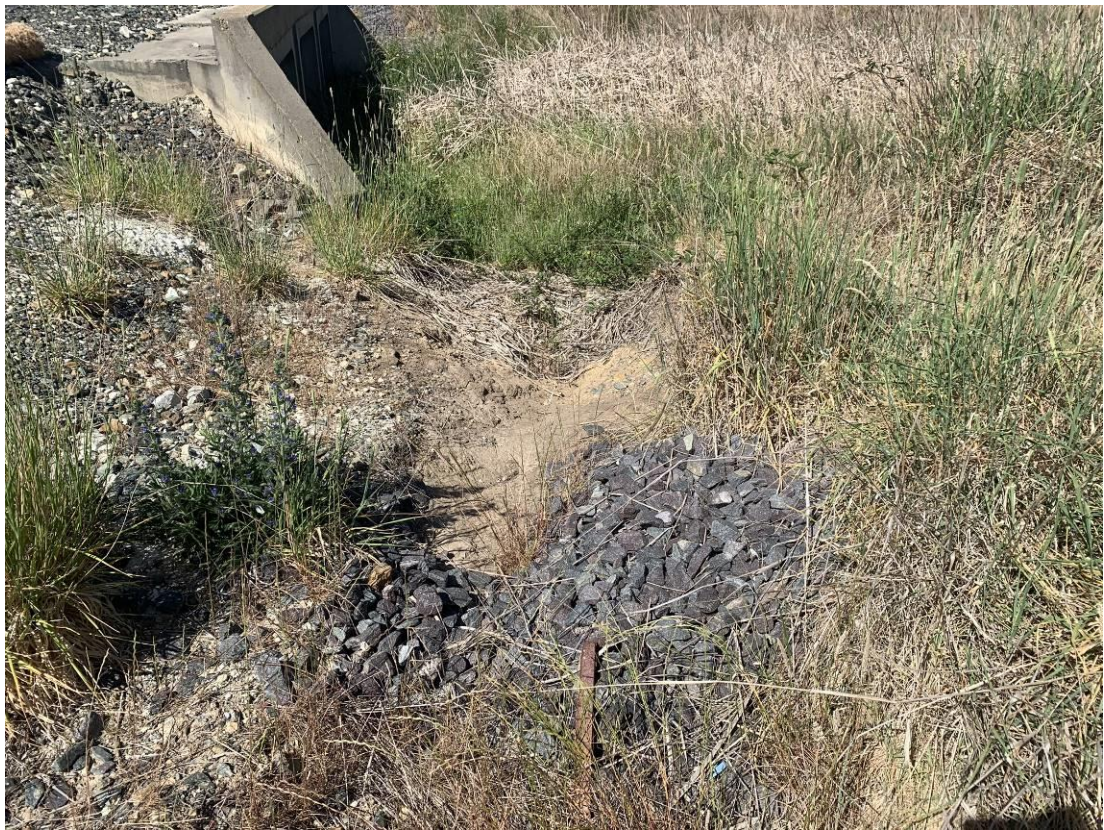
Photo 25: Additional photograph of southern rock armour. Pictured is the closest rock armour to the culvert opening appearing misshaped and with a build-up of sediment.
