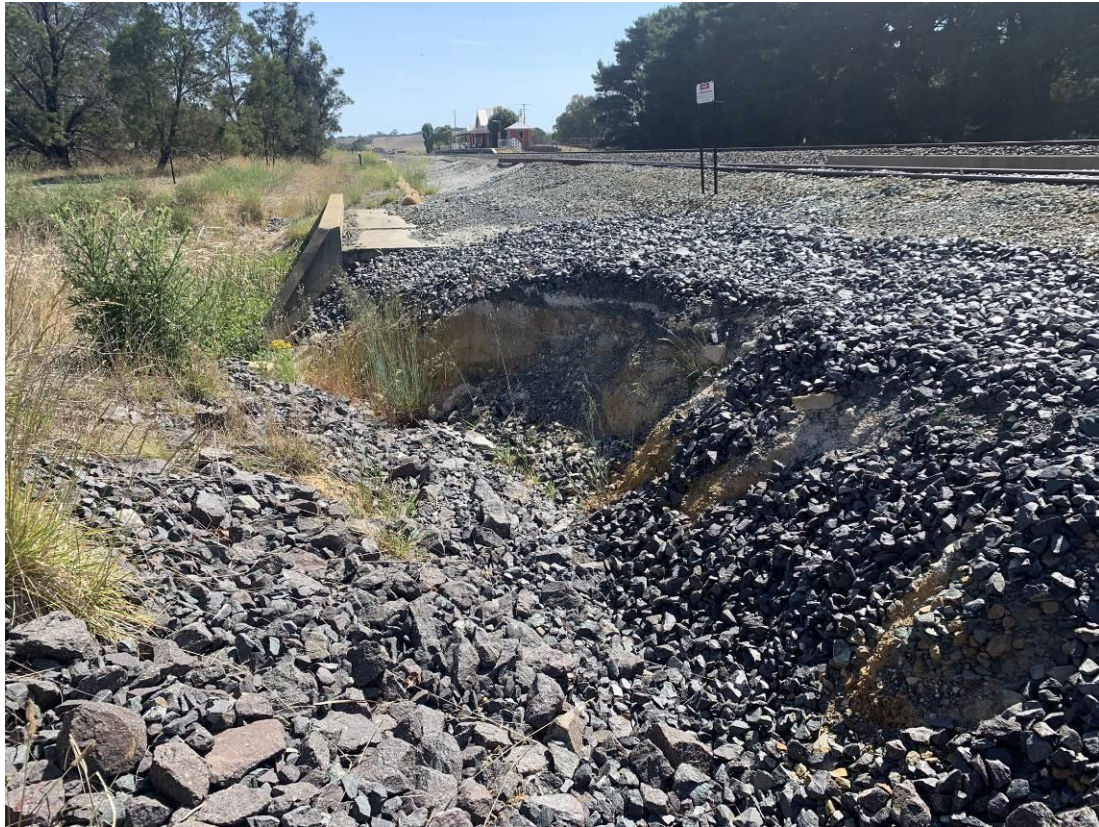
Photo 21: Visible evidence of erosion due to loss of ground cover (ballast material) upgradient of southernmost culvert. Remaining material is stable and no major further erosion is noted since last inspection (19/10/11). Facing north-east.
