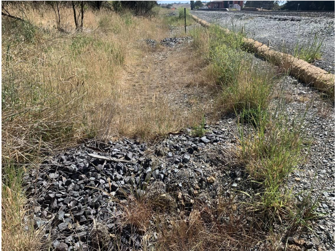
Photo 23: Southern culvert upgradient of railway tracks rock armour for sediment control.
