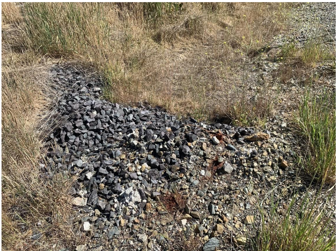
Photo 24: Additional photograph of southern rock armour with a build-up of debris.
