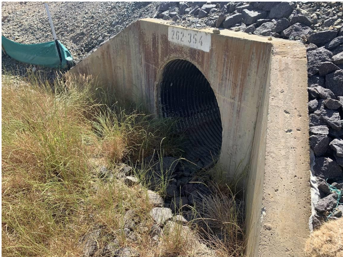
Photo 5: Middle culvert upgradient of the railway line with no flowing or pooled surface water. No observed build-up of sediment on rocks or in culvert. Rock armor and natural vegetation providing sediment control for surface water.
