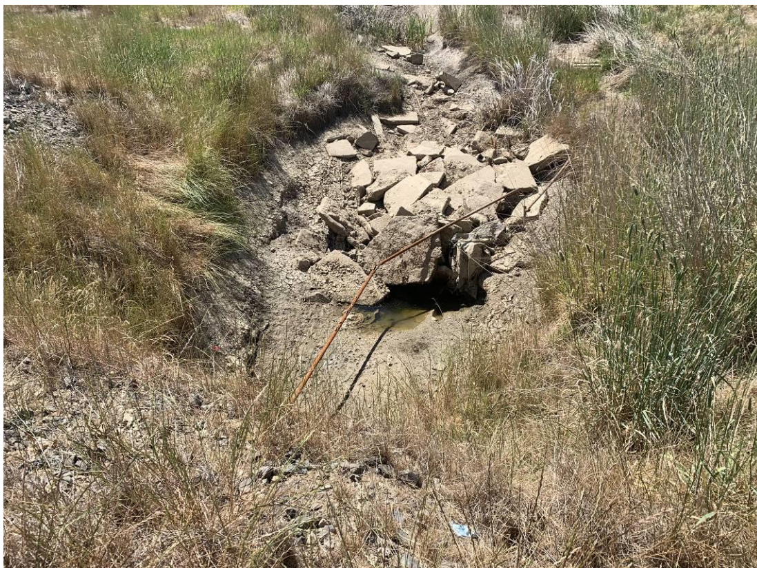
Photo 6: Middle culvert downgradient of the railway line with no flowing surface water. Soil dampness and a small pool of water is present. Water appeared to have low turbidity. No evidence of surface water currently running off site at middle culvert.
