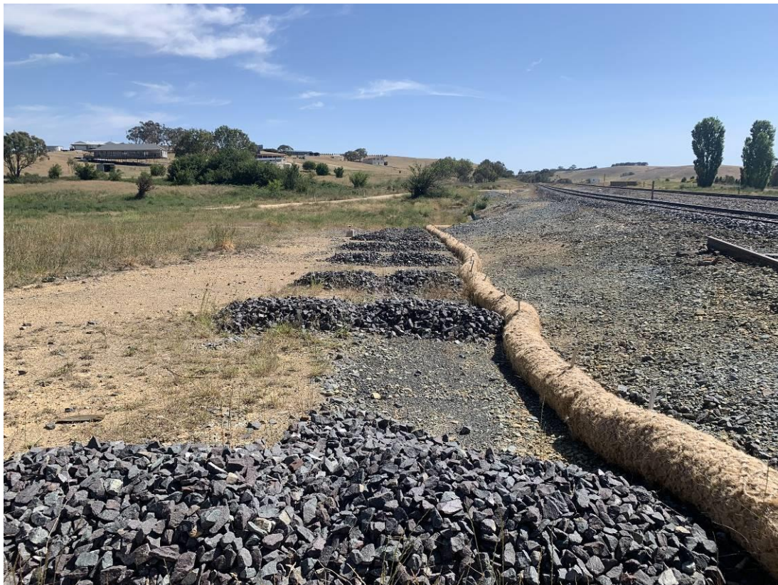
Photo 13: Rock checks running alongside former Woodlawn siding towards the middle culvert. No evidence of sediment build-up in rock armour or coir sediment control logs.
