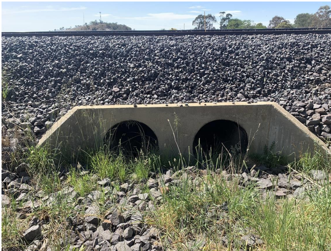
Photo 7: Northern culvert upgradient of the railway line with no flowing or pooled surface water. No observed build-up of sediment on rocks or in culvert. Rock armor and vegetation providing sediment control for surface water.
