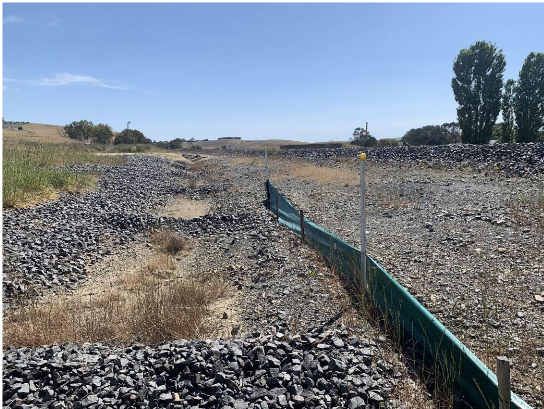
Photo 15: Rock armour west of the rail formation running from the middle to the north culvert. Some sediment visible on rock armour. Facing north-east.
