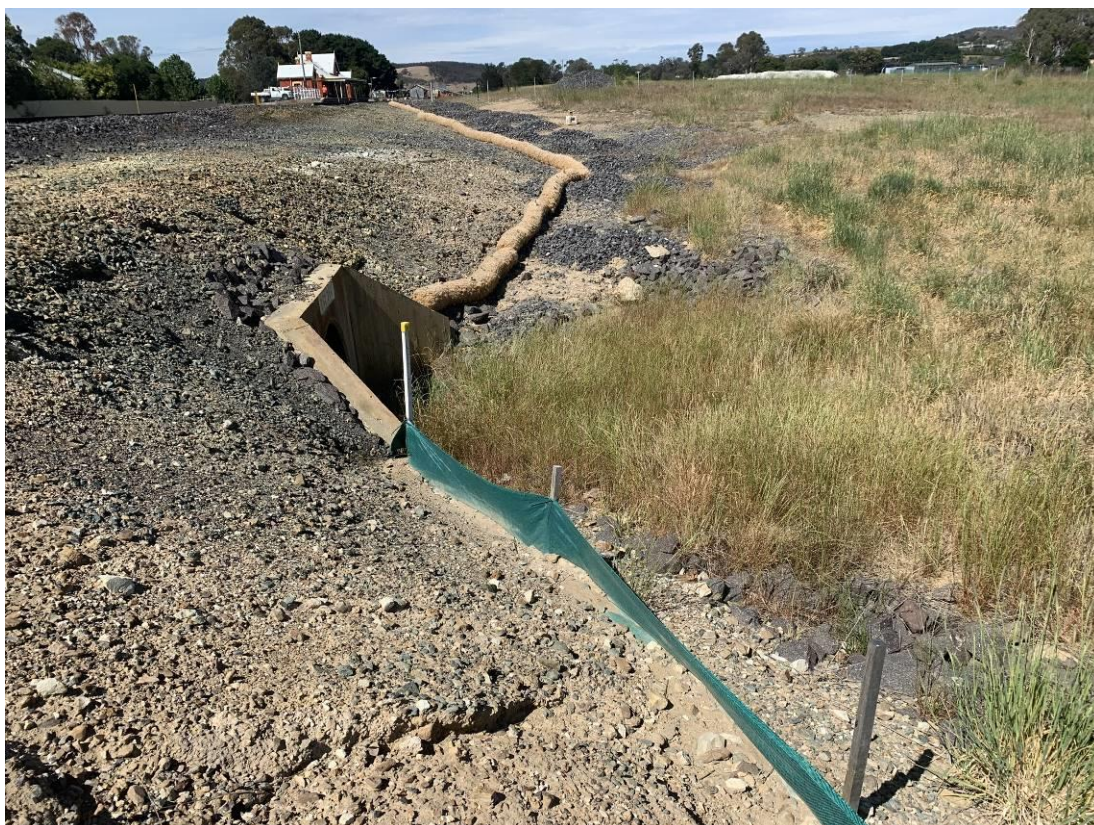
Photo 14: Upgradient of middle culvert facing east. Silt fencing is clear with some sediment visible.
