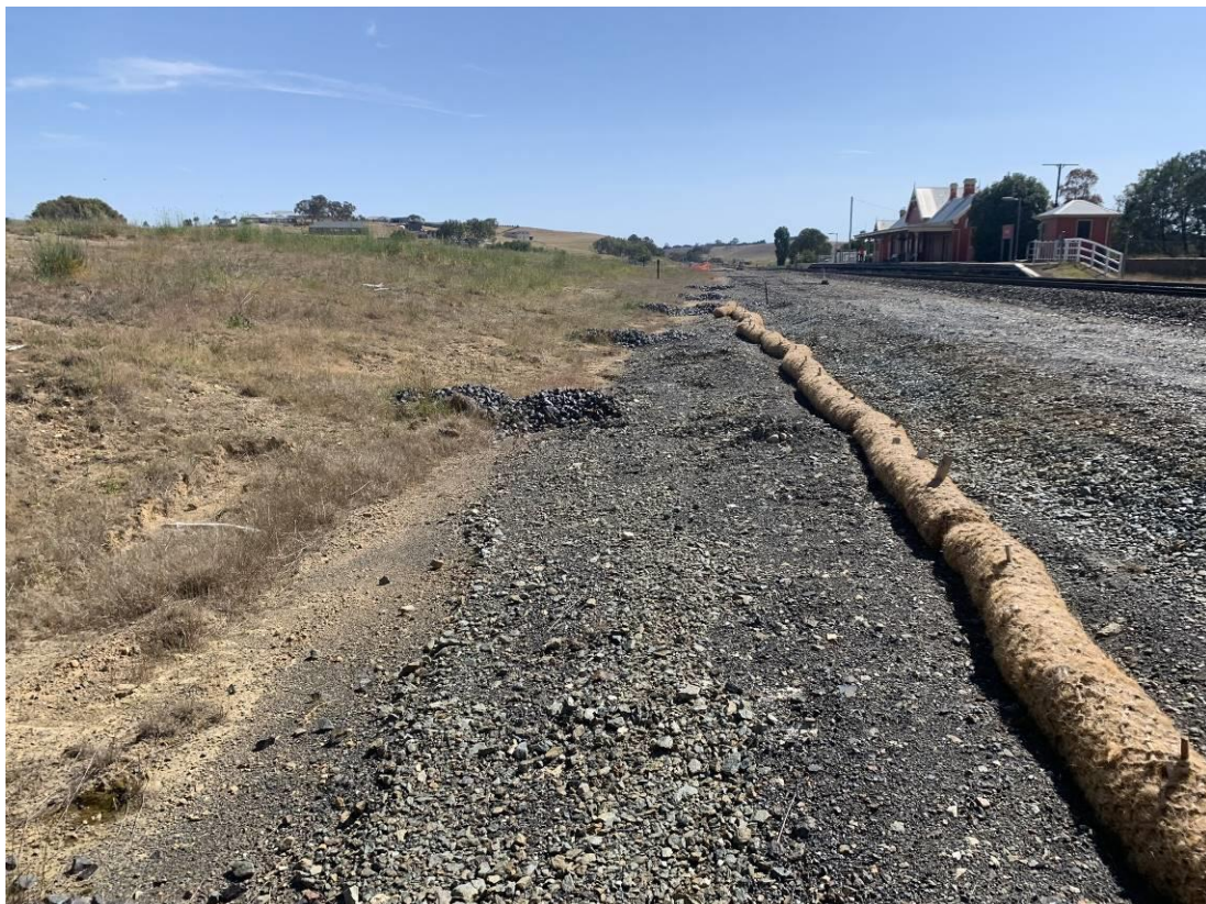
Photo 12: Rock checks running along former Woodlawn siding and between southern and middle culverts. Previously silt fencing, since replaced by Coir sediment control logs.
