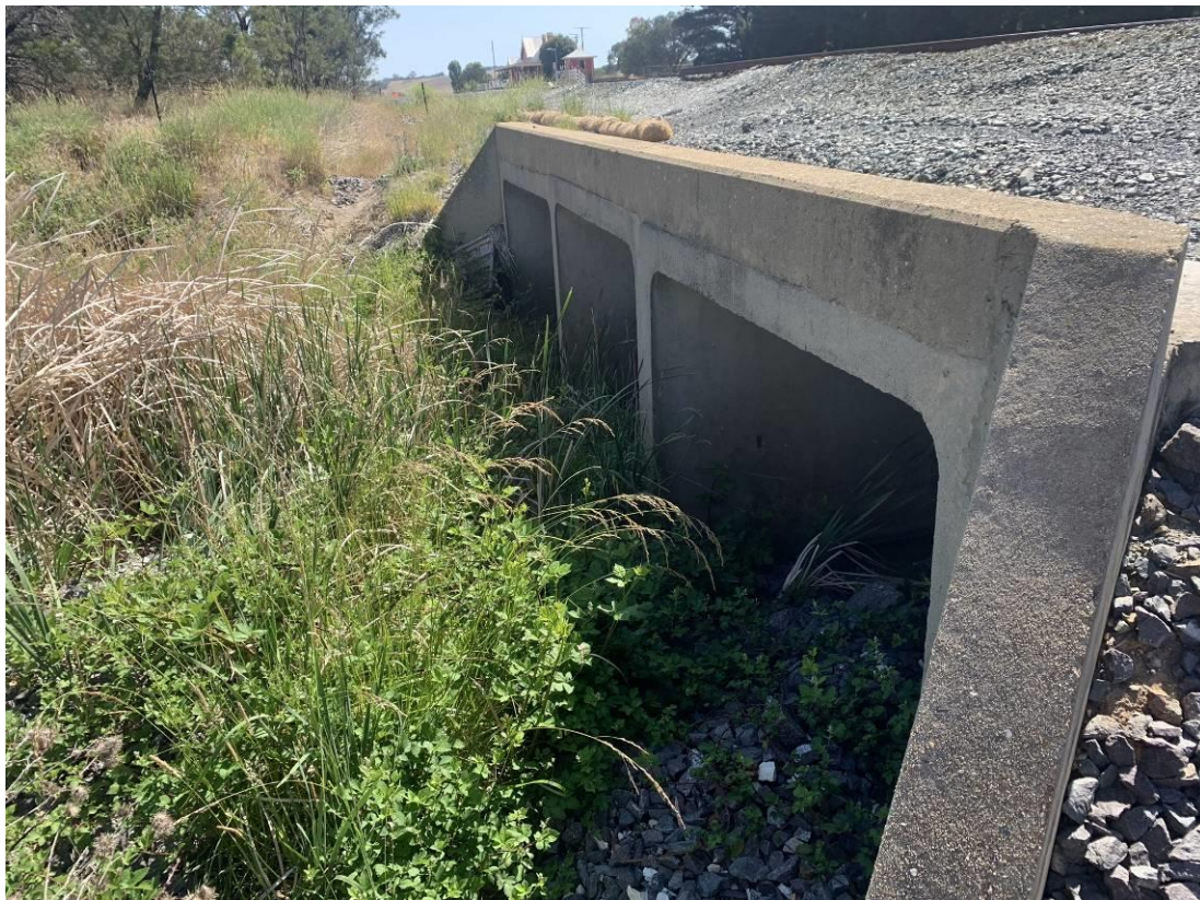
Photo 3: Southern culvert upgradient of the railway line with no flowing surface water. No observed build-up of sediment on rocks. Rock armor and natural vegetation providing sediment control for surface water.
