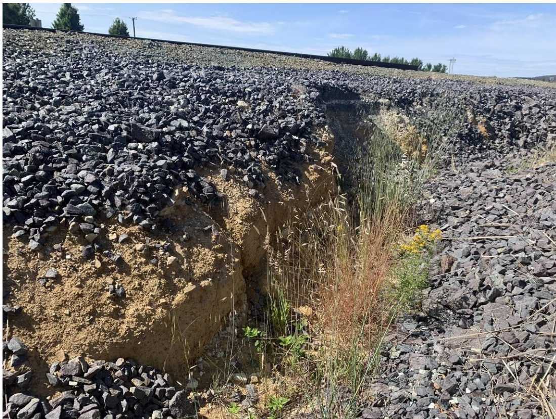
Photo 22: Additional photograph of erosion upgradient at southern culvert.
