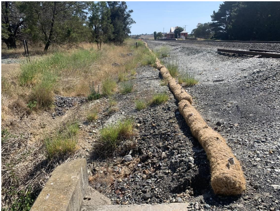
Photo 11: Upgradient of southern culvert showing Coir sediment control logs, used as control measures for sediment control. Facing north-east.
