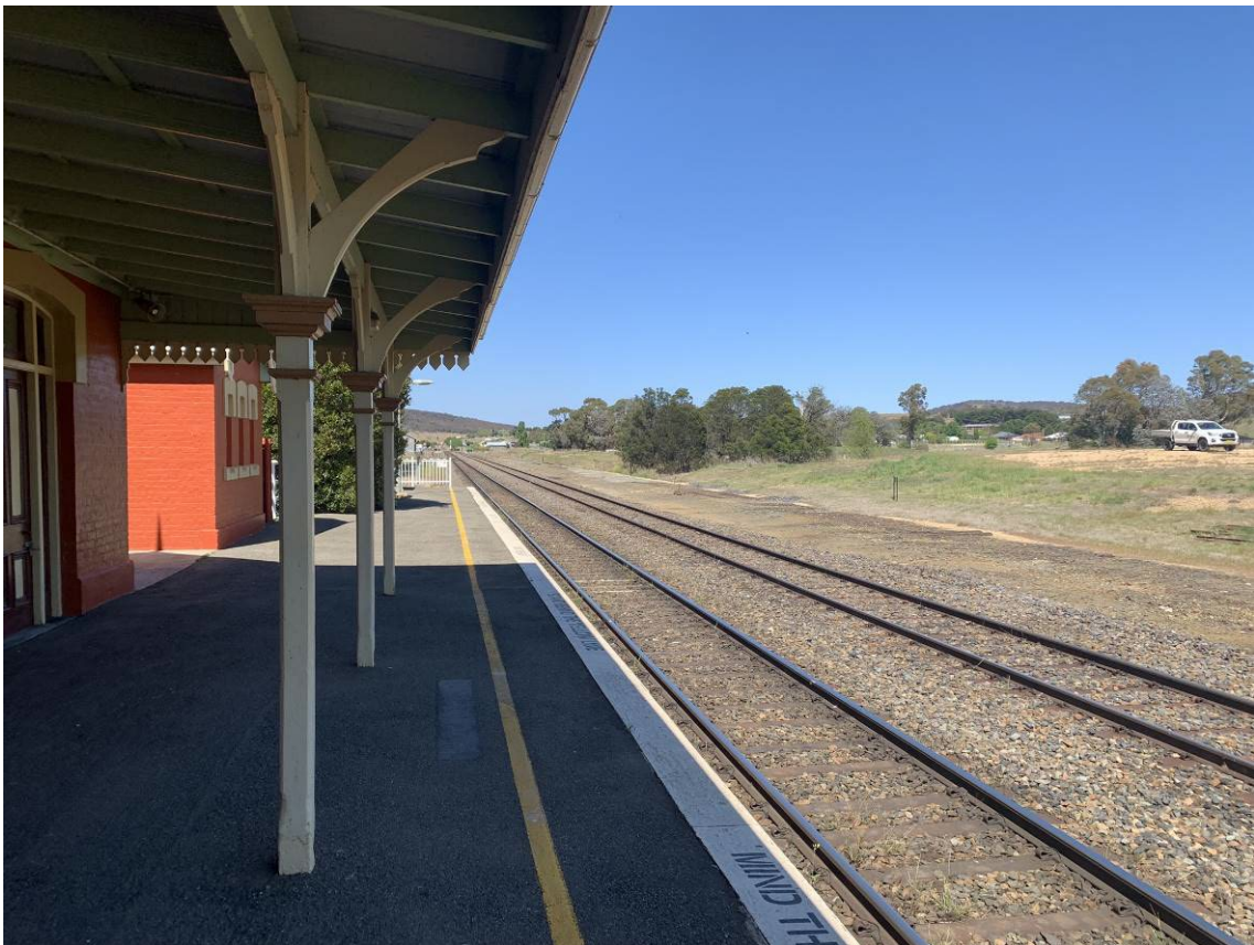
Photo 1: Picture at halfway point at Tarago railway station platform facing south-west. No airborne dust visible.
