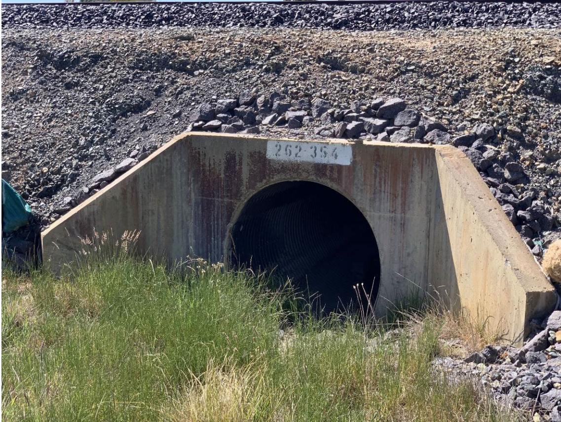
Photo 13: Upgradient of Middle culvert showing no flowing or pooled water. No evidence of sediment build-up in culvert.
