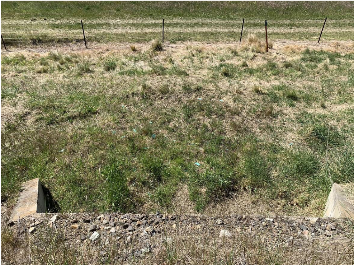
Photo 7: Downgradient of northernmost culvert showing evidence of no surface water runoff from site into neighbouring property.
