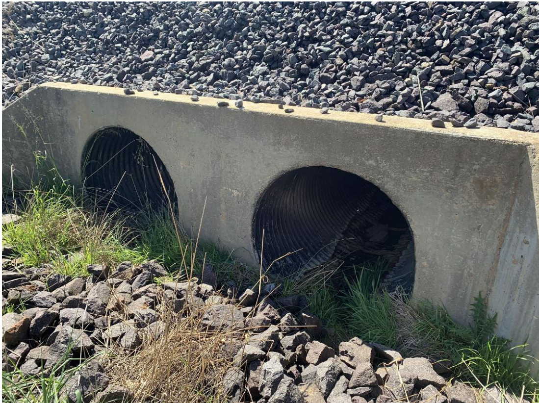
Photo 16: Upgradient of northernmost culvert. No evidence of surface water run off on site. No evidence of sediment buildup on rocks. Rock armor and natural vegetation allow for sediment control in surface water.
