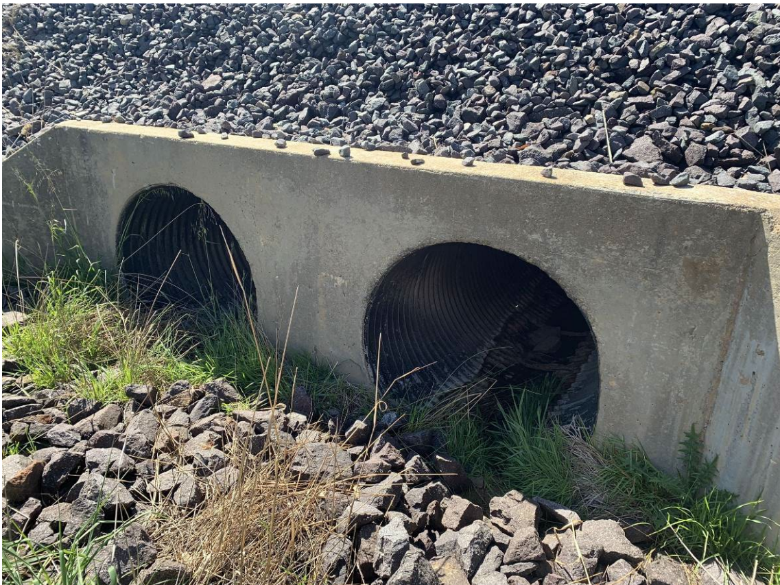
Photo 8: Upgradient of northernmost culvert showing evidence of no surface water present.
