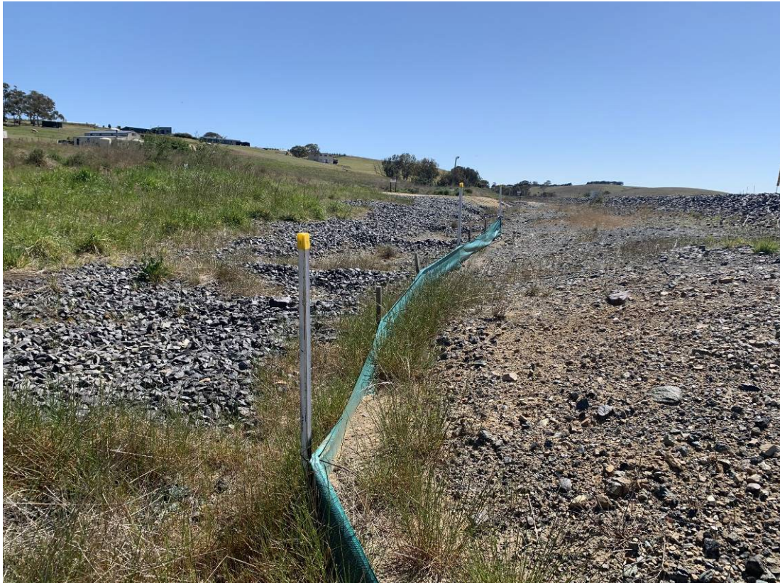
Photo 15: Rock armour upgradient of trainline running from the middle to the north culvert. Some sediment visible on rock armour. Facing north-east.
