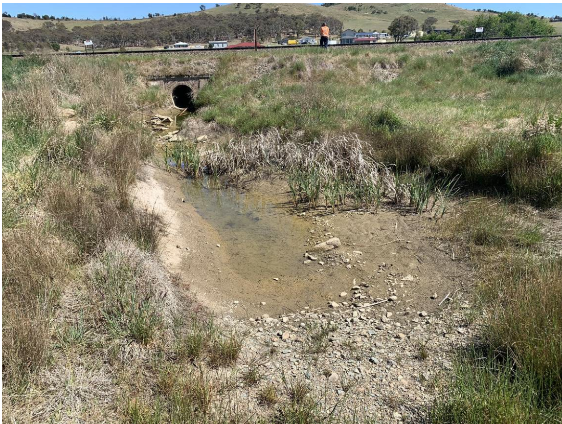
Photo 4: Downgradient of middle culvert showing brown turbid water on site. Surface water levels notably less than in the previous inspection (14/09/23). No surface water currently running off site at middle culvert.
