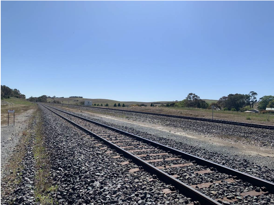
Photo 22: No pooled water adjacent to railway tracks. Facing North-East.
