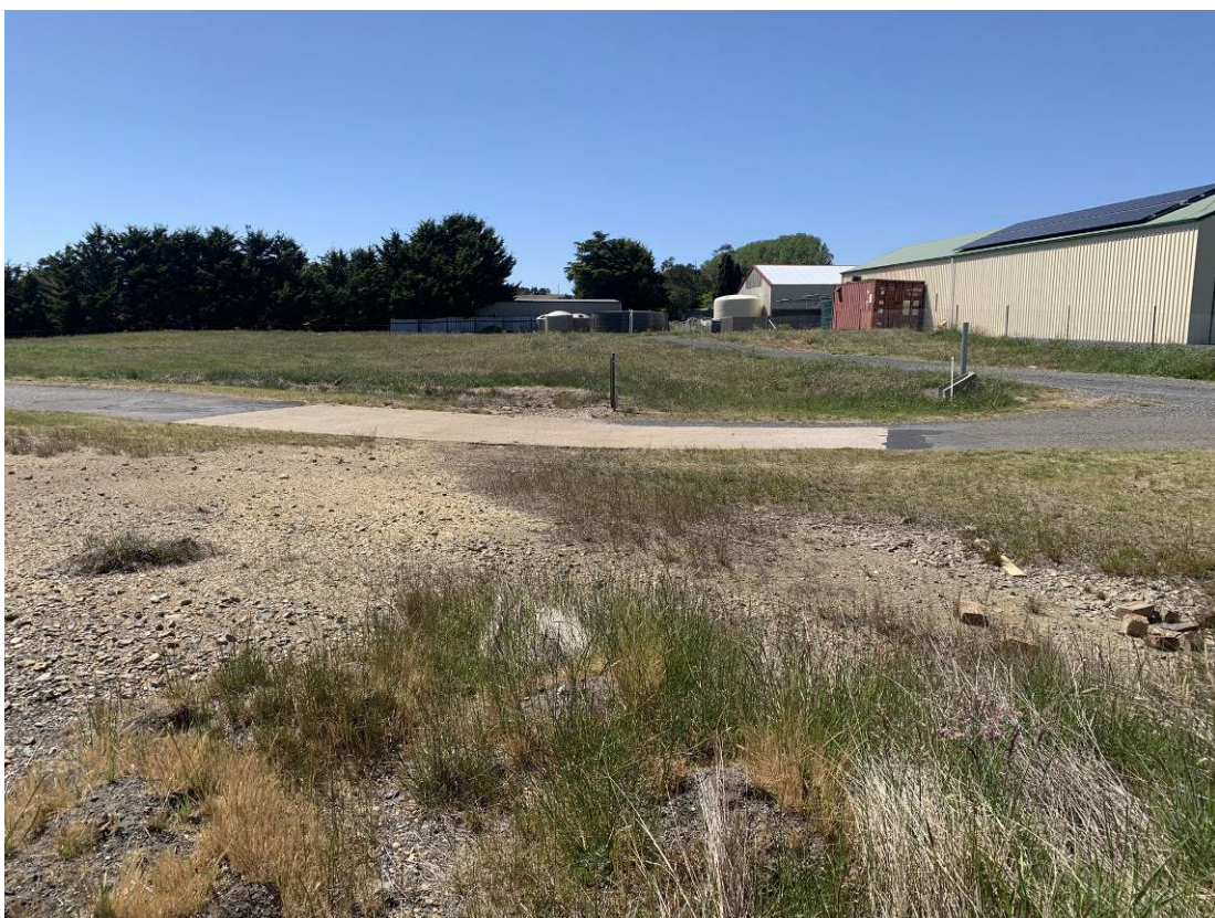
Photo 6: Causeway downgradient of middle culvert showing no evidence of current surface water moving off site. No visible sediment on road or vegetation nearby from sediment water was running off site in between inspections.
