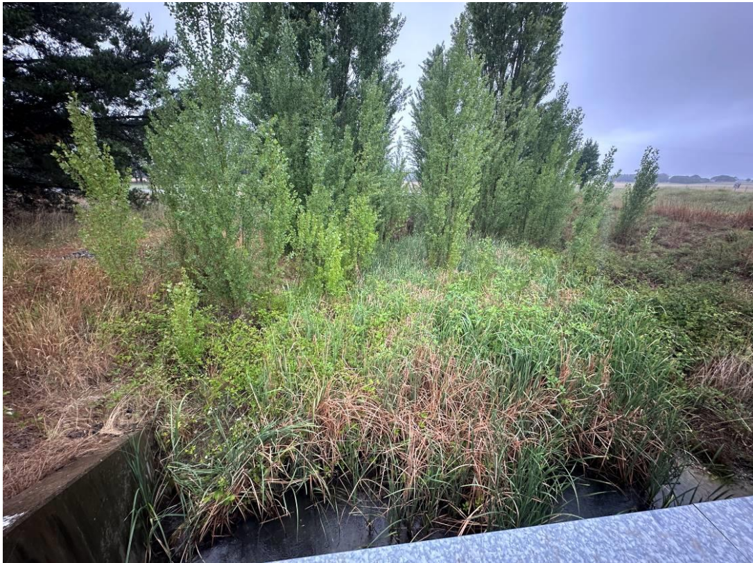
Photo 4: Downgradient of southern culvert with surface water flowing offsite. Surface water is clear with low turbidity.
