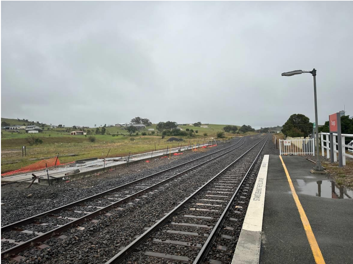
Photo 1: Picture at northern end of Tarago railway station platform facing north. No airborne dust visible.
