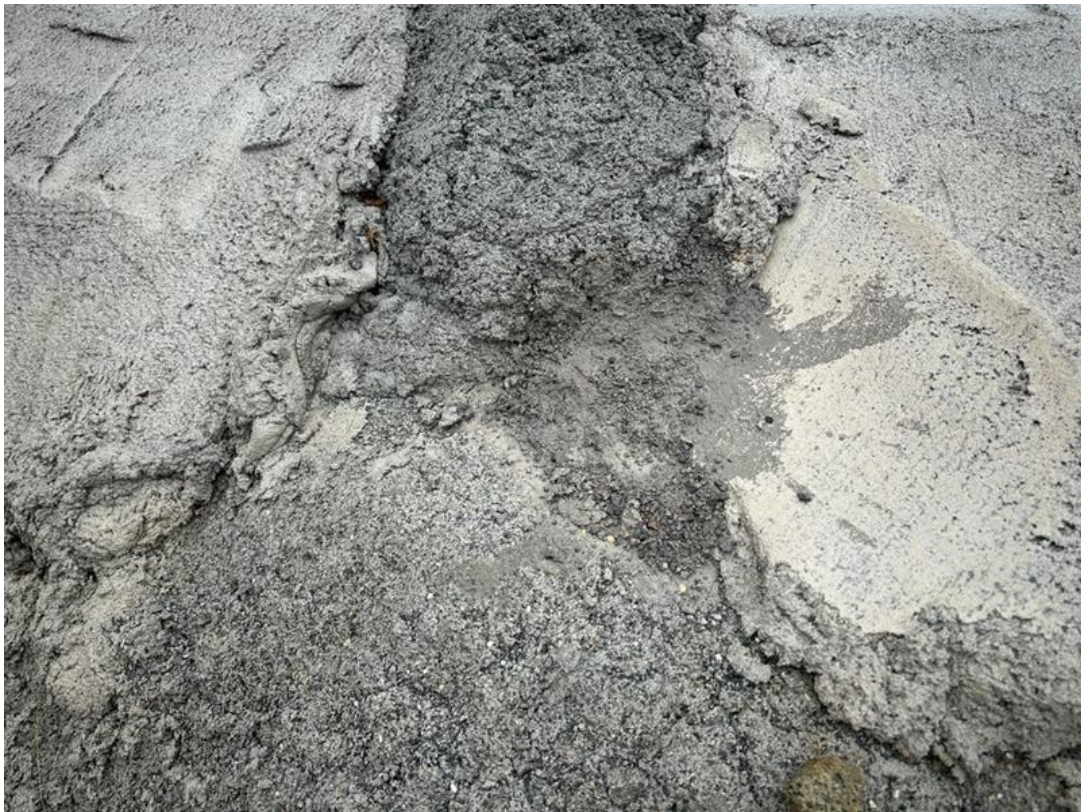
Photo 12: Geofabric marker layer visible in stockpile capping in previous inspection. Covered with cement by UGL Representatives as advised.
