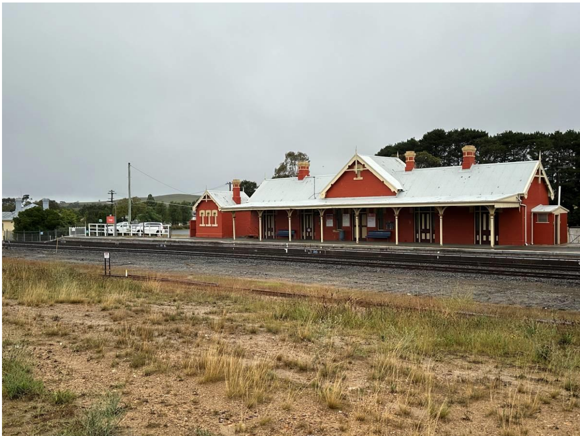
Photo 2: Picture at of Tarago railway station. No airborne dust visible.
