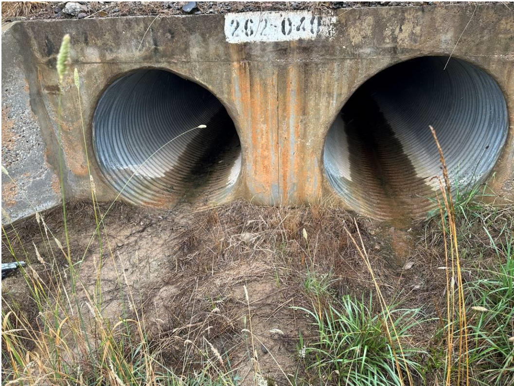
Photo 10: Downgradient of northernmost culvert with no flowing surface water.
