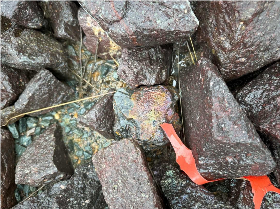
Photo 17: Minor suspected hydrocarbon spill noted on wet ballast material on site. Located between rail lines near drain between middle and northernmost culverts.
