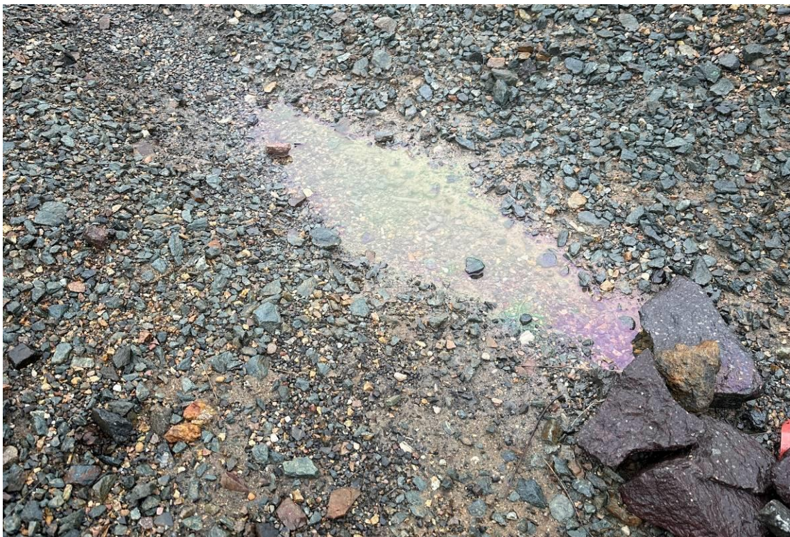
Photo 16: Minor suspected hydrocarbon spill noted in pooled surface water on site. Located between rail lines near drain between middle and northernmost culverts.
