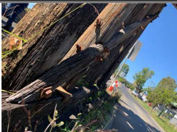
Pier 5 southern diagonal brace small section size lower end
