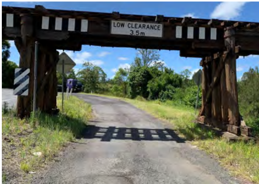
Photo 28: Road width – Alexandra Parade bypass viaduct
