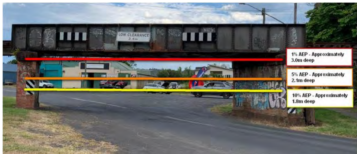
Figure C-7 Union Street – Flood levels (Source: LCC)
