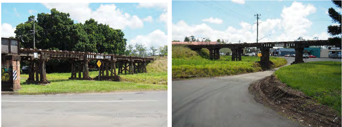
Figure 2-7 Union Street north timber approach spans (Source: FBE)
