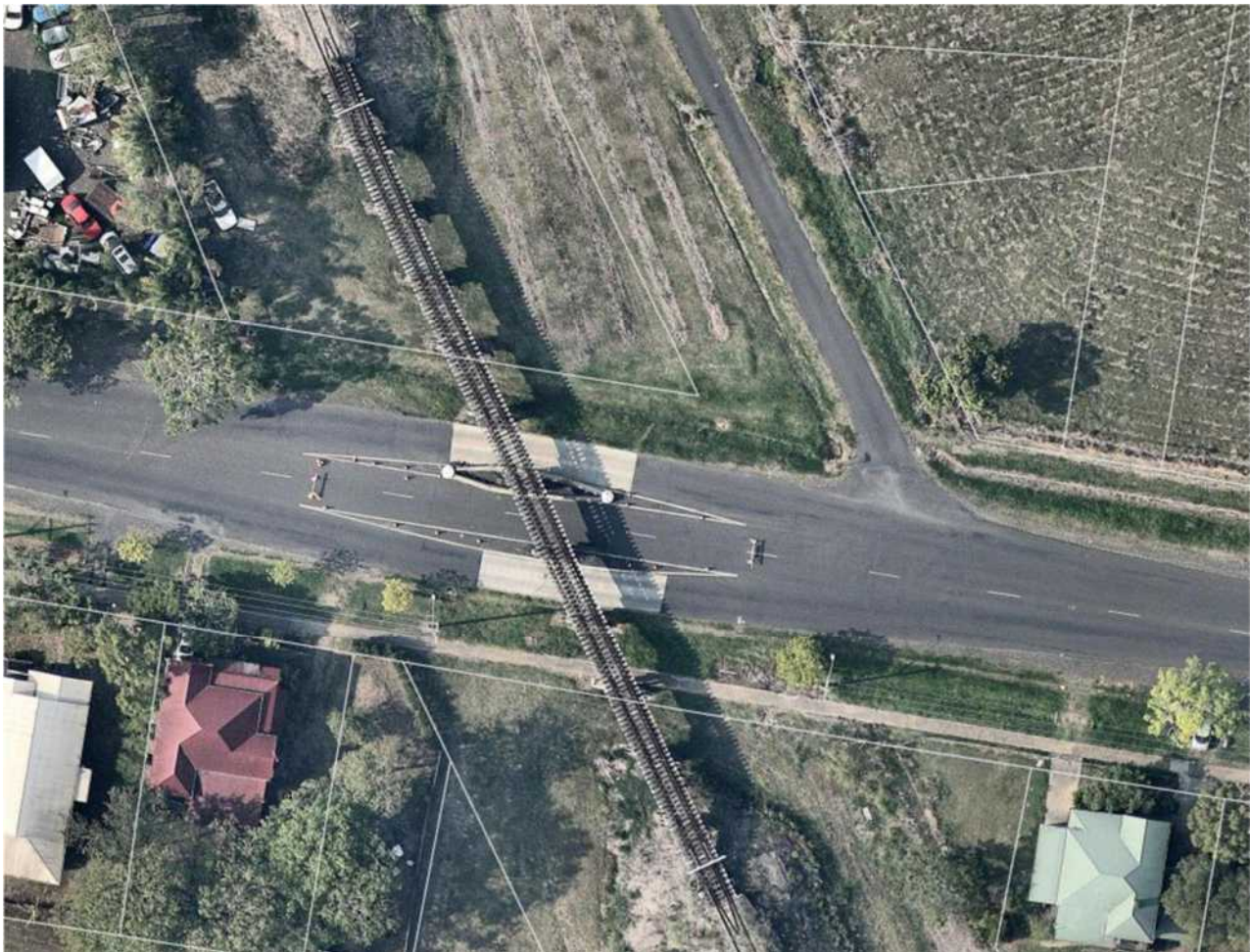
Figure 4-1 Aerial image of Terania Street Underbridge (Nearmap, 2020)
