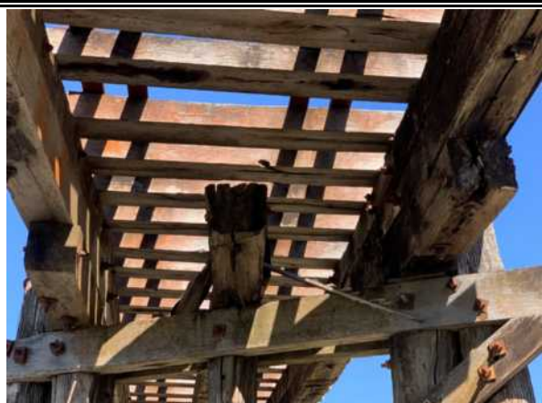
Pier 5 corbels northend general view
