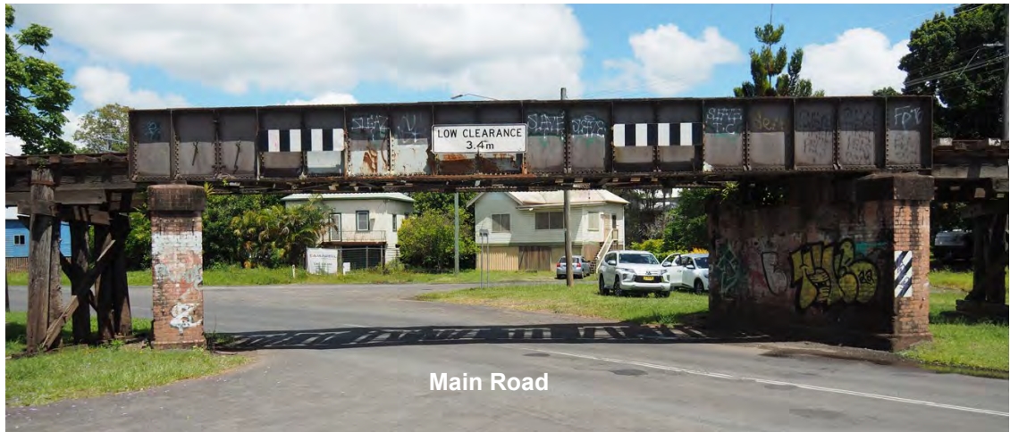
Figure 9-2 Union Street Underbridge road clearance over main road (Source: FBE)
