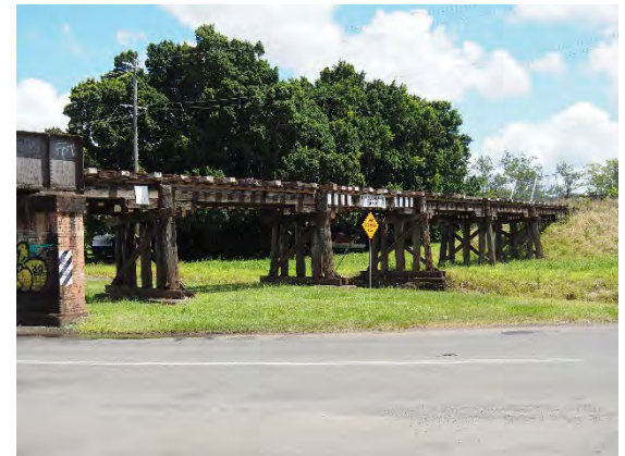
Figure 4-4 Union Street metal and timber spans (Source: FBE)
