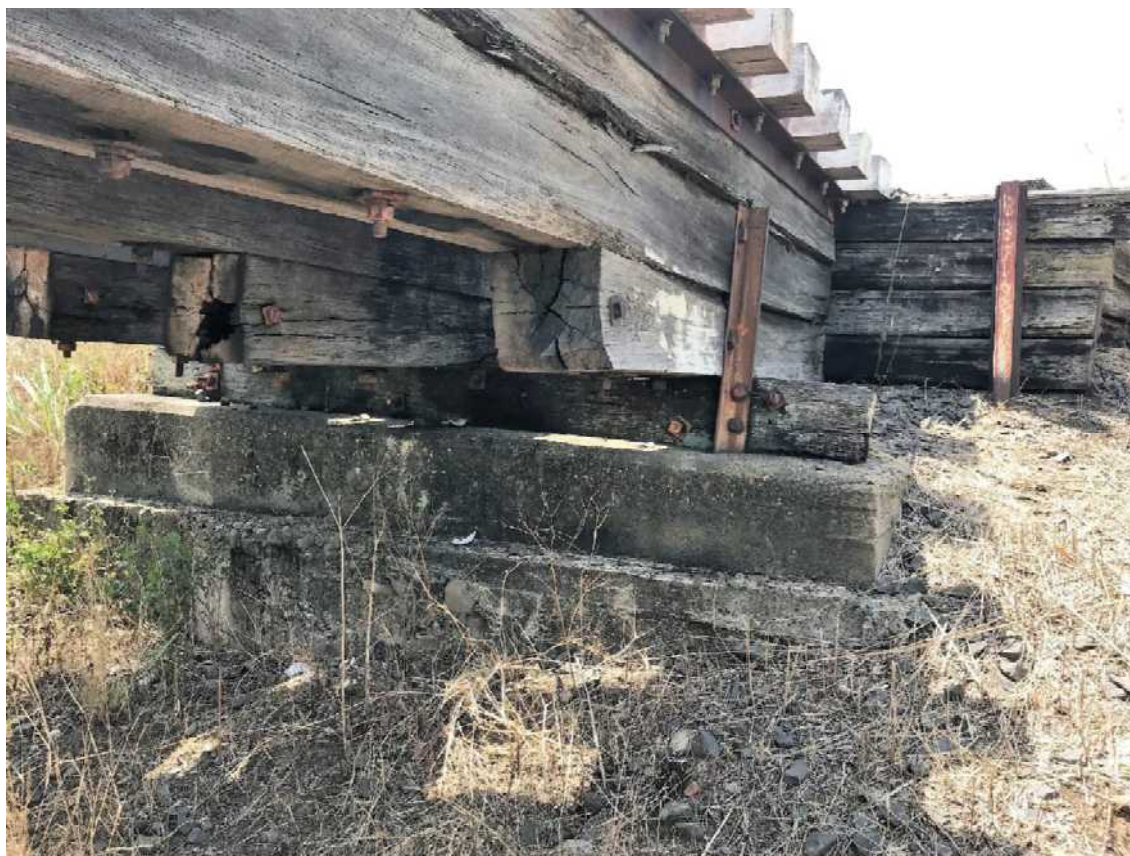
Figure 3-5 General view of Abutment 2 (north)
