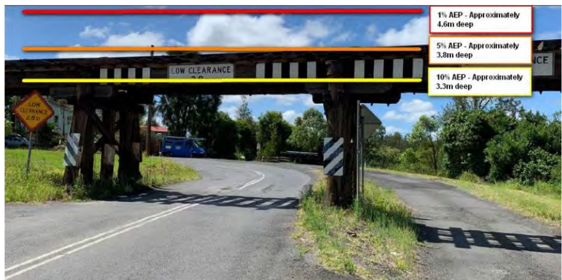
Figure 6-1 Alexandra Parade Underbridge flood levels (Source: LCC)
