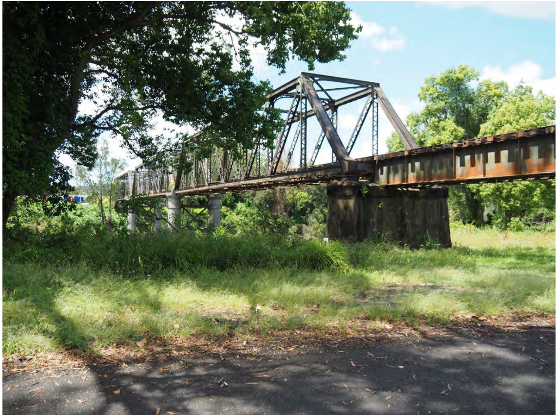
Figure B-6 Crane Street – Pratt truss east elevation, typical condition (Source: FBE)
