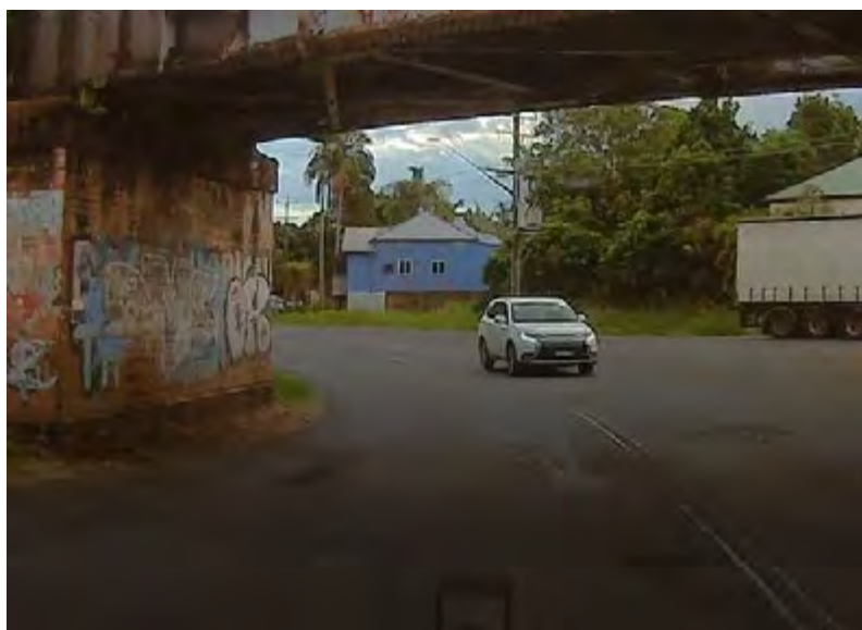
Photo 2: Minimal edge clearance - Union Street viaduct
