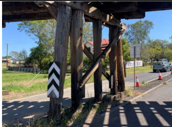
Pier 5 general view
