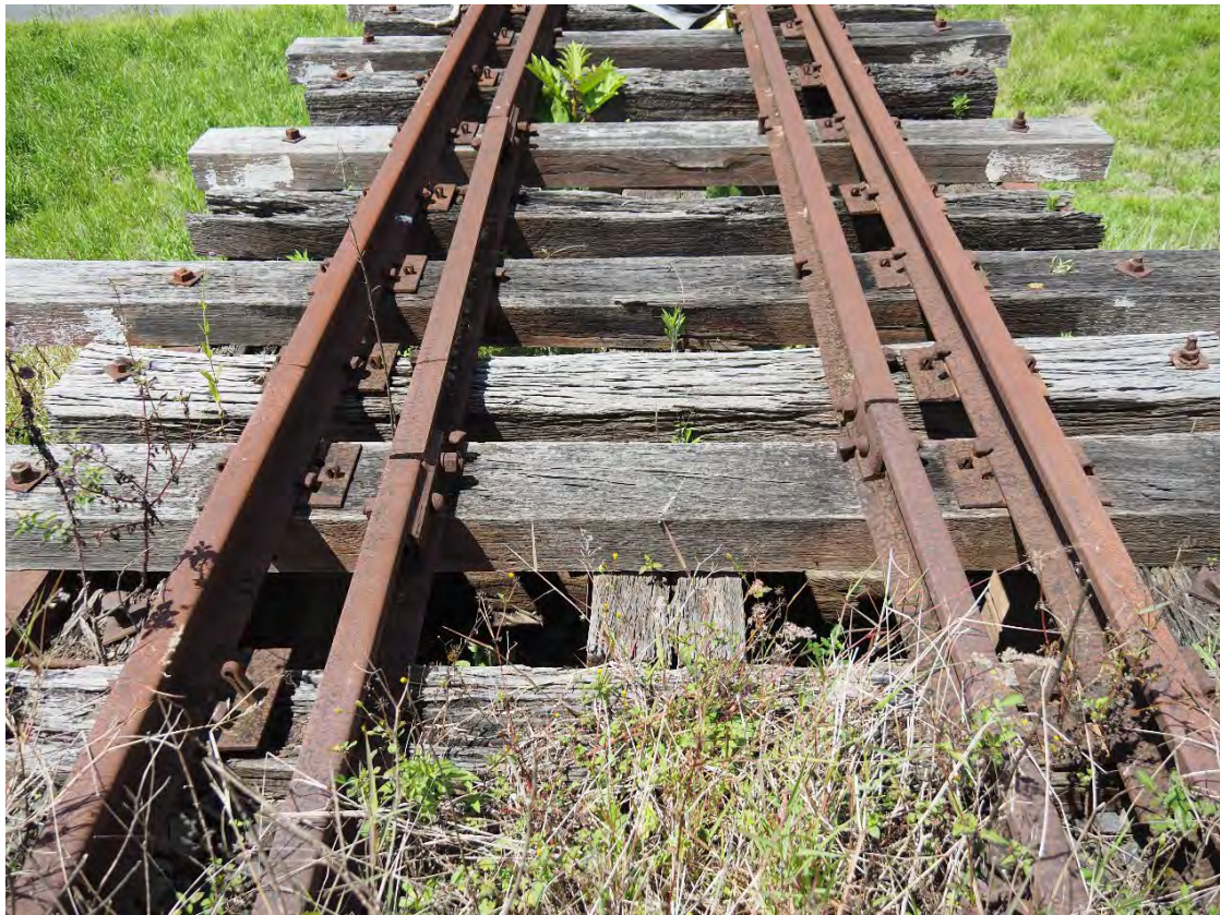
Figure B-21 Union Street – View overlooking south, typical condition (Source: FBE)
