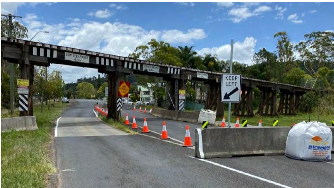
Figure 2-5 Terania Street Underbridge east elevation (Source: FBE)
