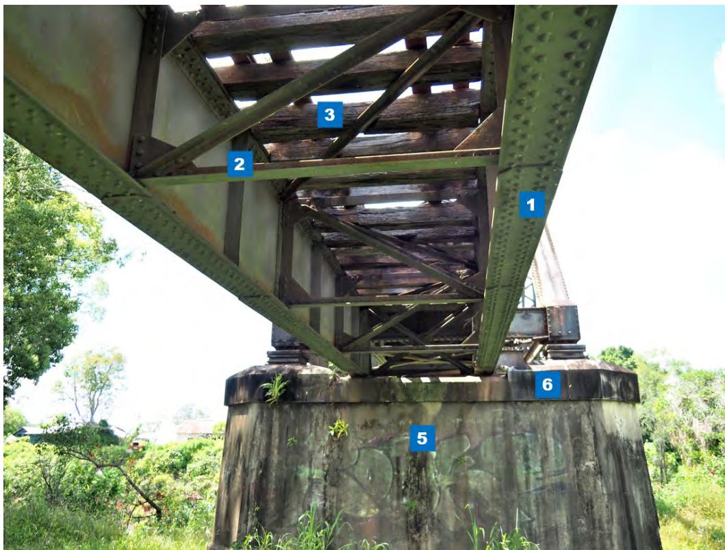
Figure A-3 Crane Street Underbridge elements (Source: FBE)
