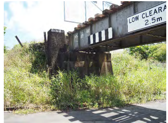
Figure 4-2 Terania Street typical span and trestle support condition (Source: FBE)
