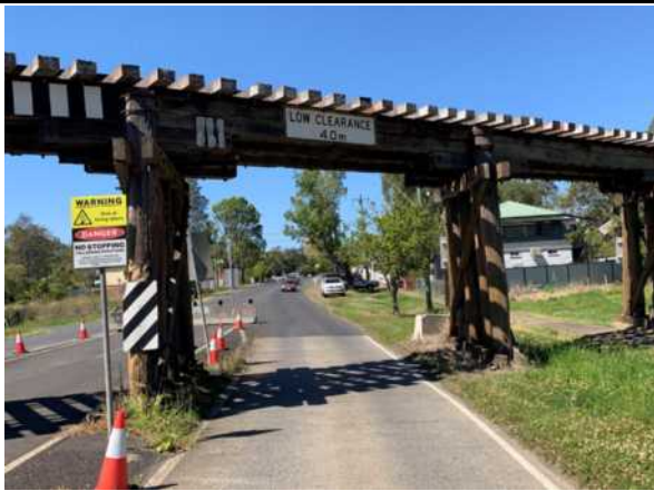
Span 5 west view
