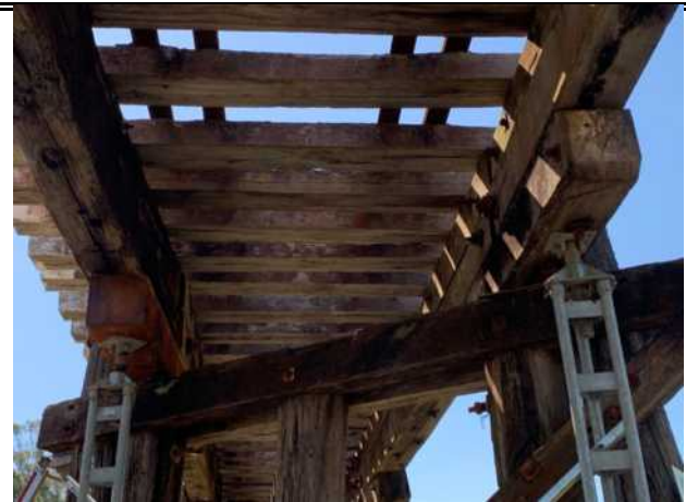
Pier 6 corbels south end good condition
