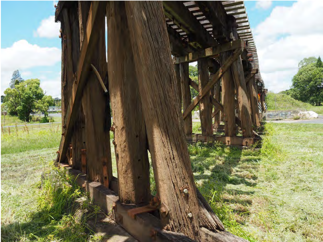
Figure B-15 Terania Street – Splitting & weathering of piles at Pier 11 (Source: FBE)
