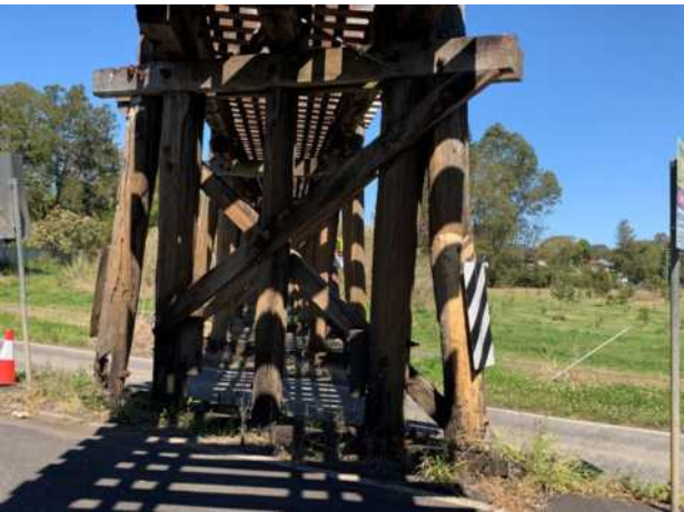
Pier 4 north view
