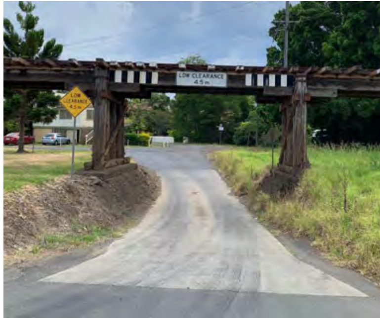
Photo 4: Road width - Frank Street viaduct
