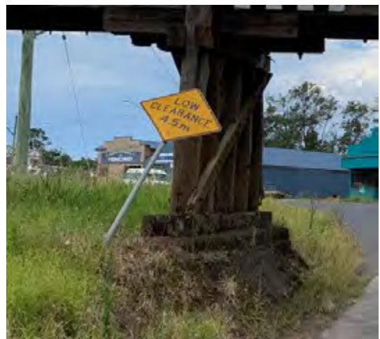
Photo 6: Damaged signs - Union Street viaduct
