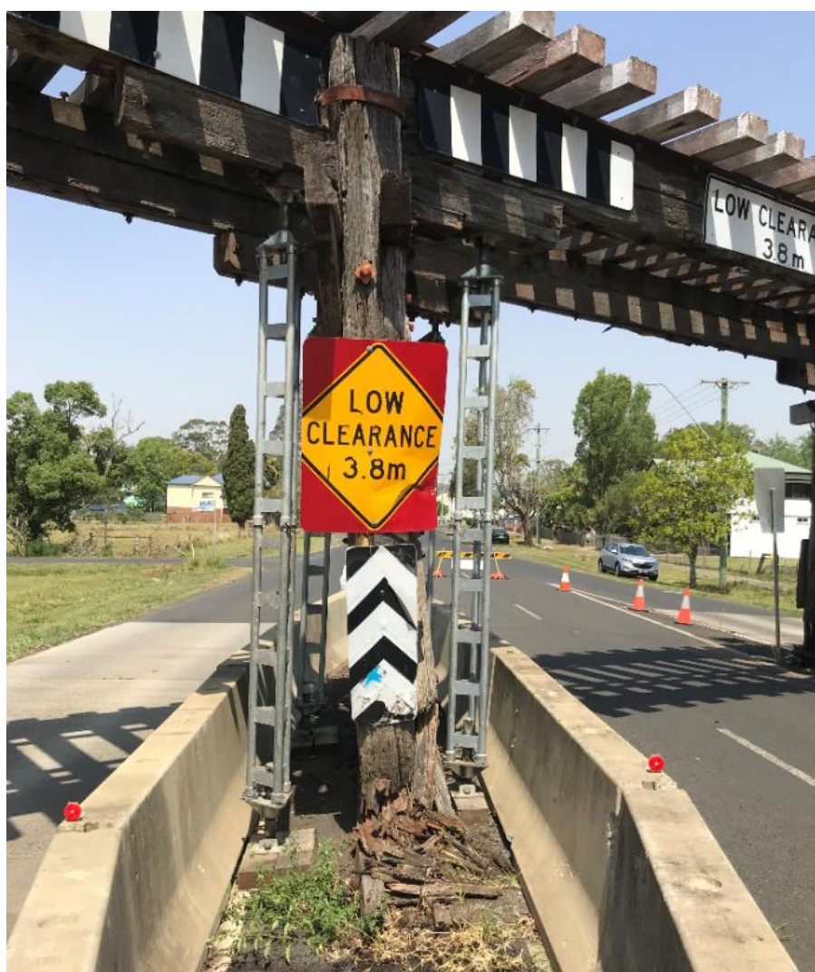
Figure 4-3 Trishore support to damaged Pier 6
