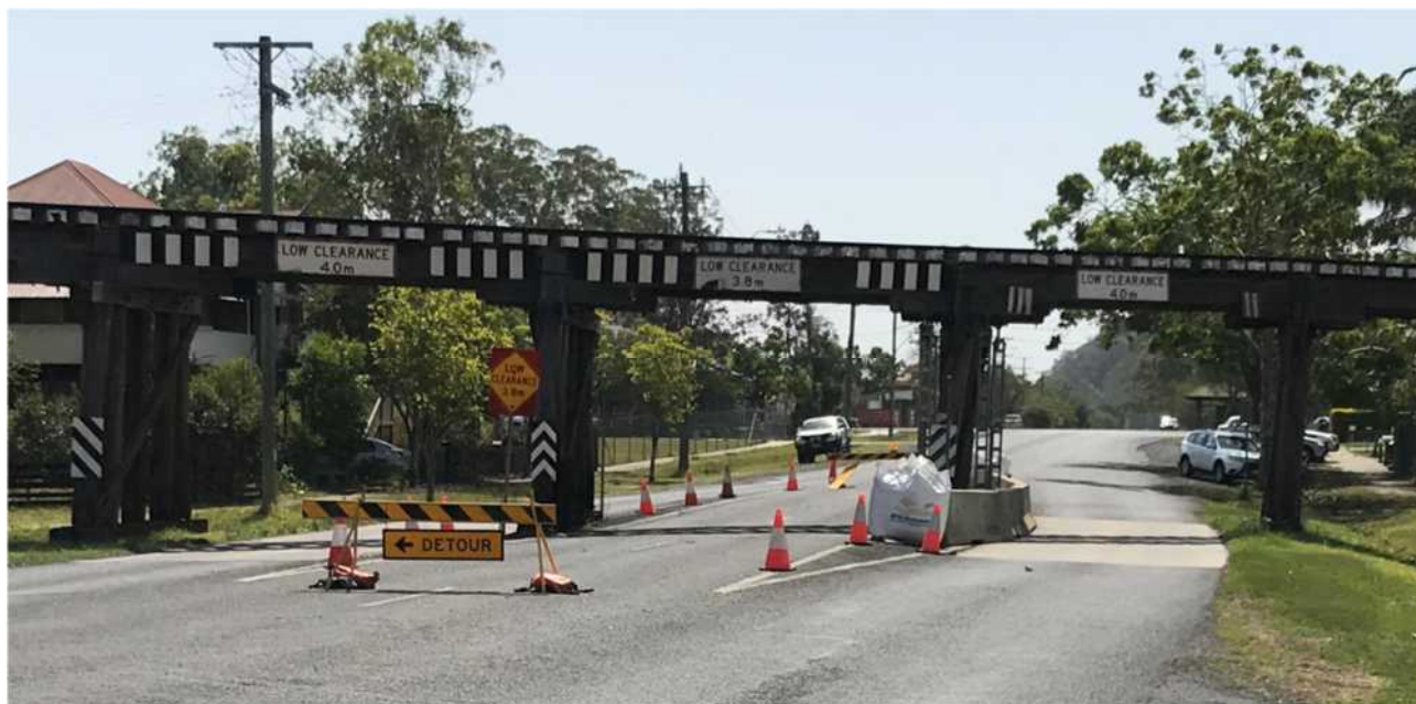
Figure 4-2 Underbridge facing west
