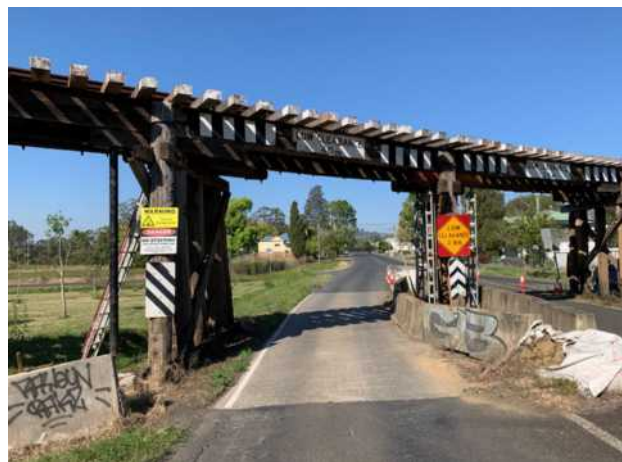
Span 7 west view
