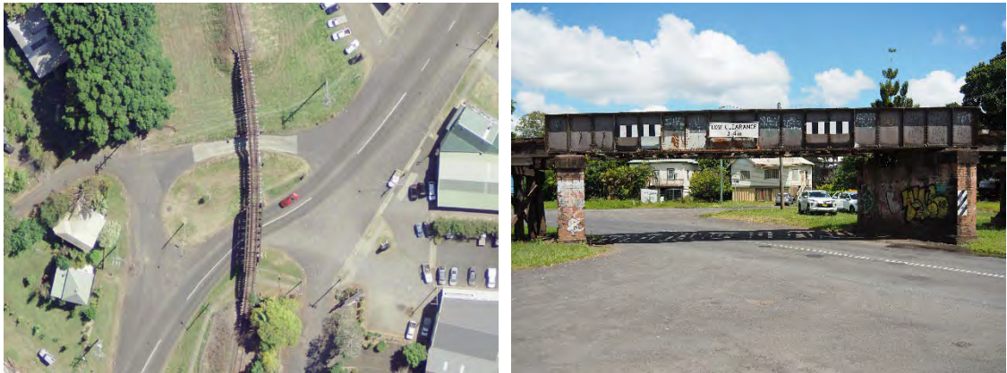
Figure 2-6 Union Street Underbridge aerial view and metal span elevation (Source: FBE)
