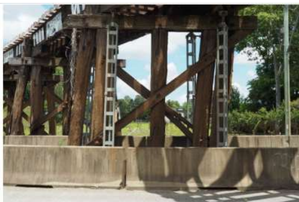
Figure B-13 Terania Street – Evidence of global rotation of Pier 6 together with failed pile (Source: FBE)
