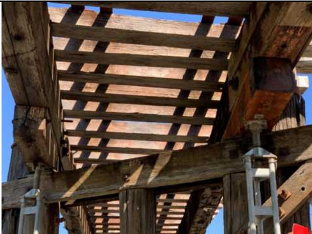
Pier 6 corbels north end good condition
