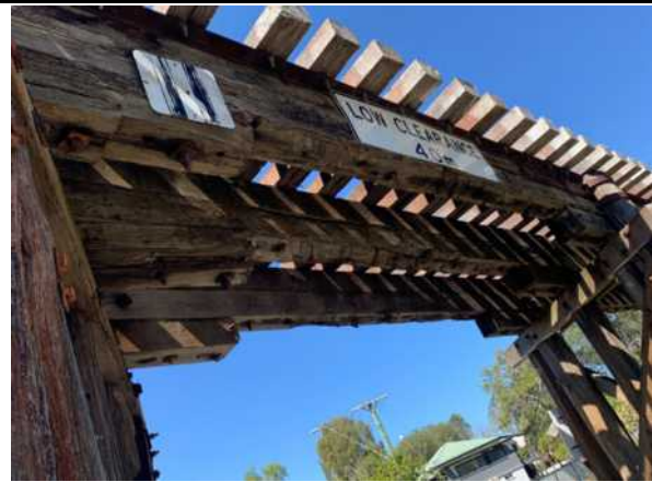
Span 5 general view of girders
