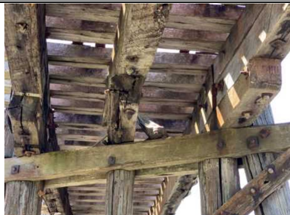
Pier 5 corbels southend
