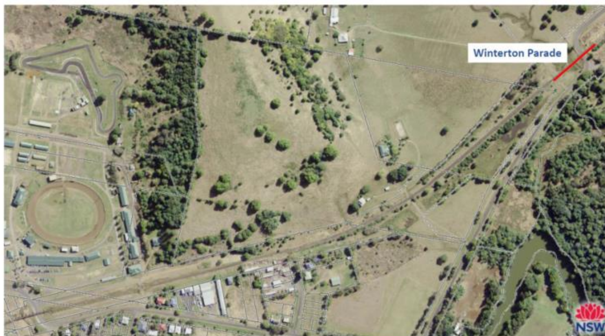
Plate 4: Additional bridges proposed for demolition in Lismore CBD (Source: UGLRL)
