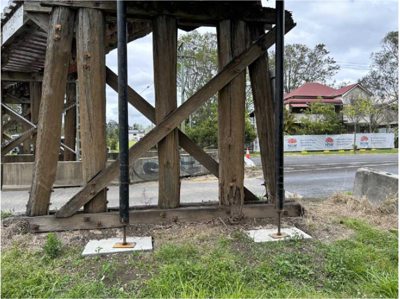
Figure 5: Pier 7 – Props installed
