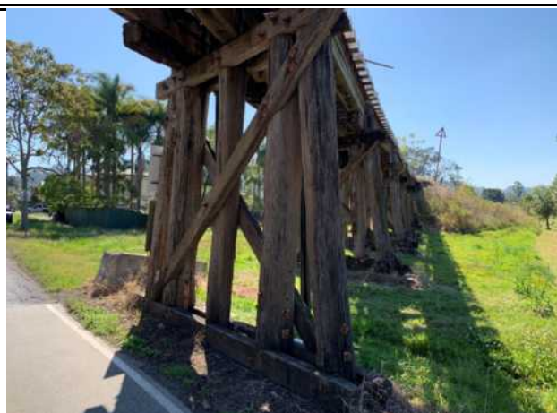
Pier 7 piles general view
