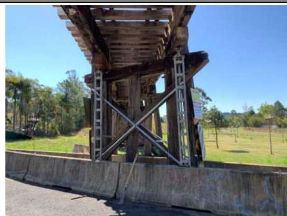
Pier 6 temporary support under outer corbels
