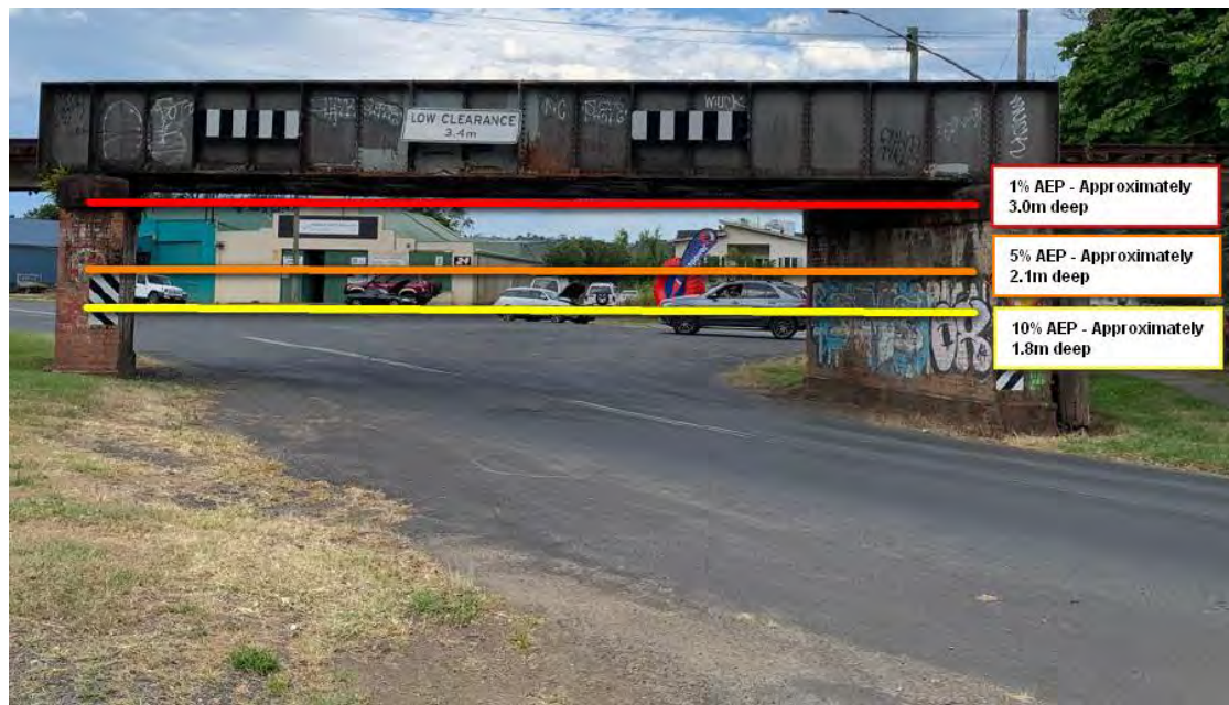
Figure 1: Union Street Bridge with Flood Depths
