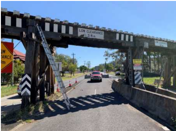
Span 6 east view
