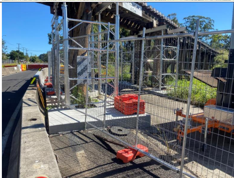
Photo 5: Safety scaffolding; note poured concrete bases, which will require removal following demolition (est. 4-5 days)
