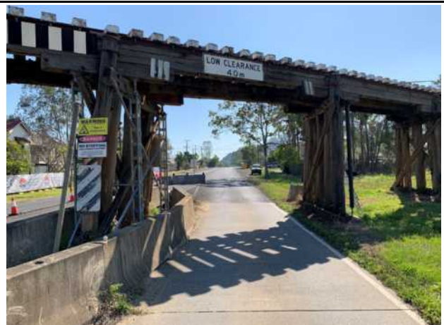
Span 7 east view
