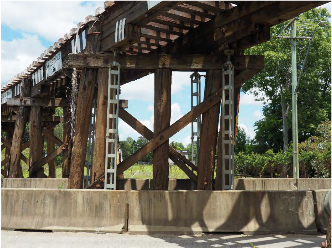
Figure B-13 Terania Street – Evidence of global rotation of Pier 6 together with failed pile (Source: FBE)
