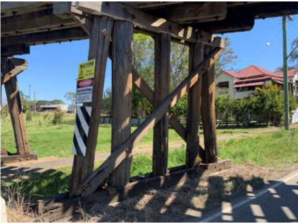
Pier 4 general view piles
