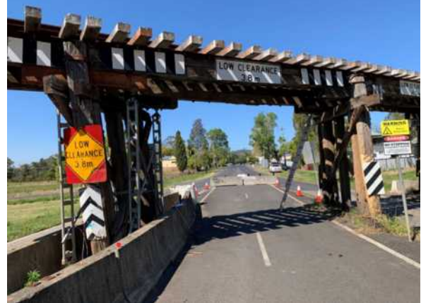
Span 6 west view
