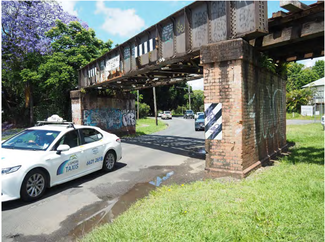
Figure B-19 Union Street – Metal span west elevation, typical condition (Source: FBE)
