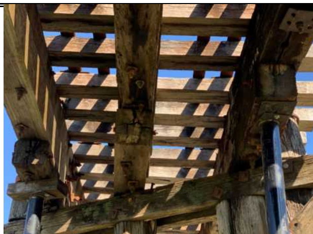
Pier 7 north end of corbels
