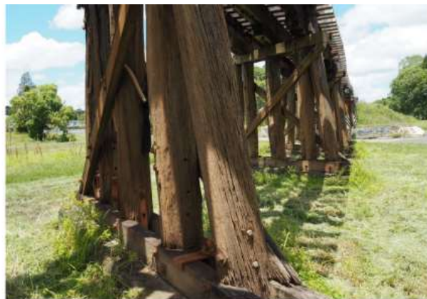
Figure B-15 Terania Street – Splitting & weathering of piles at Pier 11 (Source: FBE)
