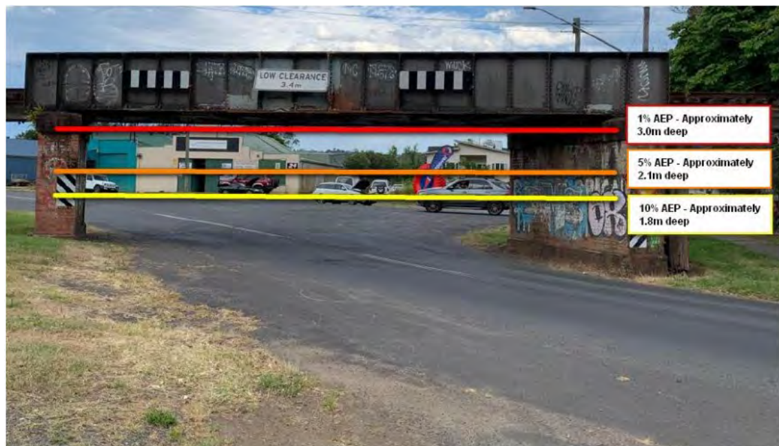
Figure 9-1 Union Street underbridge flood levels (Source: LCC)
