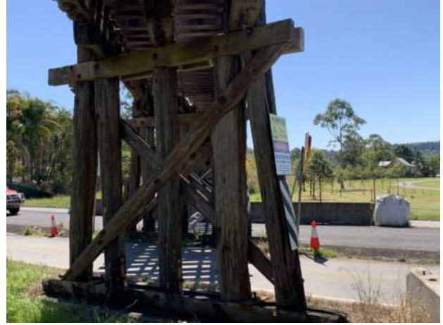
Pier 4 south view
