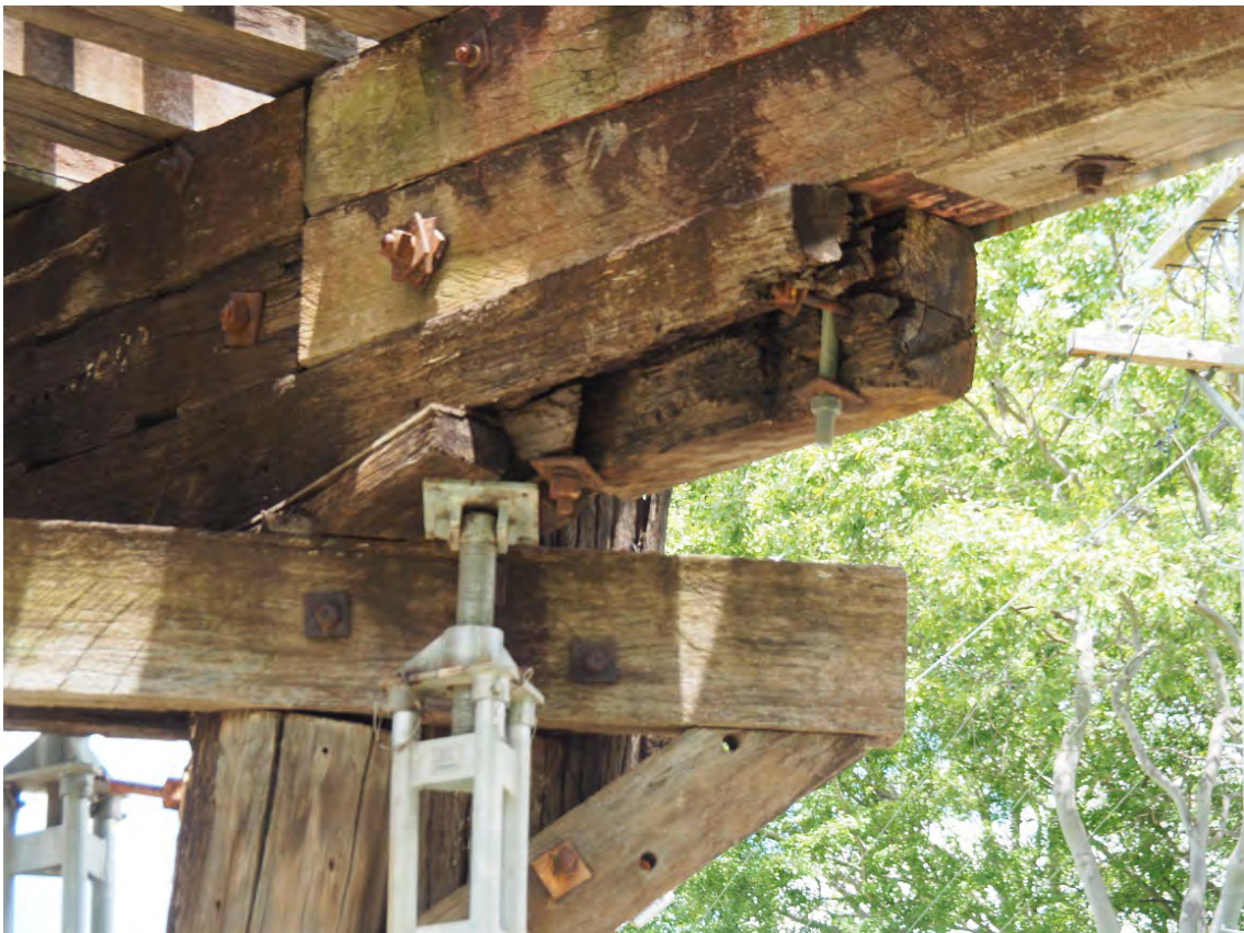
Figure B-14 Terania Street – Rotten and damaged east corbel at Pier 6 (Source: FBE)
