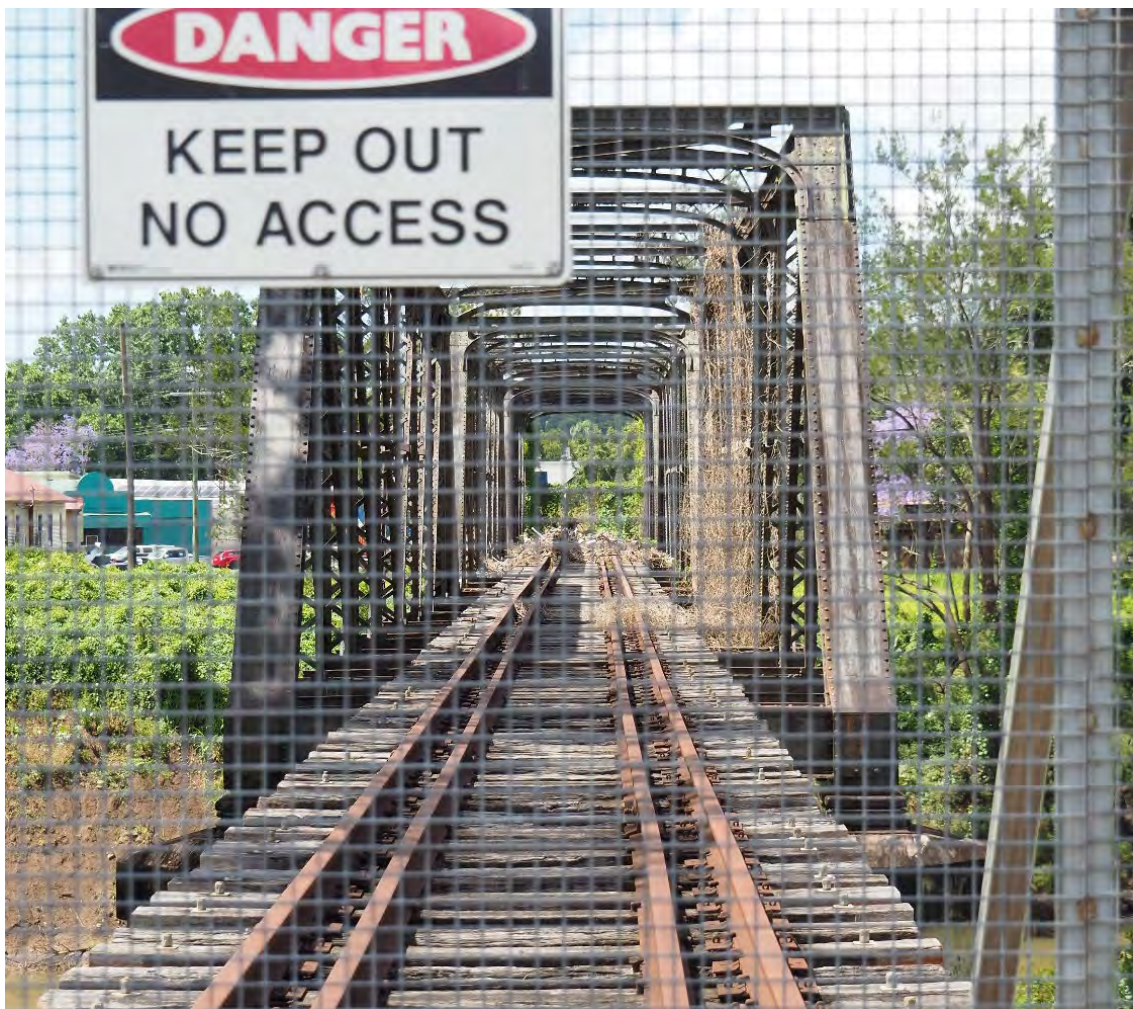
Figure B-11 Crane Street – View over looking south (Source: FBE)
