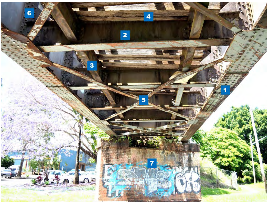
Figure A-2 Union Street metal span elements (Source: FBE)
