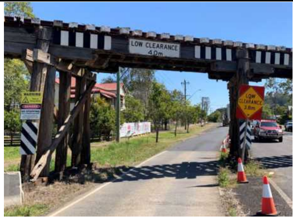
Span 5 east view
