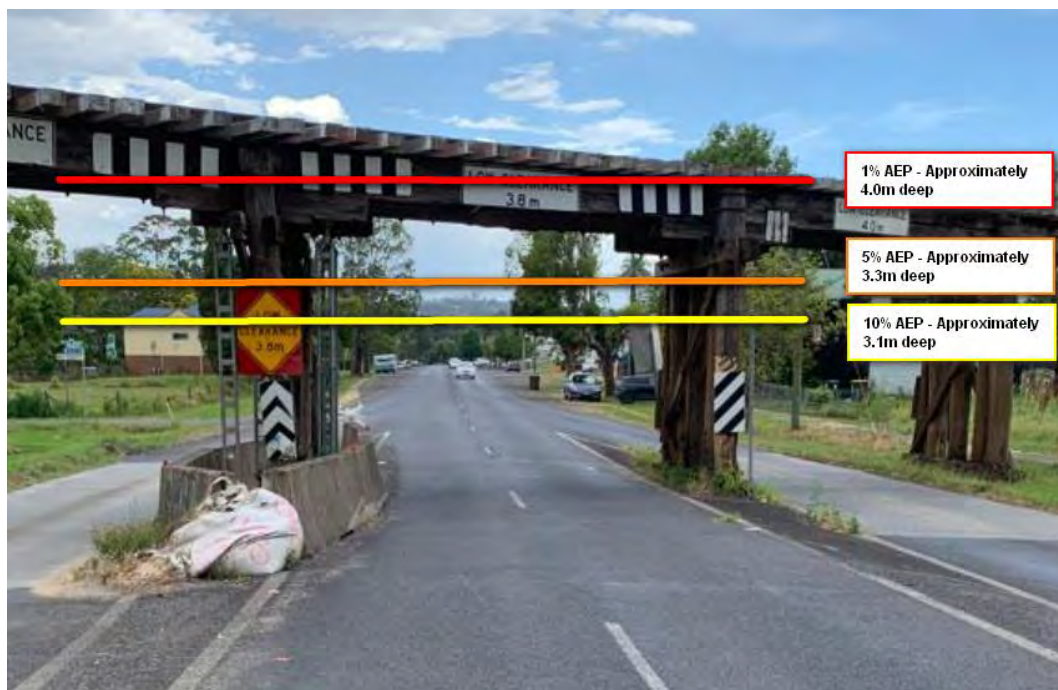
Figure 2: Terania Street Bridge with Flood Depths
