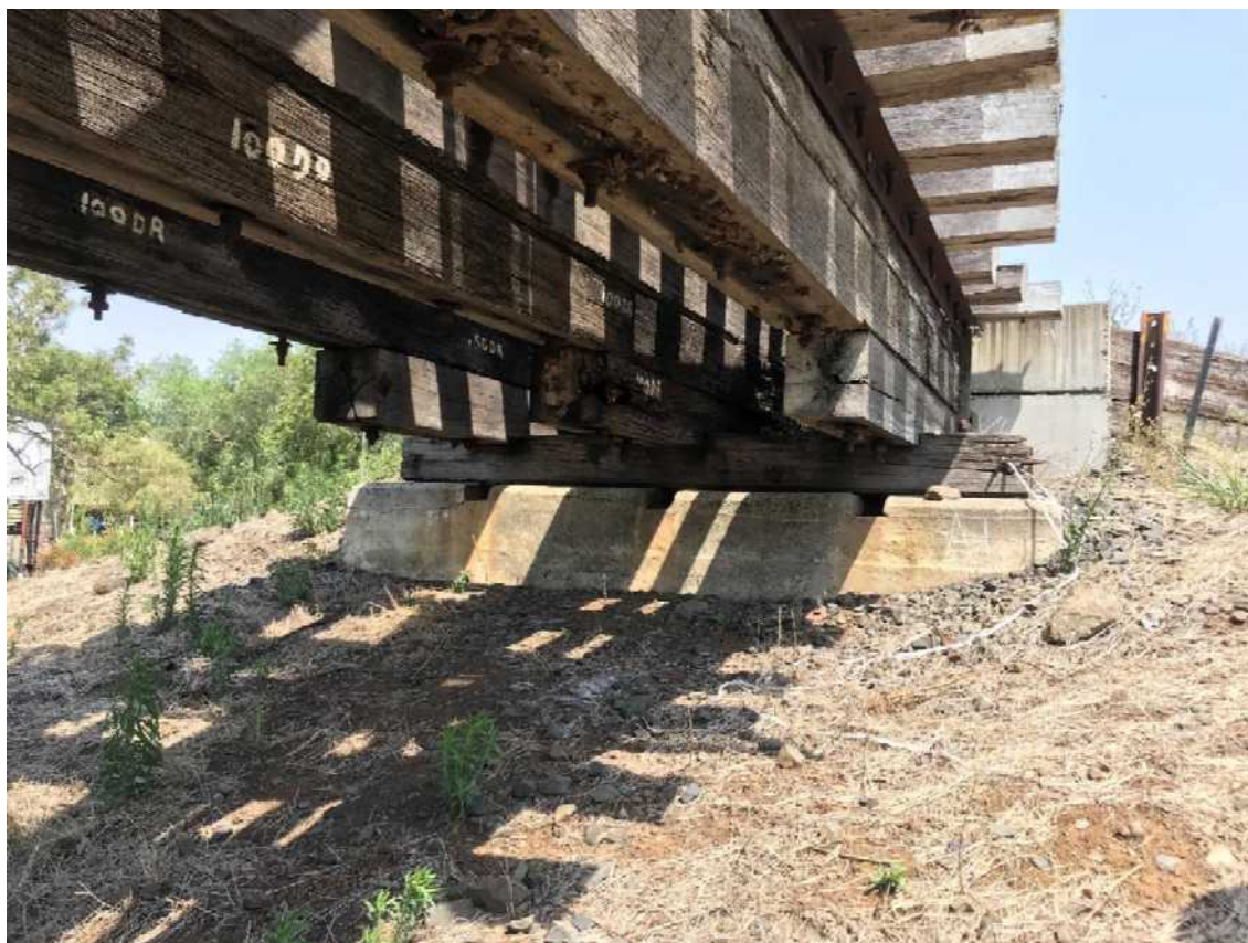
Figure 3-4 General view of Abutment 1 (south)
