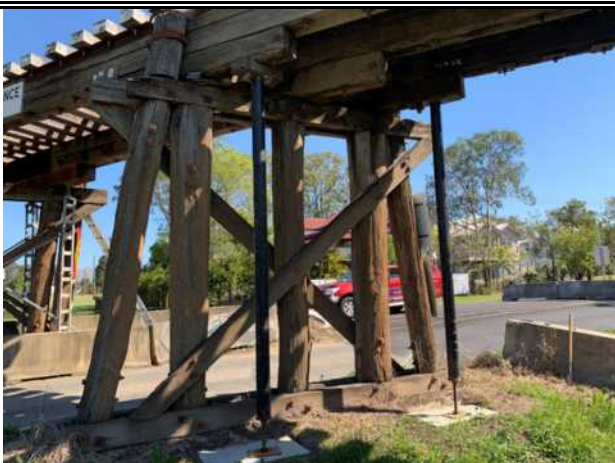
Pier 7 temporary propping under north end of outside corbels
