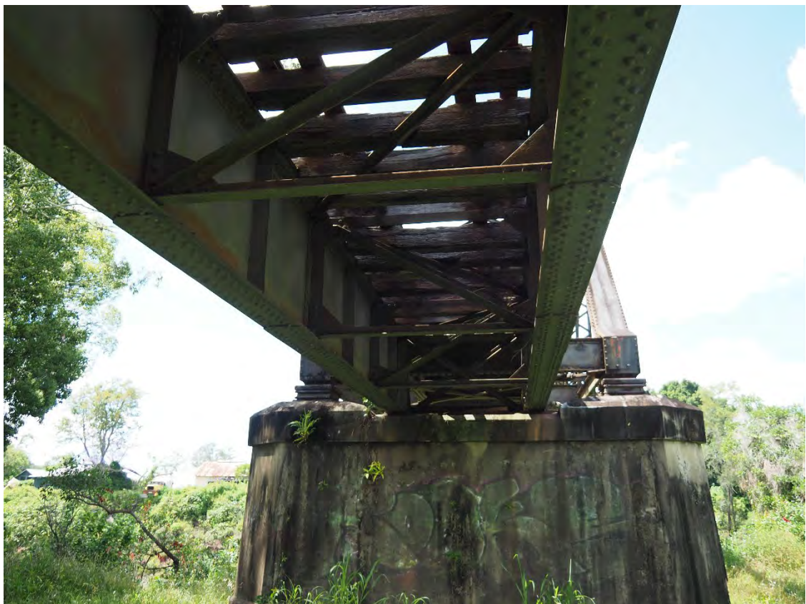
Figure B-8 Crane Street – Superstructure view from underside, Span 2 (Source: FBE)
