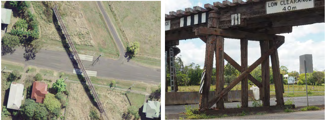
Figure 2-4 Terania Street Underbridge aerial view and trestle support (Source: SIX Maps / FBE)
