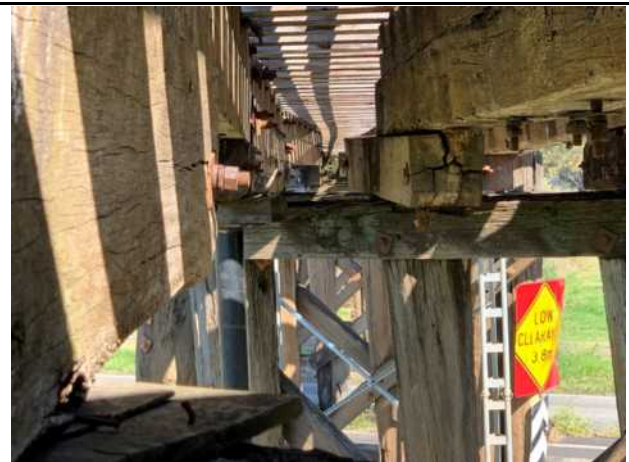
Piers 6 & 7 moved 300mm to east from vehicle impact
