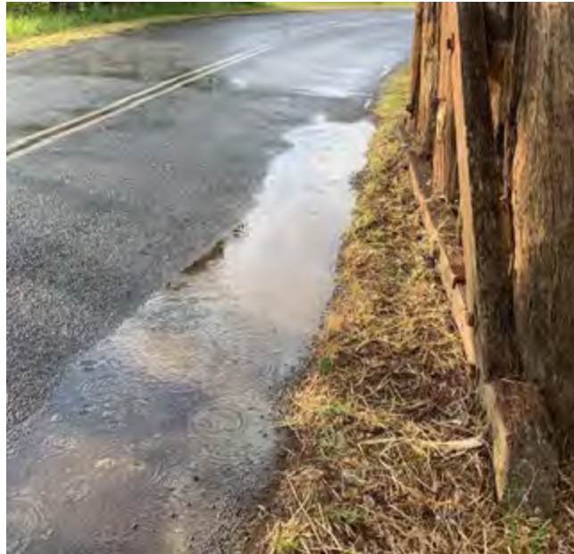
Photo 22: Roadside drainage at Winterton Parade viaduct
