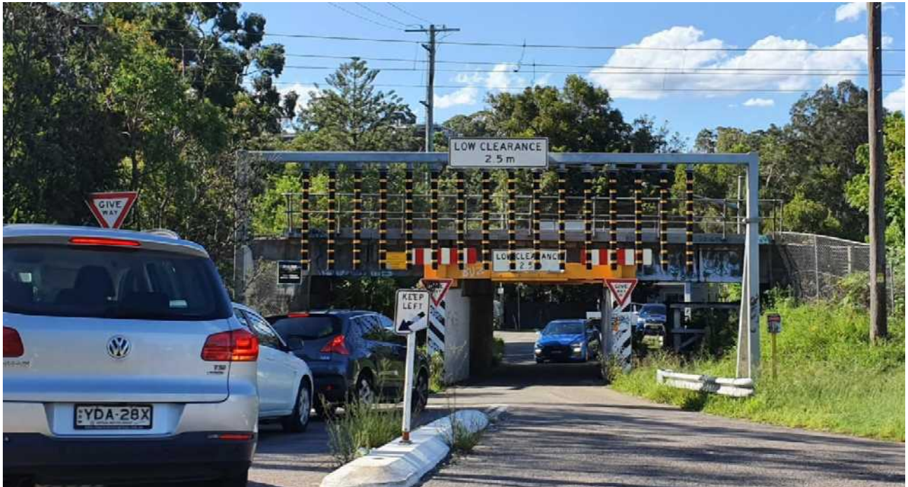
Example of Overhead Early Warning System (Woy Woy, NSW)
