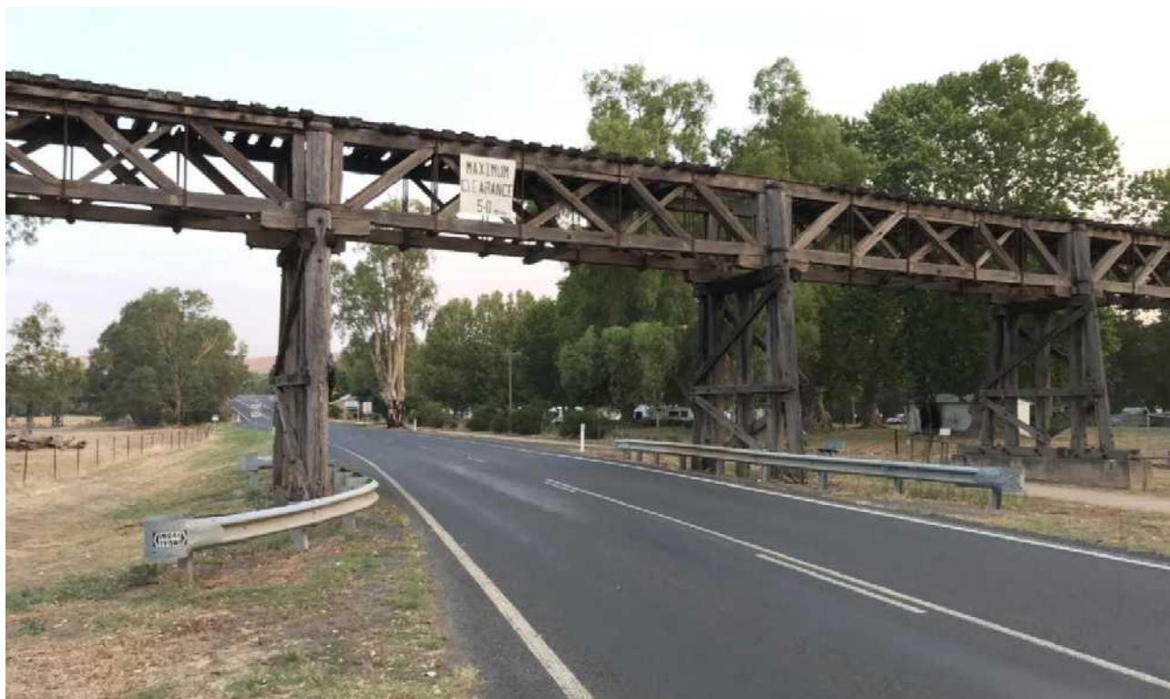
Example of Guard Rail protecting timber trestles (Gundagai, NSW)
