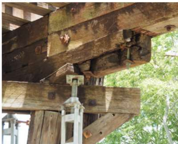
Figure B-14 Terania Street – Rotten and damaged east corbel at Pier 6 (Source: FBE)
