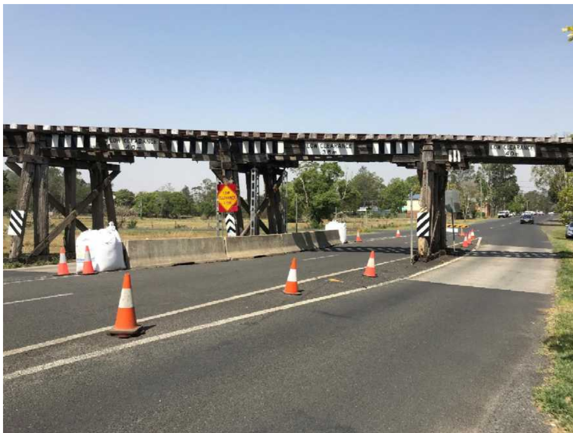
Figure 3-2 Downside elevation of bridge over Terania Street (looking east)
