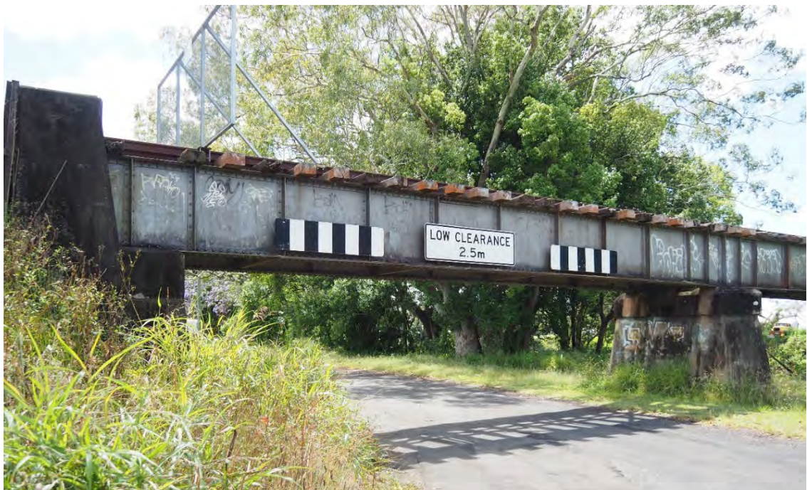
Figure B-7 Crane Street – East elevation, typical condition (Source: FBE)
