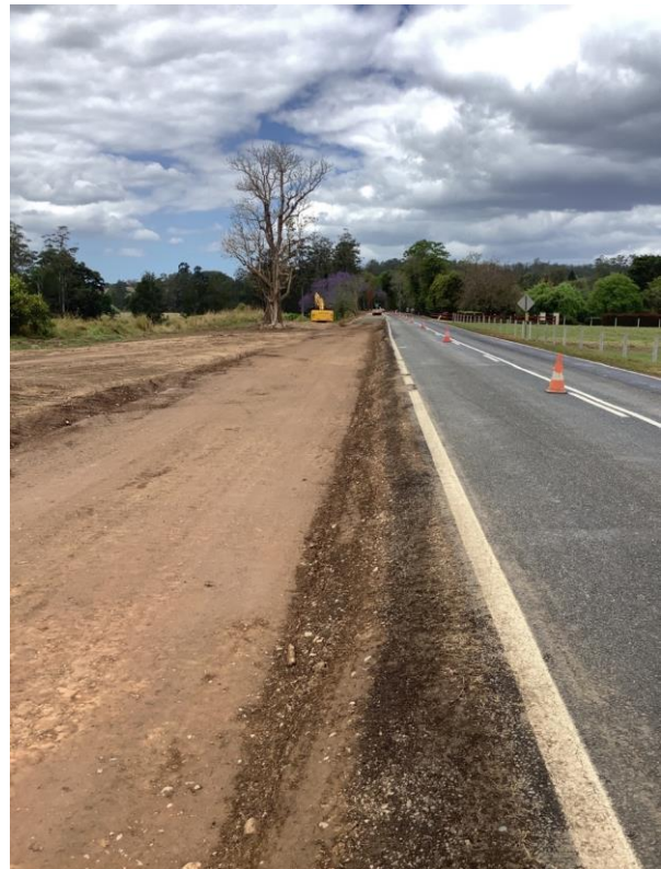
Wills Creek in progress 2023
