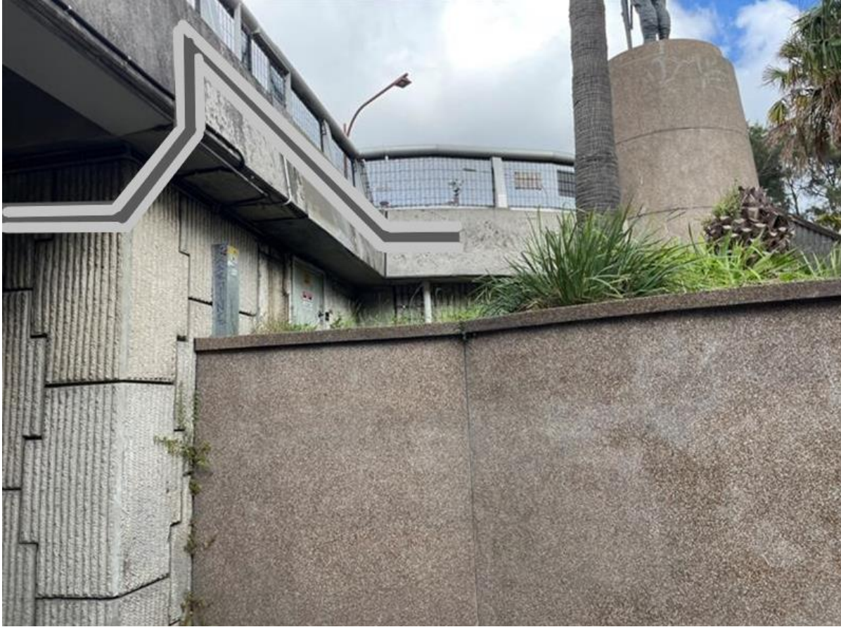
Figure 16 - Final Concept Design for Cable Tray Installation Under the Pier of the Western side of the Anzac Bridge, Rozelle
