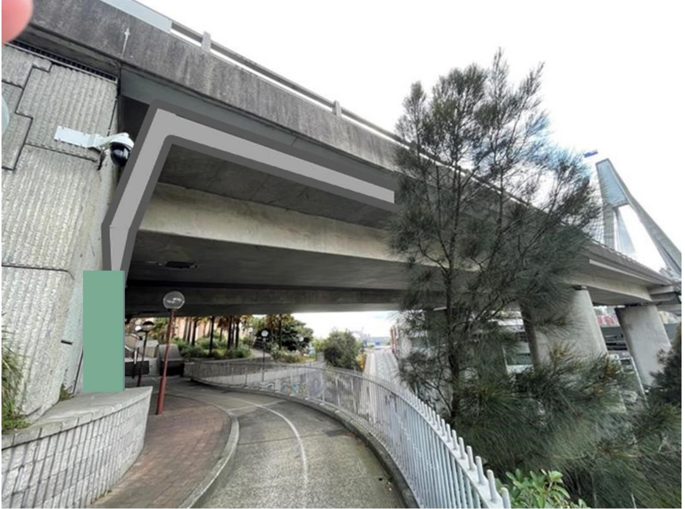
Figure 17 - Final Concept Design for Cable Tray Installation and RSC#30, Under the Pier of the Western side of the Anzac Bridge, Rozelle
