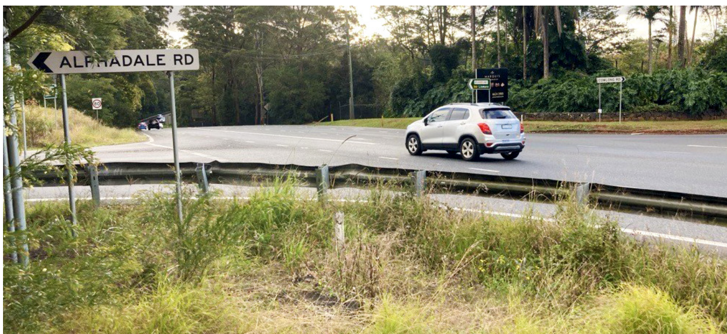
The intersection of Bruxner Highway and Cowlong and Alphadale roads
