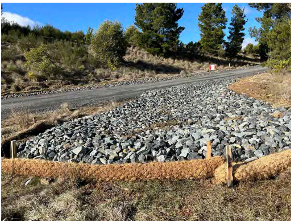
Photo 10: New rock armoury and sediment coir logs adjacent to the north of the site was observed during the inspection.
