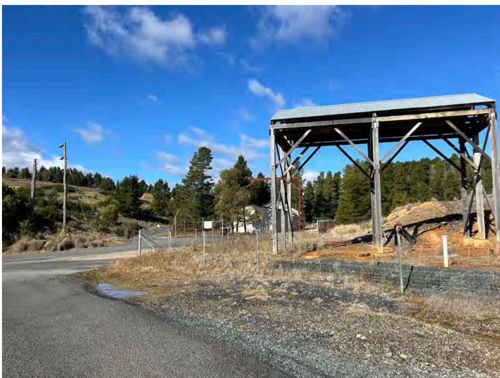
Photo 8: Sealed road over Copper Creek Road crossing, preventing inadvertent access to site materials underneath. Pooled water was observed.
