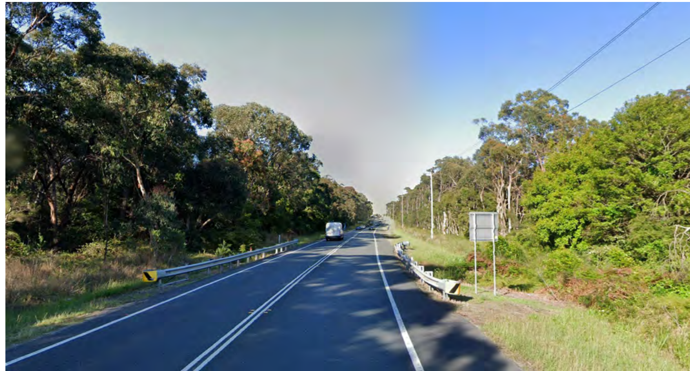
5 Hillsborough Road looking south west at unnamed creek crossing
