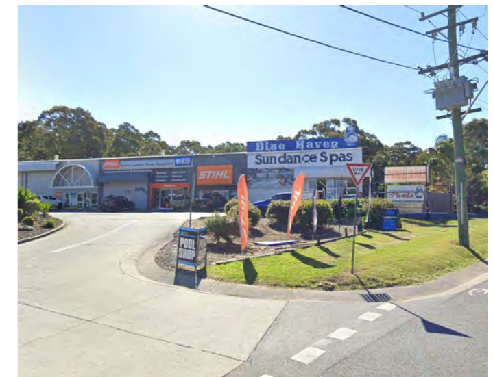
Hillsborough Road looking north at intersection with access road
