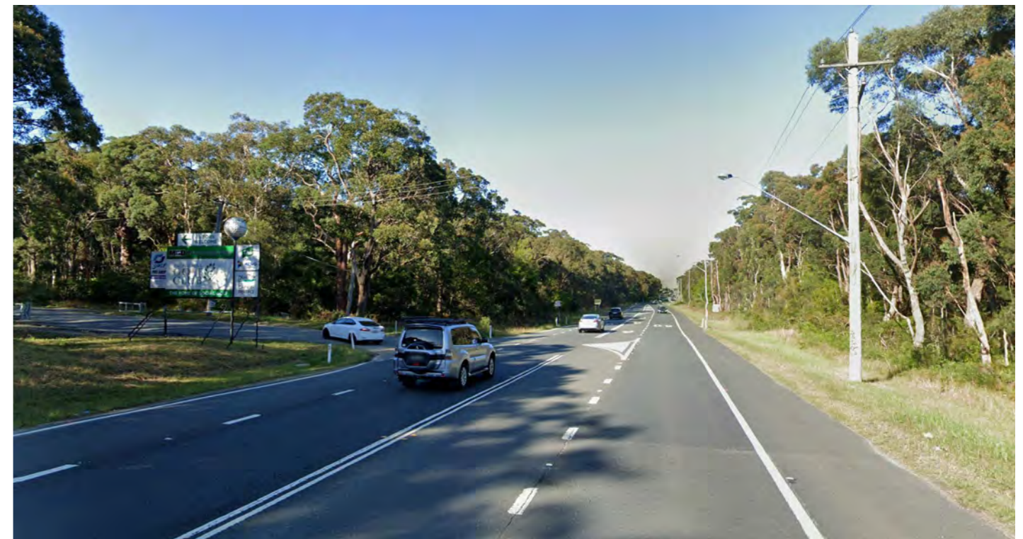
4 Hillsborough Road looking south west towards intersection with Barker Avenue
