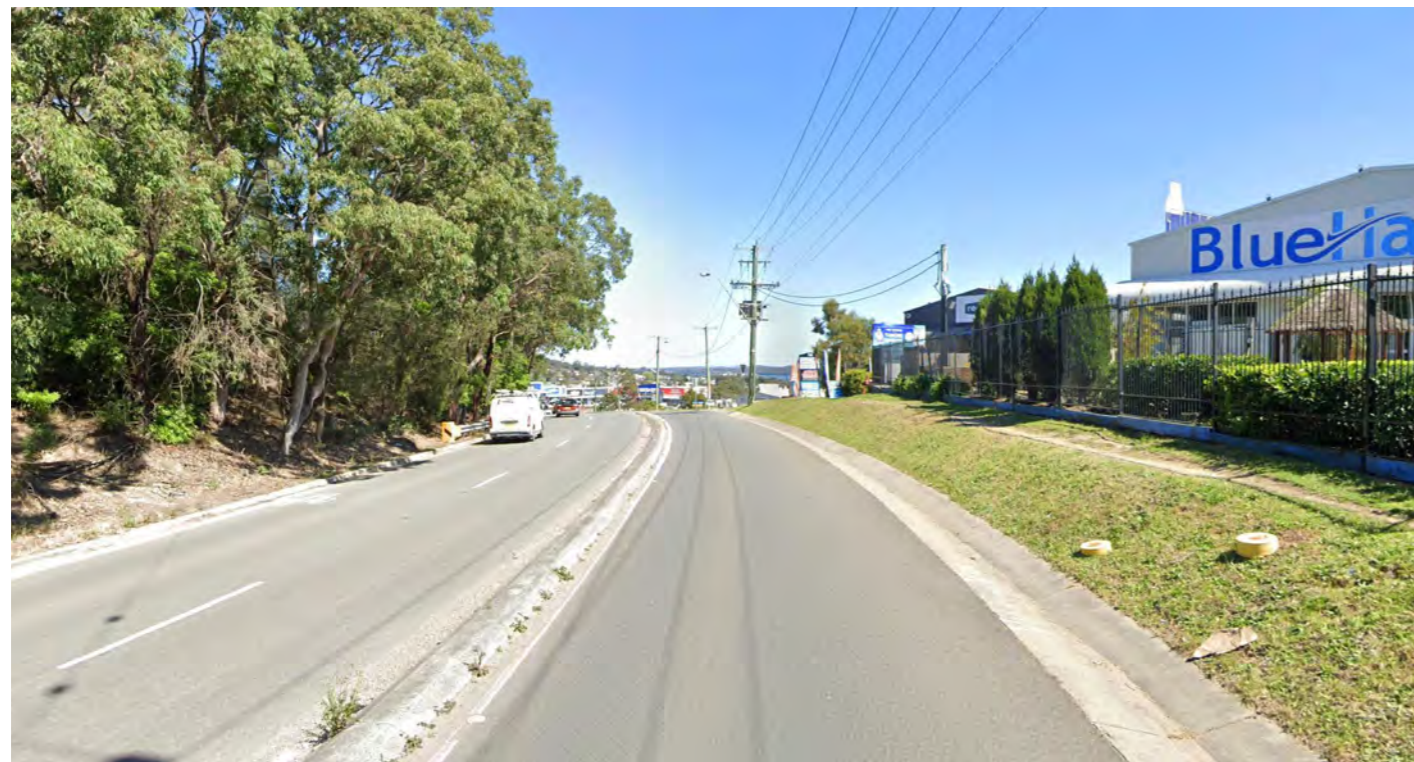
7 Hillsborough Road looking south west towards Warners Bay light industrial and bulky goods retail area
