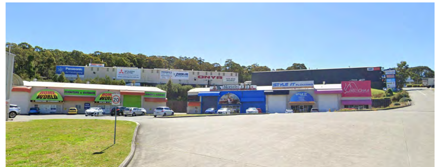
Access road looking north west towards industrial area
