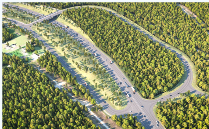
The design of the S-type intersection at Princes Highway and Hawken Road
