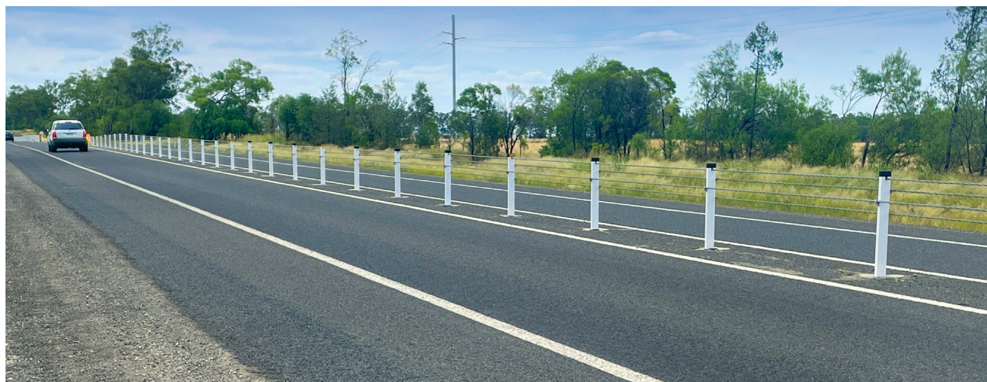
Flexible safety barriers in Section 4, February 2024
