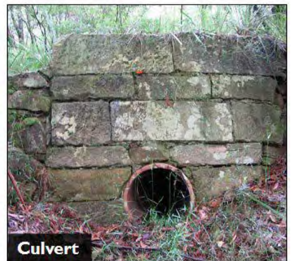
Figures: Top left-hand picture continuing clockwise: road pavement (Great Western Highway, Lawson); sandstone kerbing (Parramatta Road, Mays Hill); Telford sandstone road base (Great Western Highway, Leura); ceramic conduit and sandstone culvert headwall (Blue Mountains, NSW); corduroy timber road base (Entrance Road, Wamberal).
