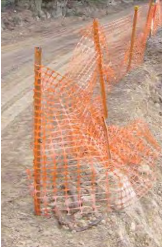
Figure B-4: Example of star pickets and boundary fencing around a restricted zone.
