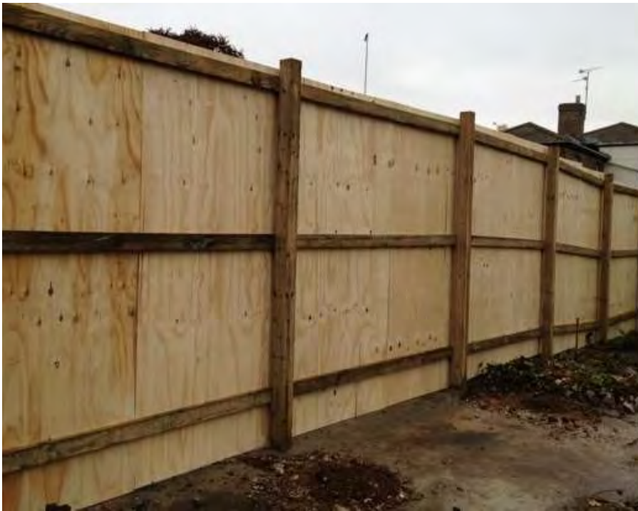
Figure B-1: Example of typical marine ply hoarding.
