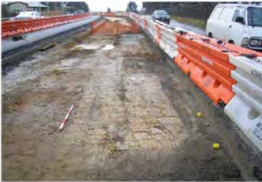
Figure 1: Telford road uncovered on the Great Western Highway (Leura) in 2008.
