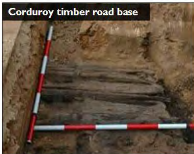
Figures: Top left-hand picture continuing clockwise: road pavement (Great Western Highway, Lawson); sandstone kerbing (Parramatta Road, Mays Hill); Telford sandstone road base (Great Western Highway, Leura); ceramic conduit and sandstone culvert headwall (Blue Mountains, NSW); corduroy timber road base (Entrance Road, Wamberal).
