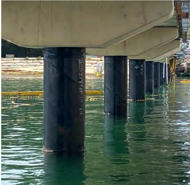
▲ Installed steel piles with protective marine-grade coating
