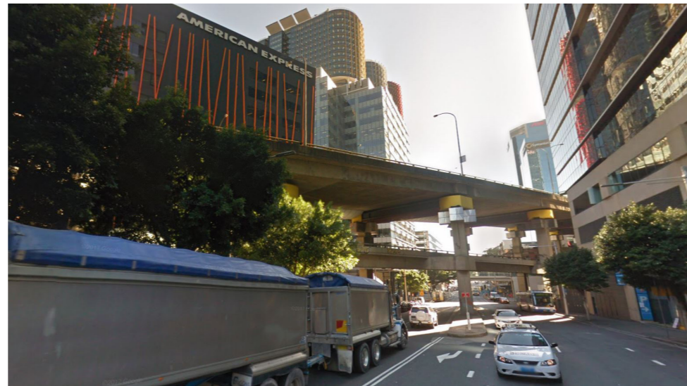
Figure 75: Existing View of Gantry Location 17 from Sussex Street
