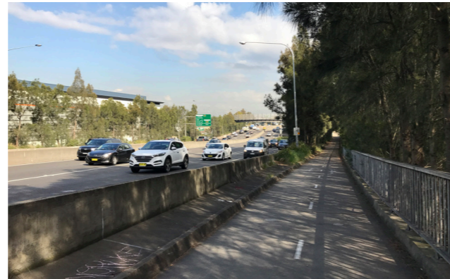
Shared path on northern side of City West Link Road.
