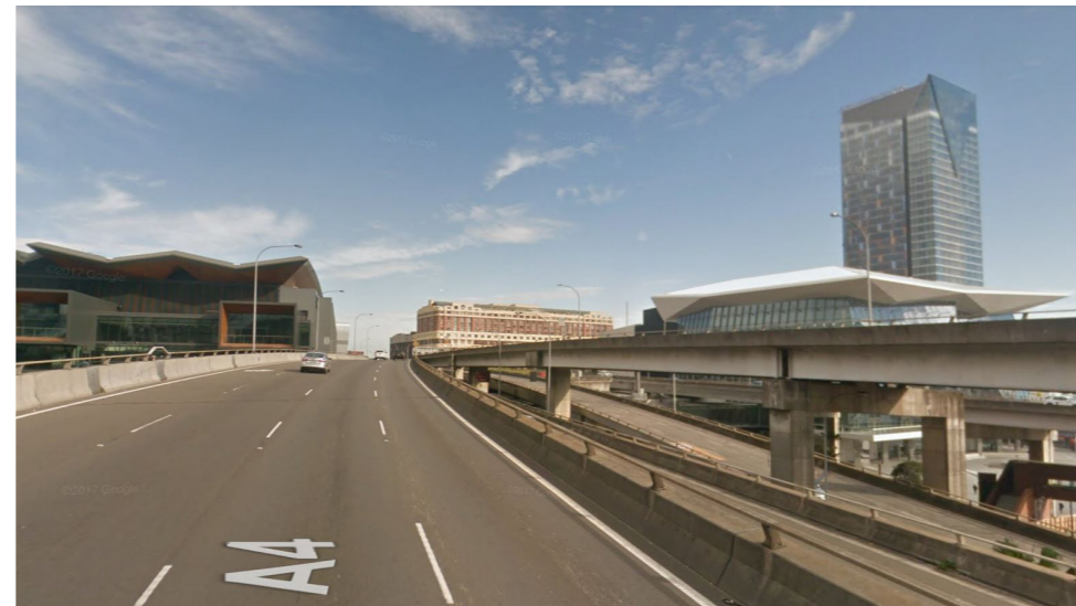
Figure 57: Existing View of Gantry Location 9
