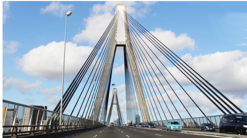
Figure 35: Existing View of Gantry Location 1
