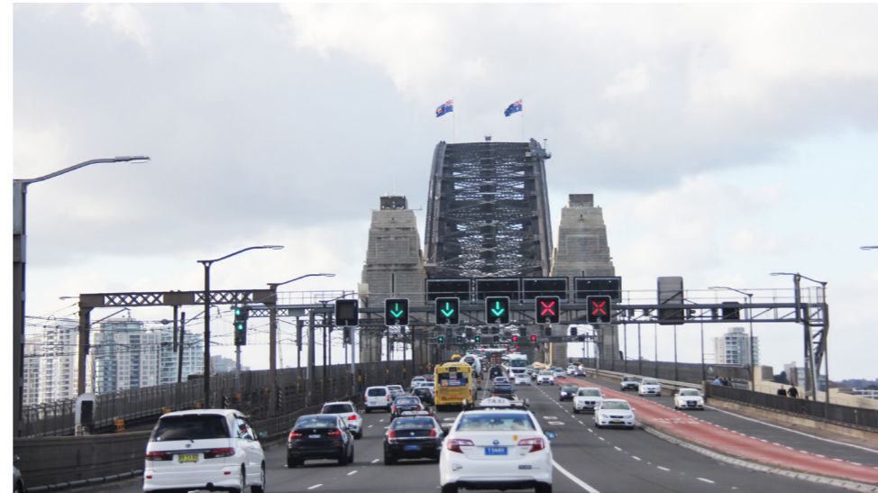
Figure 81: Existing View of Gantry Location 24
