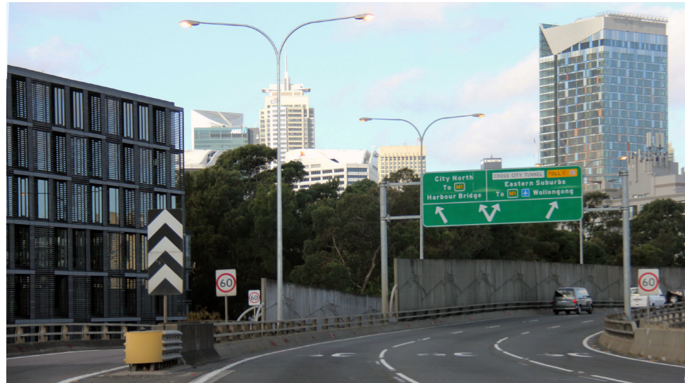
Figure 41: Existing View of Gantry Location 3
