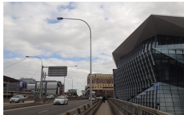
Shared path on northern side of Western Distributor at Darling Harbour, looking west.
