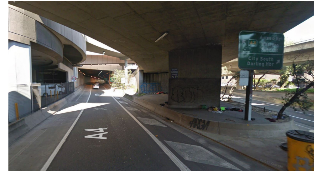
Figure 65: Existing View of Gantry Location 13
