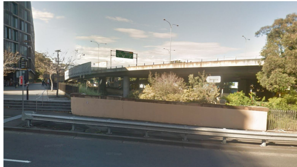
Figure 43: Existing View of Gantry Location 3
