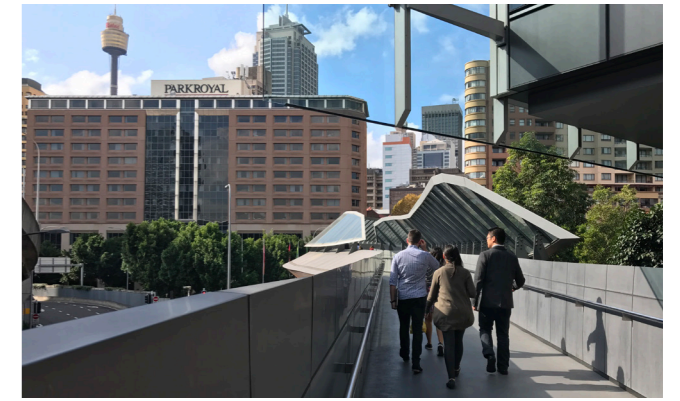
Pedestrian bridge across Harbour Street at Darling Harbour.
