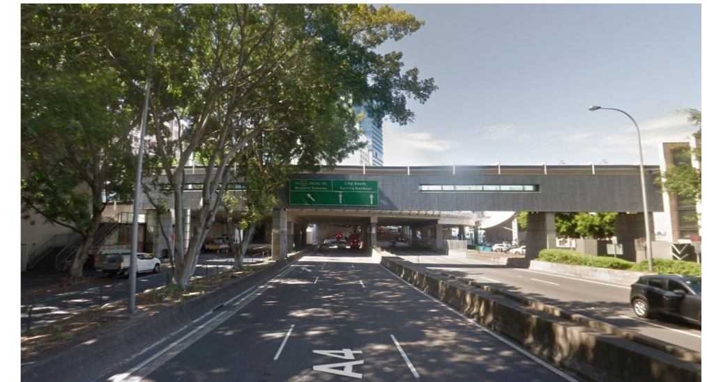
Figure 71: Existing View of Gantry Location 16
