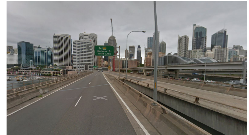
Figure 59: Existing View of Gantry Location 10
