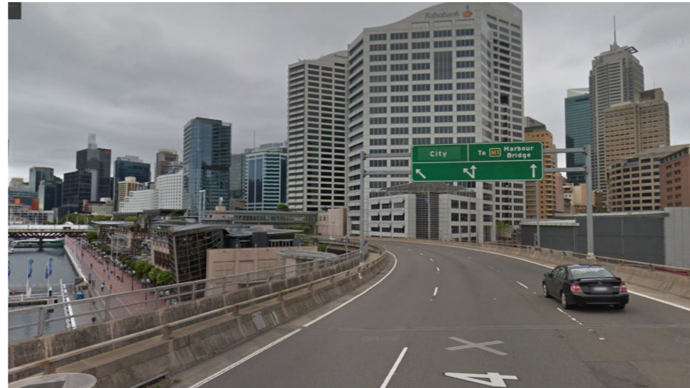
Figure 63: Existing View of Gantry Location 12
