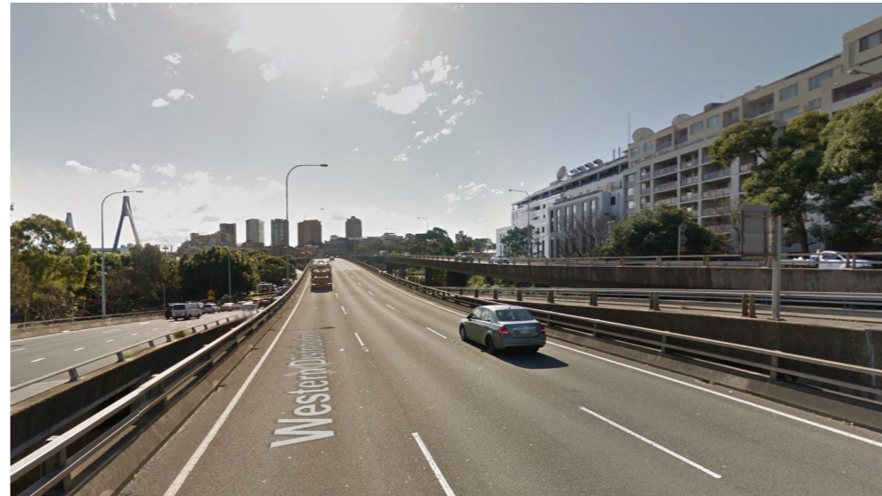
Figure 51: Existing View of Gantry Location 6
