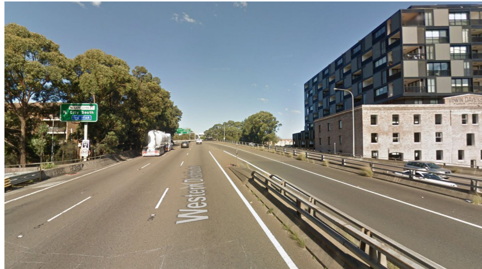
Figure 49: Existing View of Gantry Location 5
