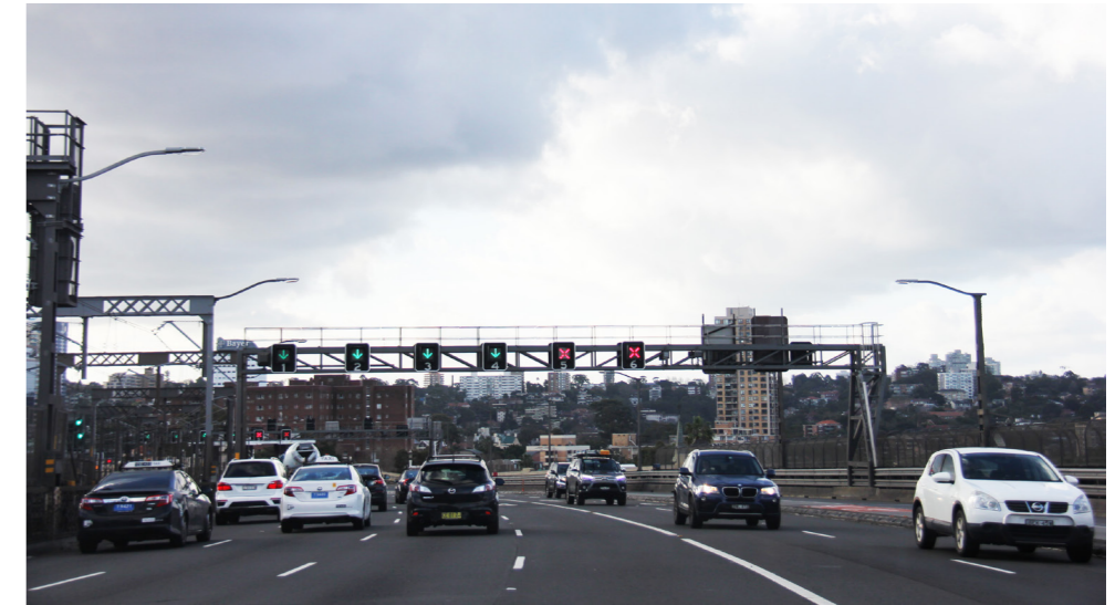
Figure 83: Existing View of Gantry Location 25
