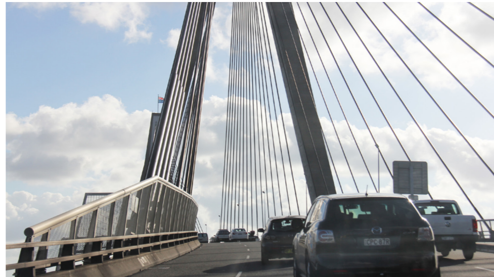
Figure 37: Existing View of Gantry Location 2
