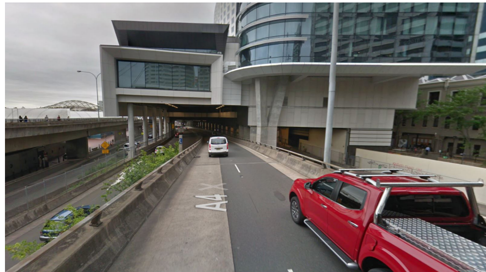
Figure 67: Existing View of Gantry Location 14
