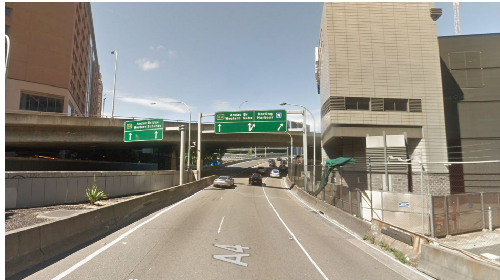
Figure 61: Existing View of Gantry Location 11
