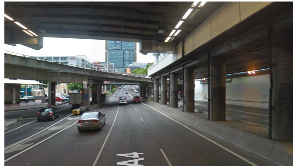
Figure 69: Existing View of Gantry Location 15
