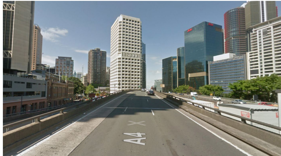
Figure 79: Existing View of Gantry Location 19
