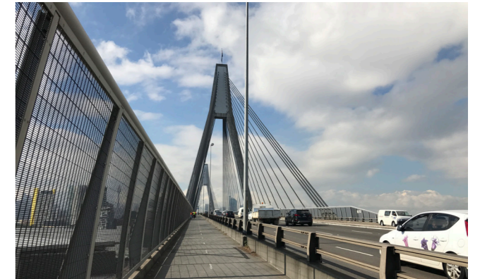
Eastern approach to Anzac Bridge.
