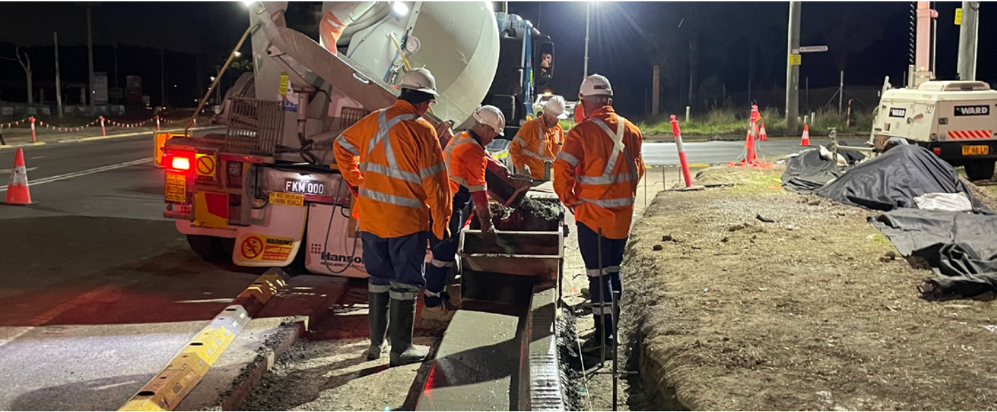
Extrusion of kerb on southwest corner of Devonshire Road and Elizabeth Drive Intersection
