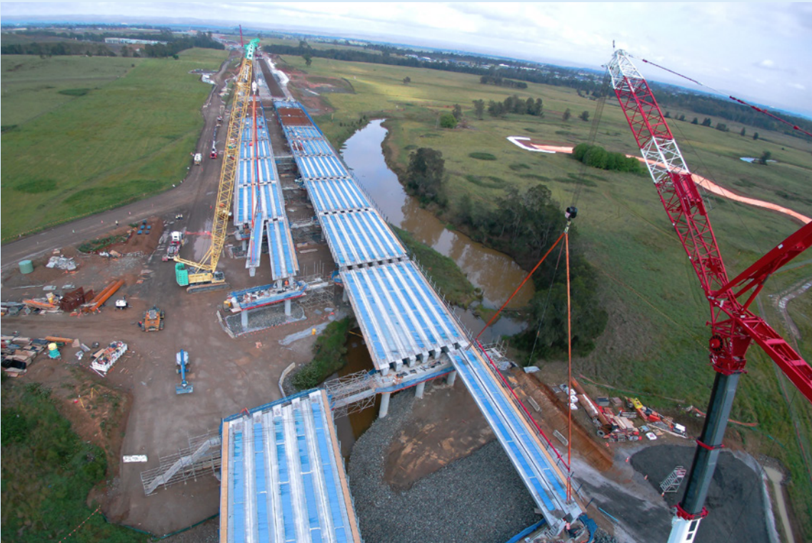
South Creek bridge girder installation
