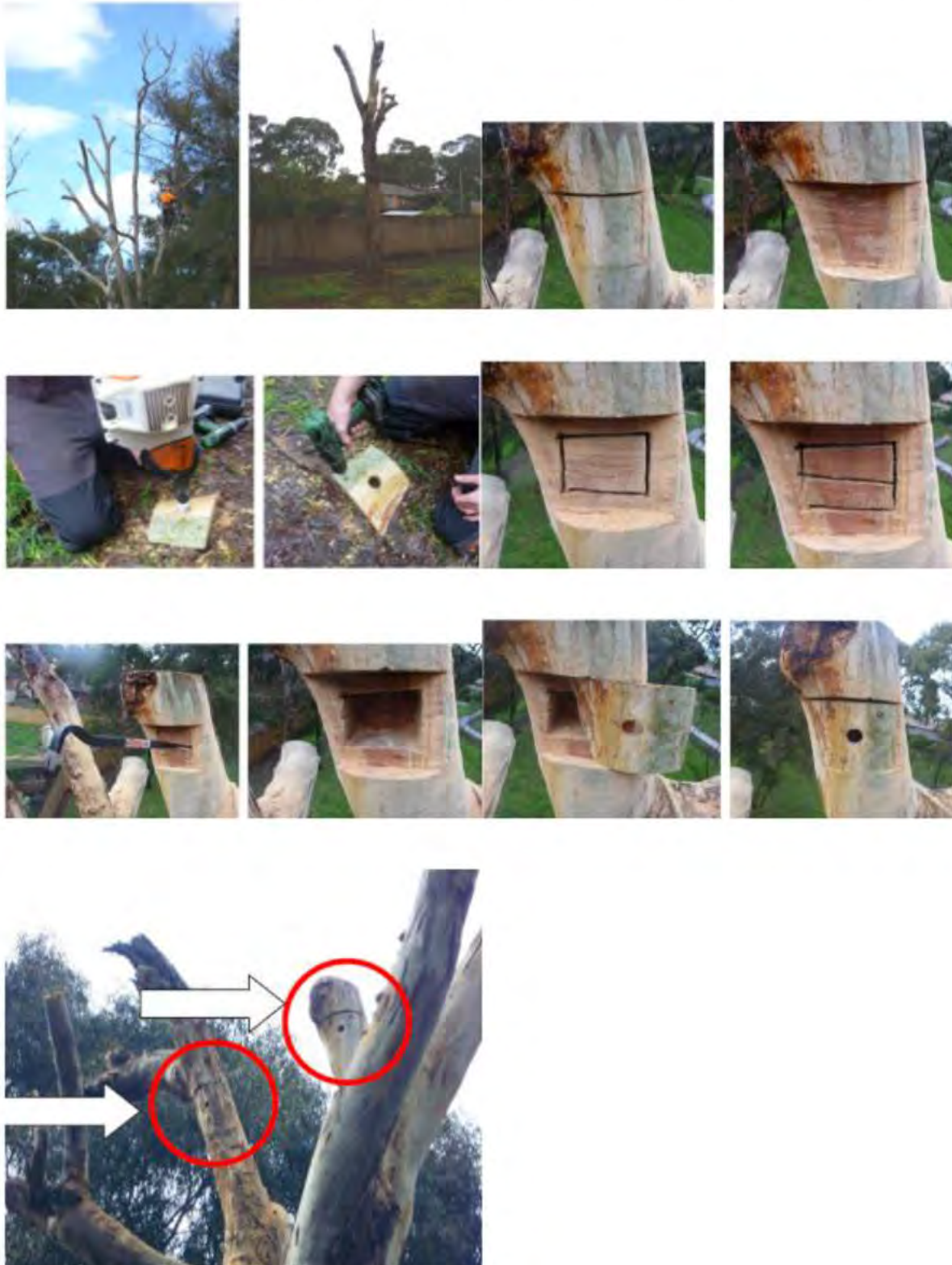
Figure 6-1 Procedure for the installation of trunk hollows (The University of Melbourne, 2013)
