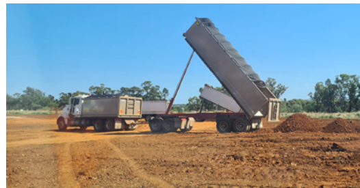
Trucks transporting and distributing the spoil for re-purpose
