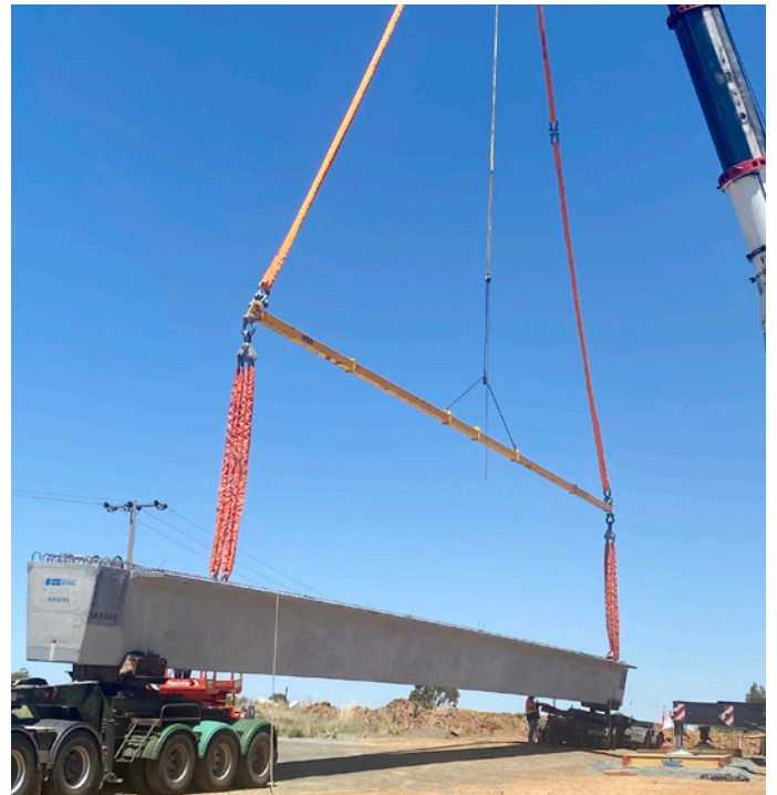
Girder being placed for the Victoria Street Bridge
