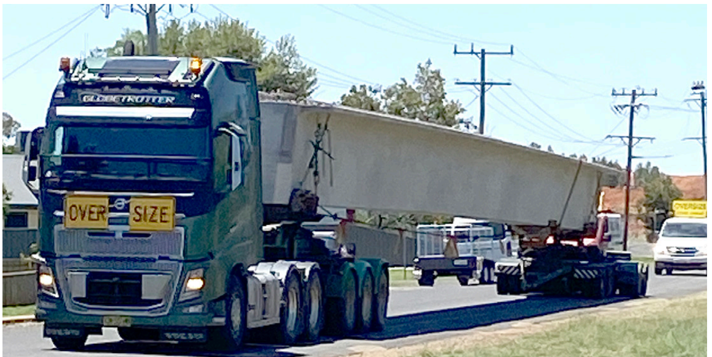
Girder being delivered for the Victoria Street Bridge
