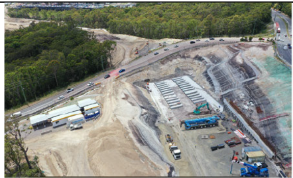
Bridge 1 and cut 1
