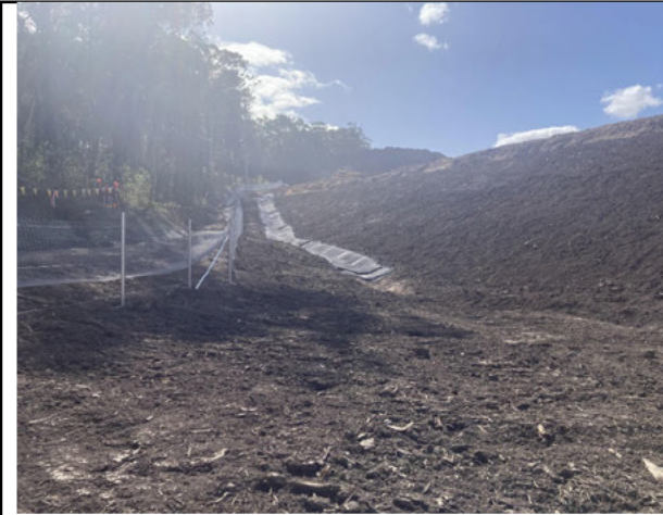
Fencing and permanent drainage
