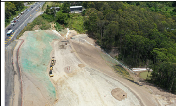
Fill 1 batter and progressive landscaping
