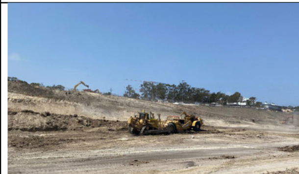
scraper and bulldozer
