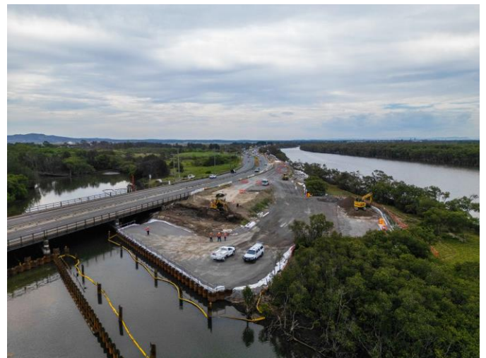
Bridge abutment work at Ironbark Creek
