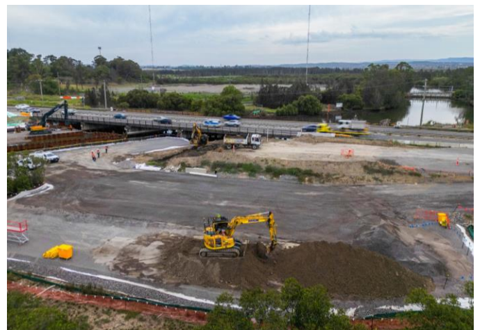
Crane platform for the Ironbark Creek bridge
