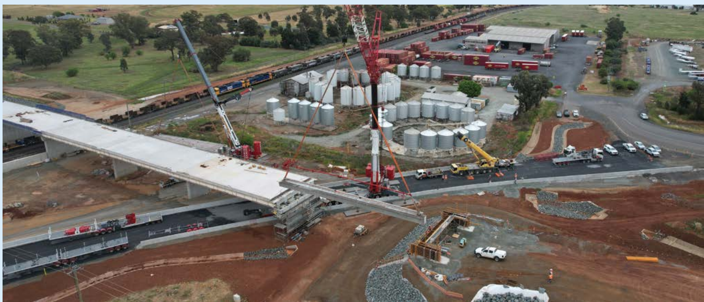
The final girders being lifted for the Bridge over Rail
